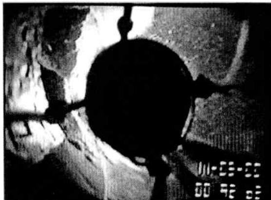
Fig. 9. Interior view of liner conforming to hole
