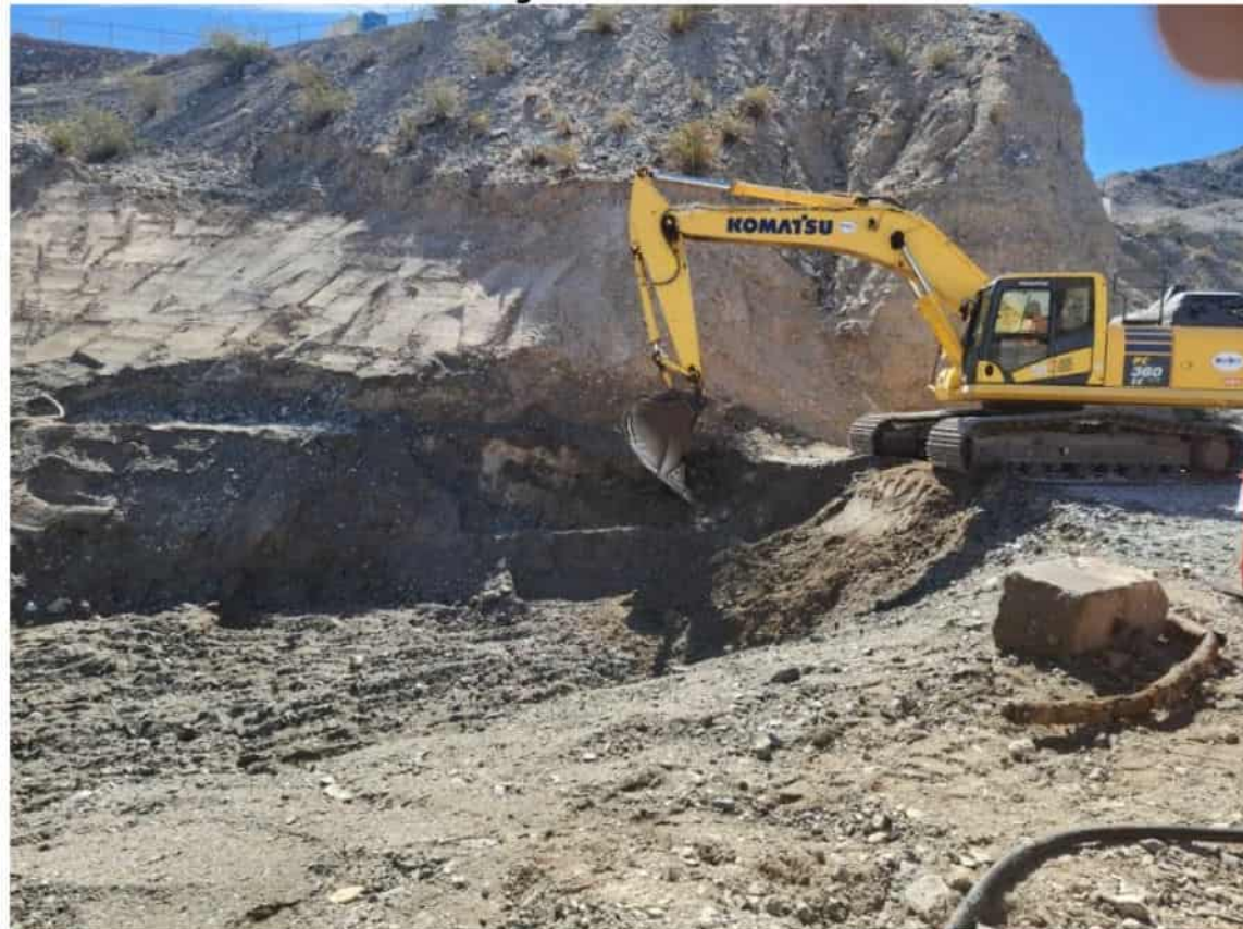
SWMU1 TAA1 Visible white powder lens and greenish gray discolored soil - Facing Southeast
