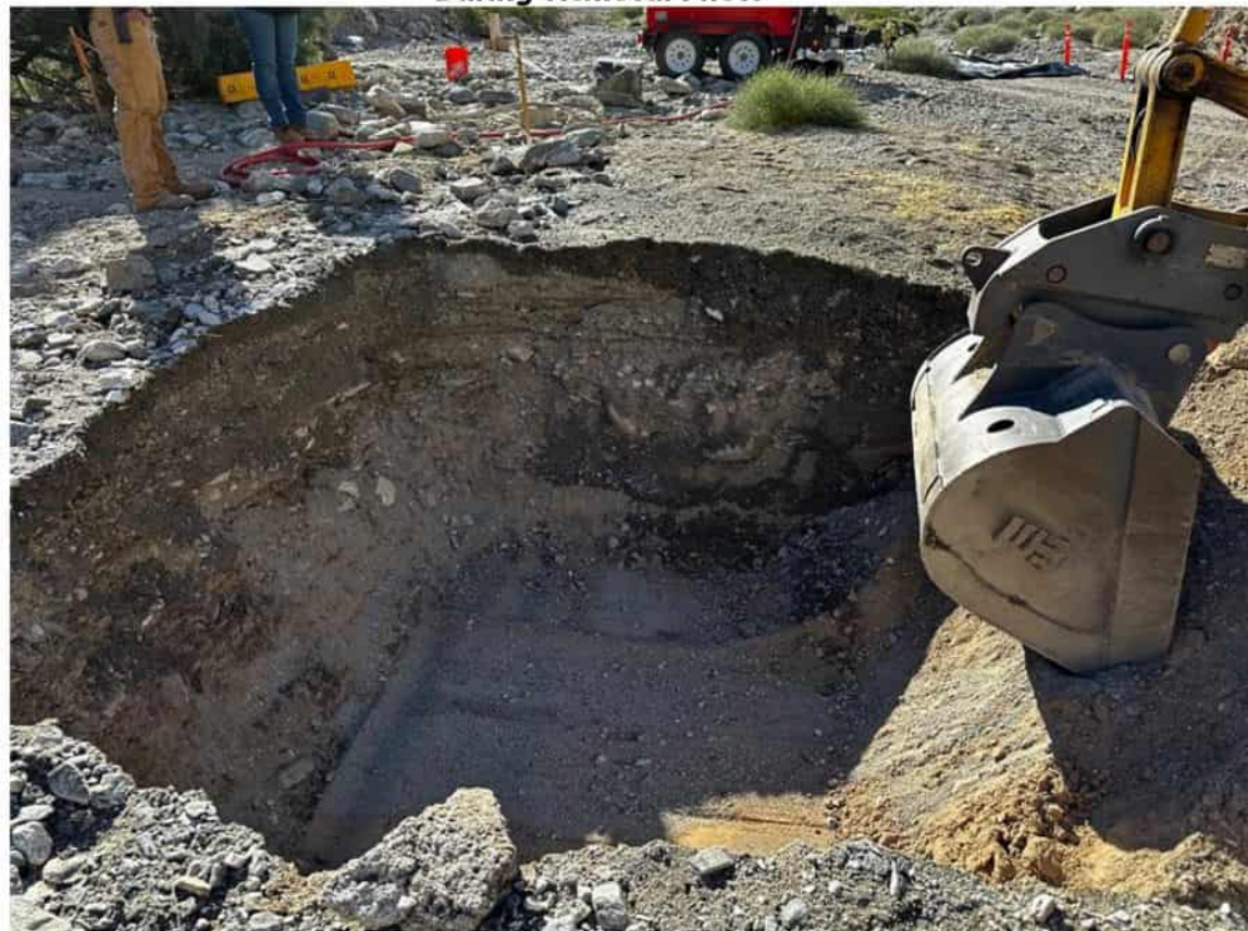
AOC1 TAA1 Initial excavation - Facing South
