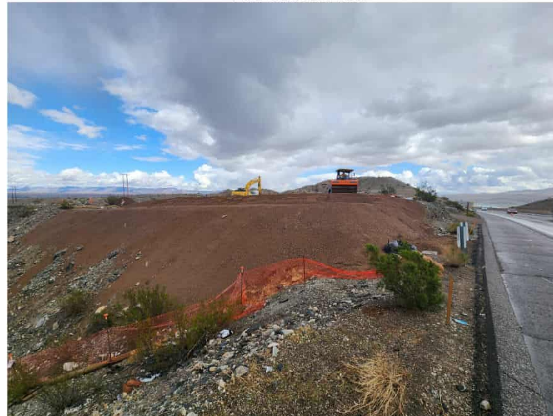
AOC14 TAA1 Facing East
