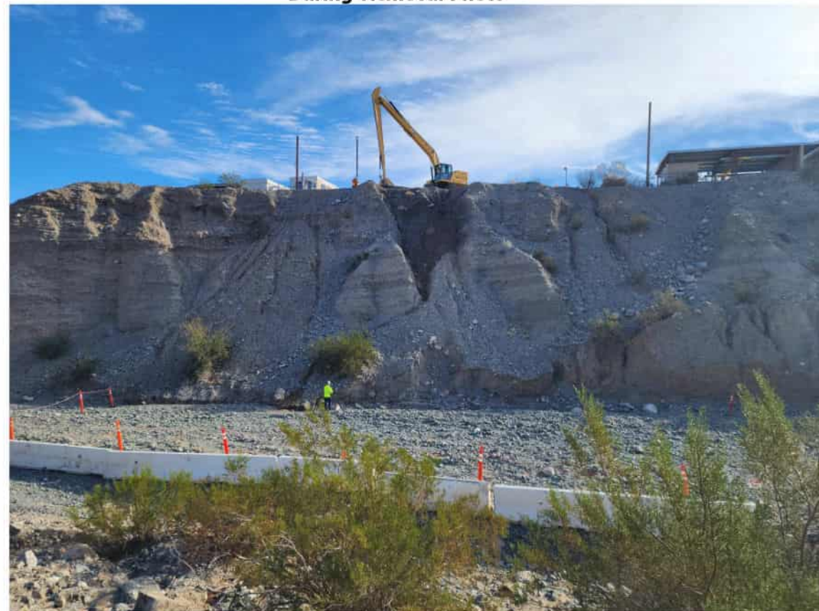
SWMU1 TAA3 Initial excavation from top of slope - Facing East
