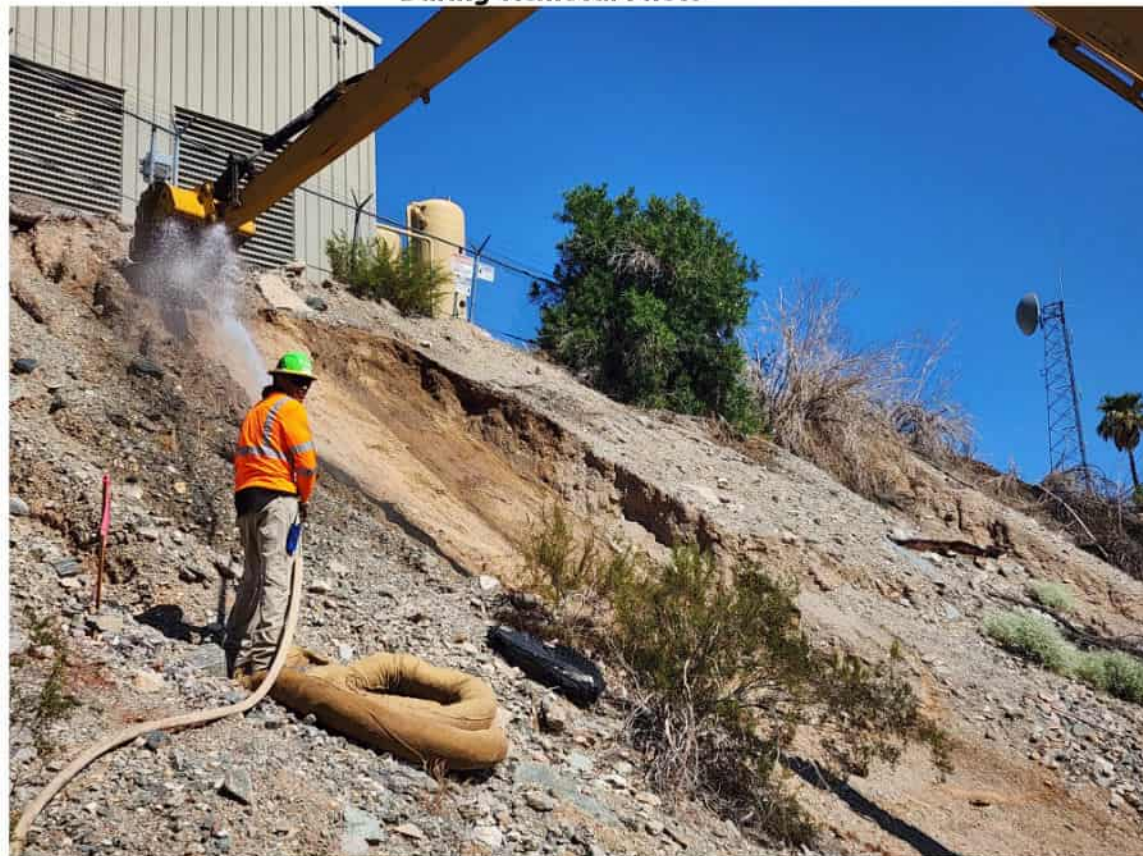
AOC9 TAA1 Initial excavation and debris removal - Facing North
