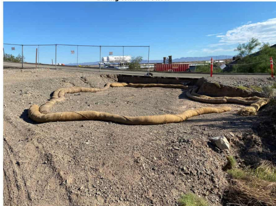
AOC10 TAA3 Initial excavation - Facing North
