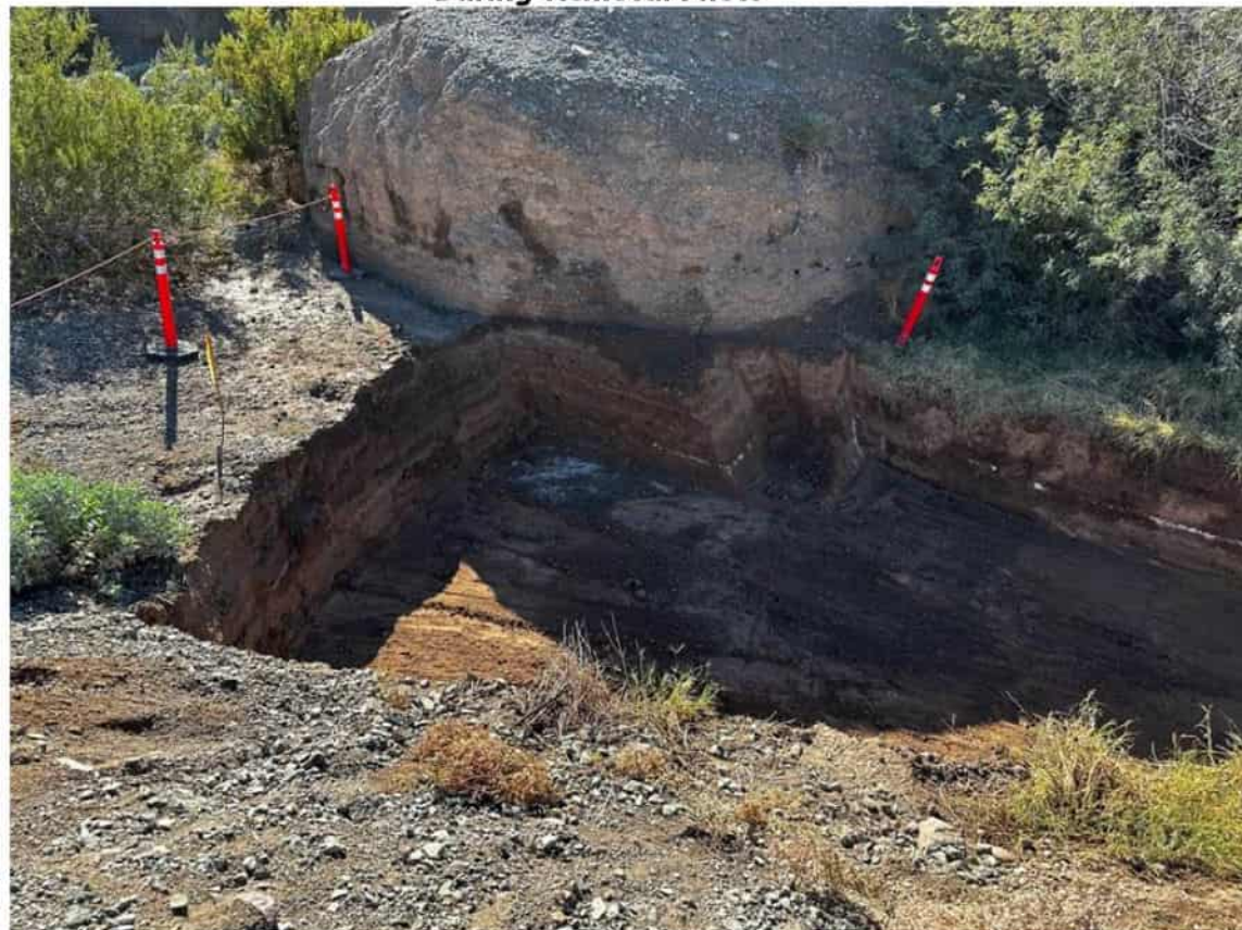
AOC10 TAA4 Initial excavation and visible white powder lens - Facing Southwest
