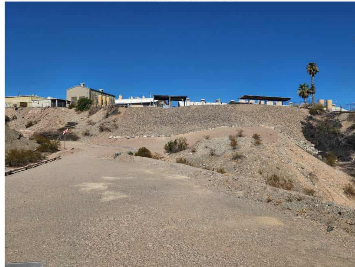
AOC10 TAA1 Facing West
