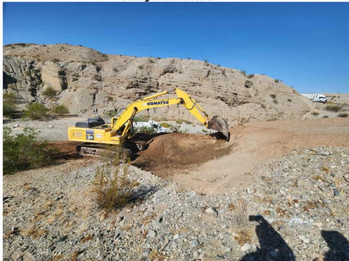
AOC27 TAA1 Initial excavation - Facing West
