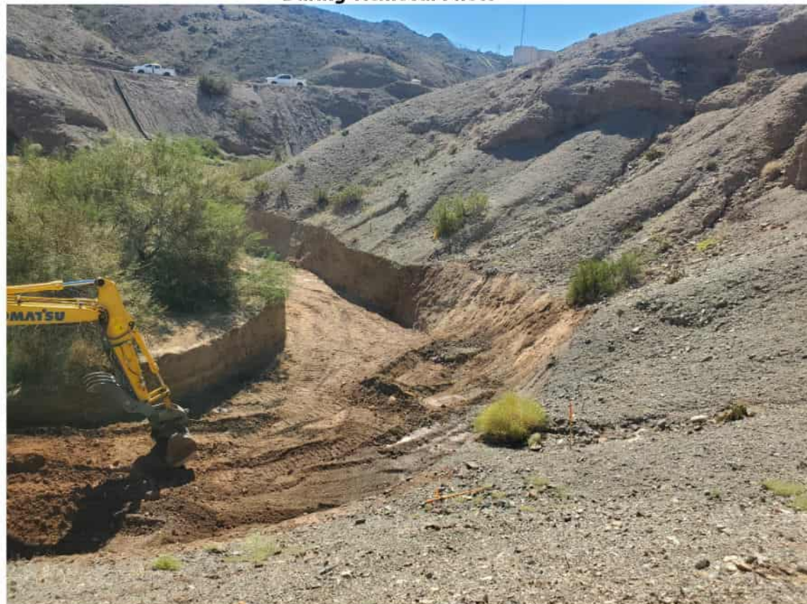
AOC10 TAA2 Initial excavation around mesquite trees - Facing South
