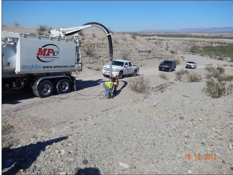
Photo 1. Potholing at SWG-HV- 4.
