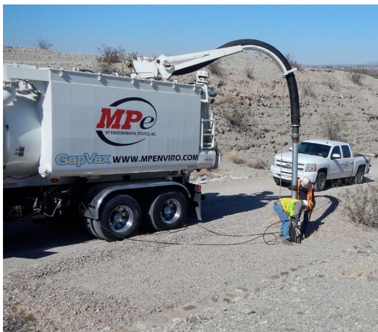
Potholing for the Topock Remediation project
