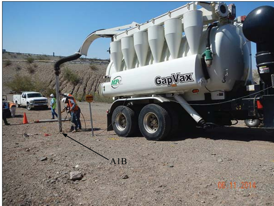
Photo 1. Potholing activity at location A1B.
