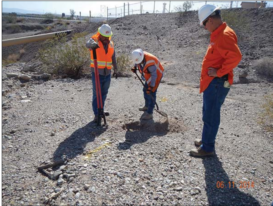
Photo 3. Manual excavation at Pothole Location A3B.
