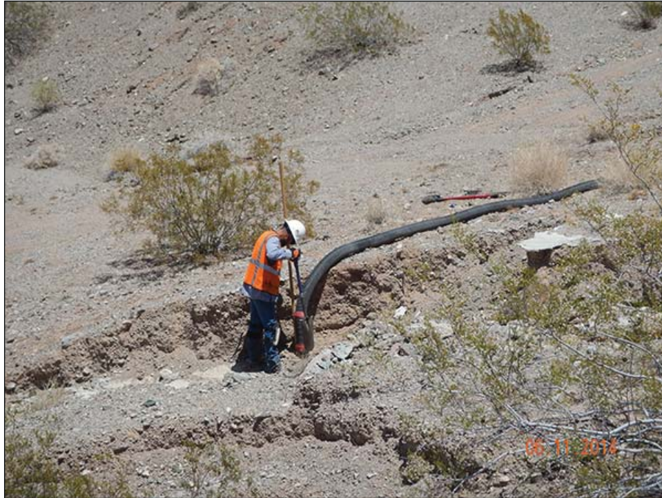
Photo 5. Potholing activity at Pothole Location A4A utilizing extension hose.
