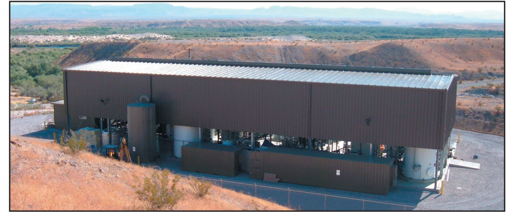
Treatment facility for Interim Measure No. 3
