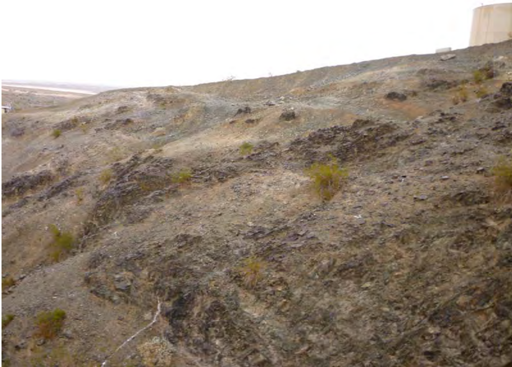
Photo 14: Post-construction view of AOC 4 from the east side of ravine.
