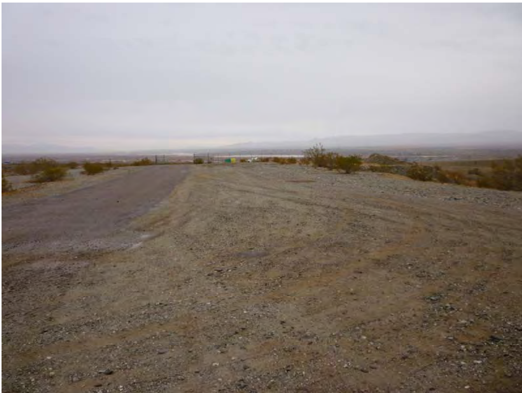
Photo 38: Post-construction view of equipment staging area at the evaporation ponds.
