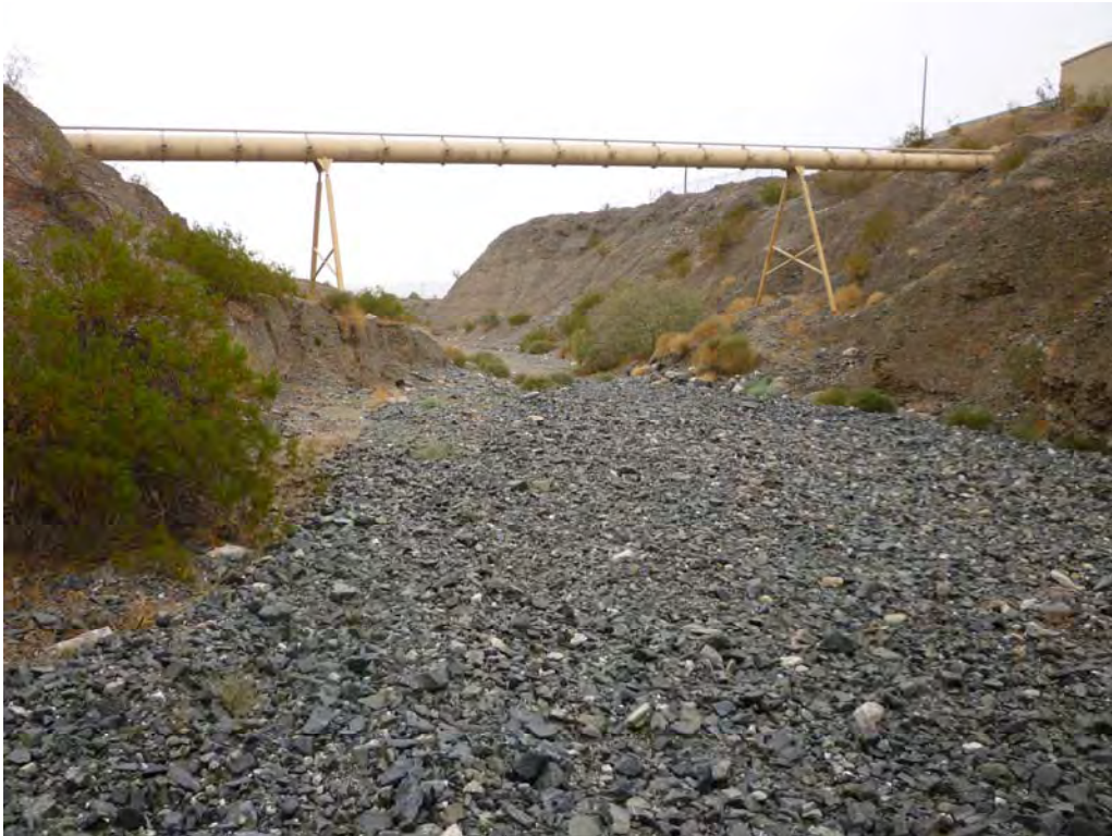
Photo 22: Post-construction view of access route to AOC 4 within Bat Cave Wash.
