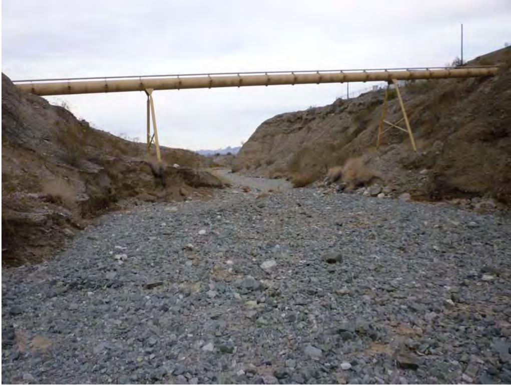
Photo 21: Pre-construction view of access route to AOC 4 within Bat Cave Wash.
