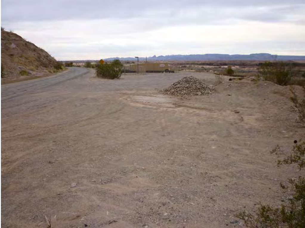
Photo 31: Pre-construction view of equipment staging area at MW-20 bench.
