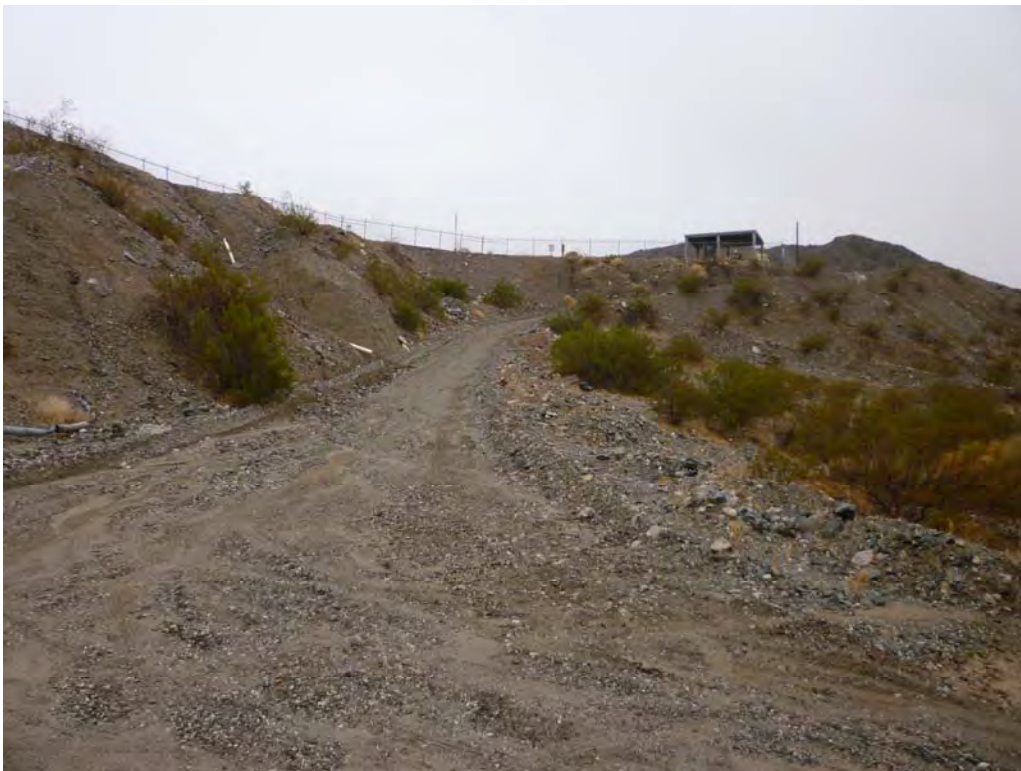
Photo 26: Post-construction view of access route to AOC 4 within Bat Cave Wash.
