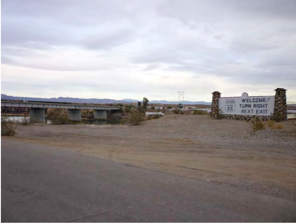
Photo 29: Pre-construction view of equipment staging area south of BNSF railroad.
