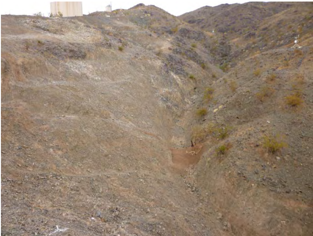
Photo 6: Post-construction view of AOC 4 from the north side of ravine.
