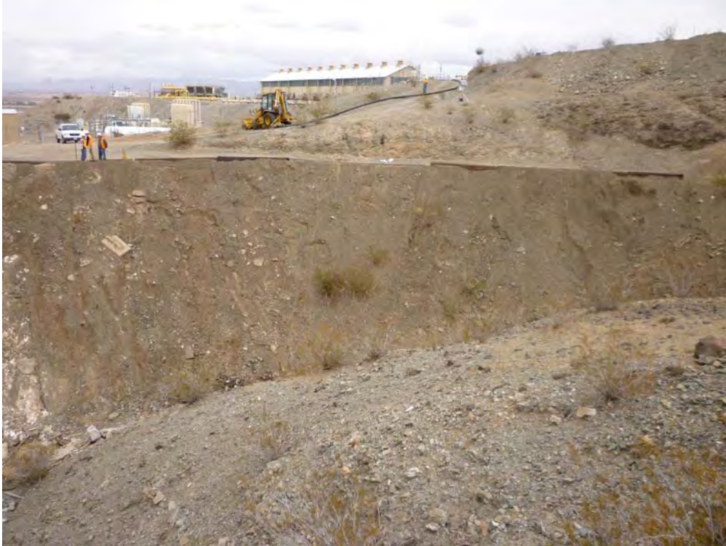
Photo 9: Post-construction view of AOC 4 from the south side of ravine.
