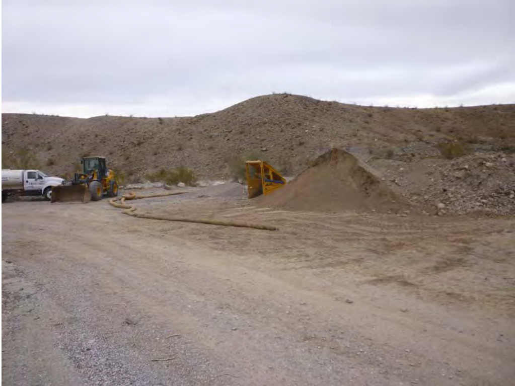
Photo 33: Pre-construction view of equipment staging area at IM3.
