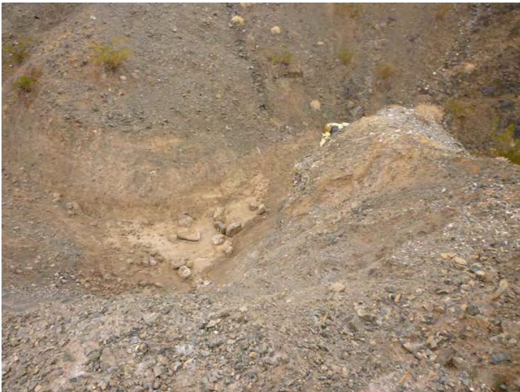
Photo 2: Post-construction view of AOC 4 from the north side of ravine.
