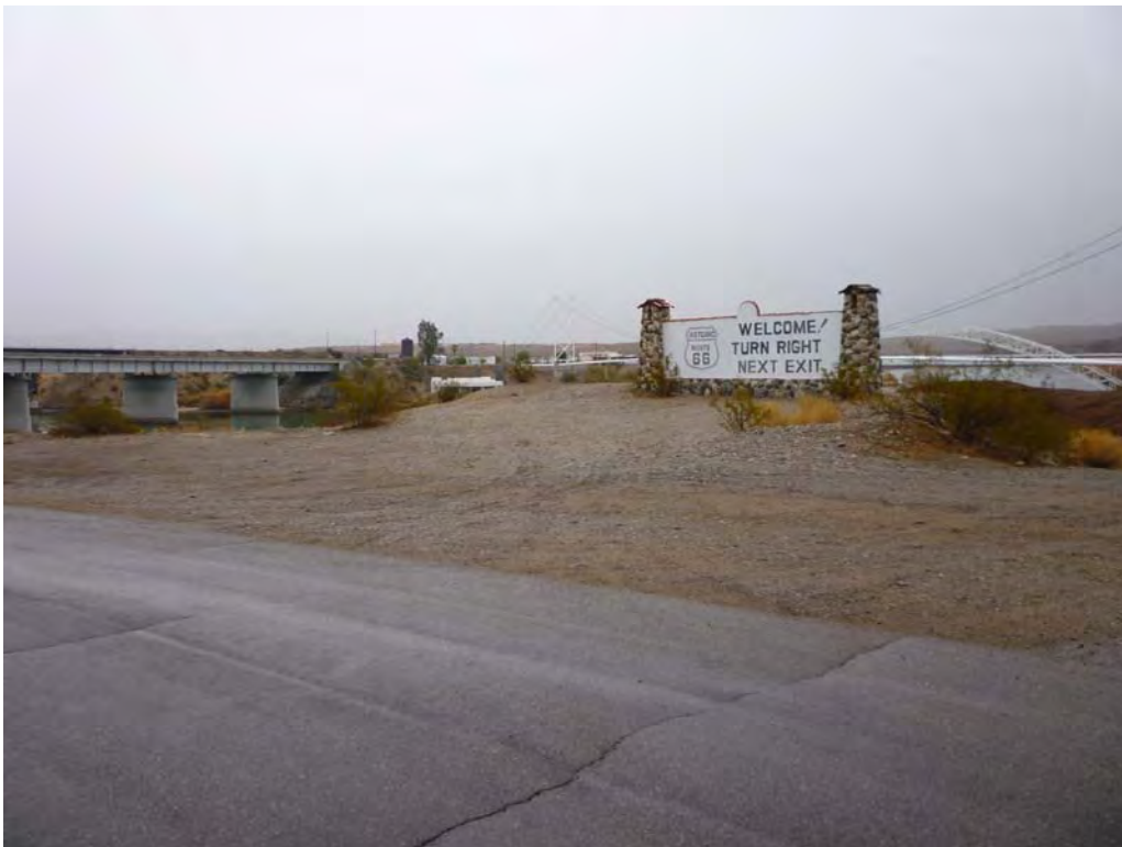
Photo 30: Post-construction view of equipment staging area south of BNSF railroad.
