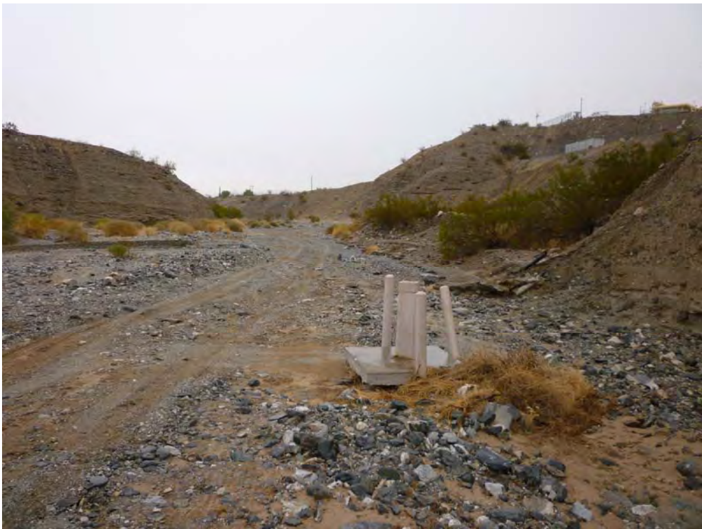
Photo 24: Post-construction view of access route to AOC 4 within Bat Cave Wash.
