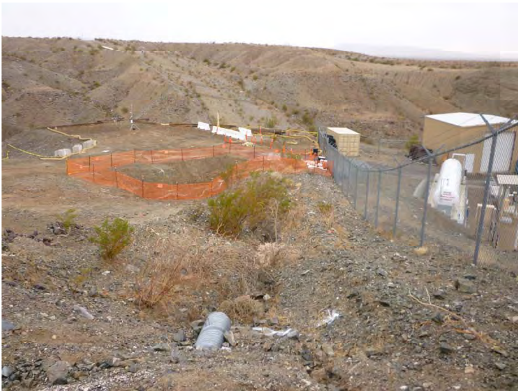
Photo 18: Post-construction view of AOC 4 from the east side of ravine.
