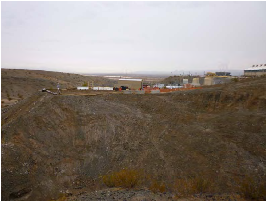
Photo 8: Post-construction view of AOC 4 from the south side of ravine.
