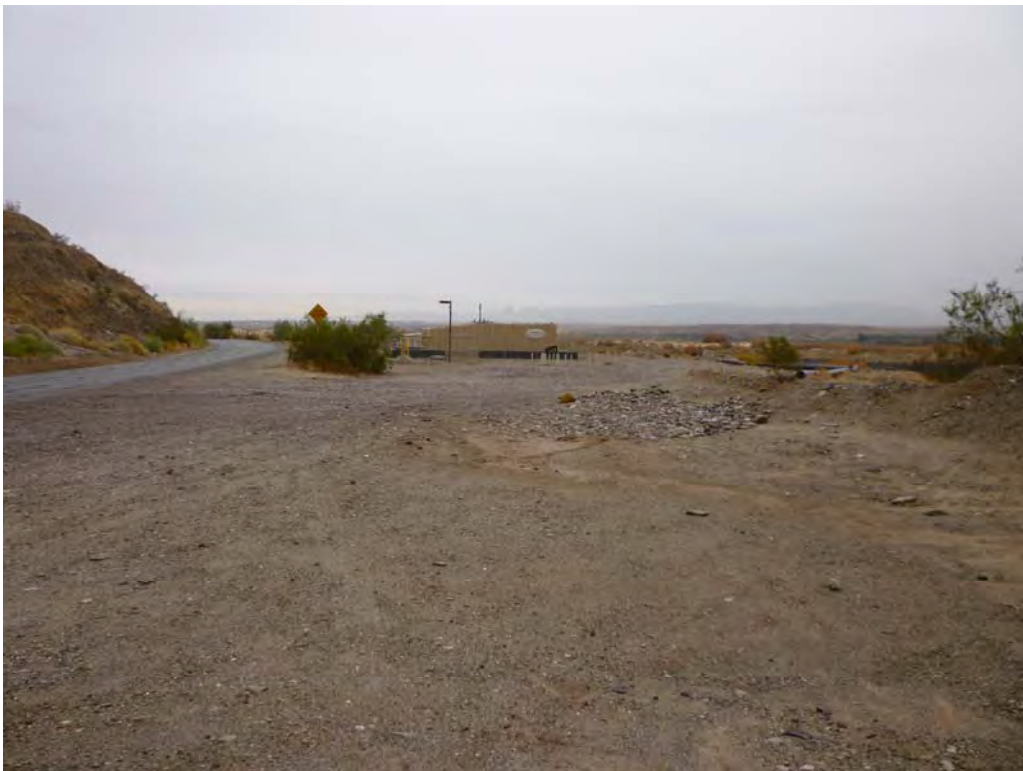
Photo 32: Post-construction view of equipment staging area at MW-20 bench.
