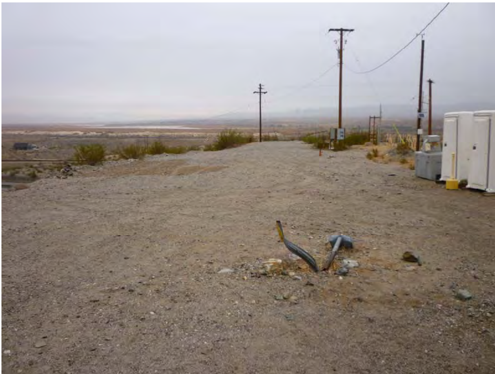
Photo 40: Post-construction view of equipment staging area north of the TCS.
