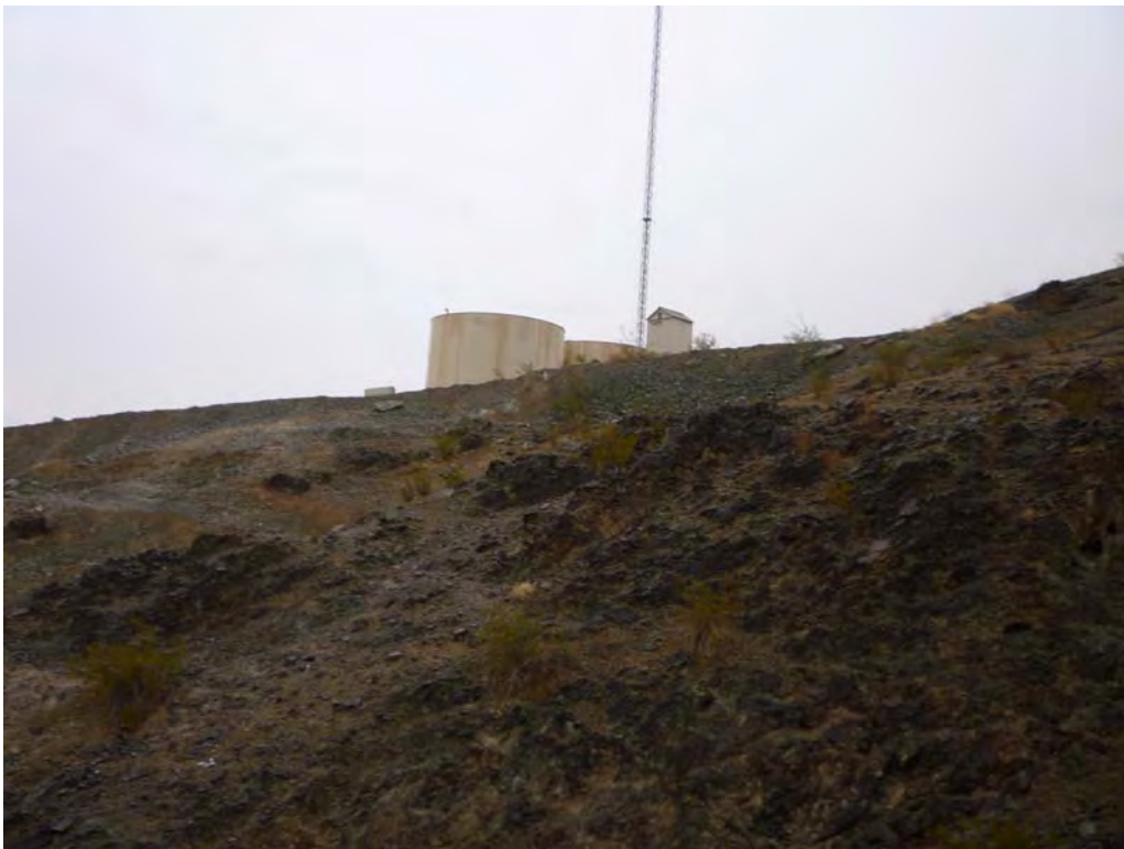
Photo 16: Post-construction view of AOC 4 from the east side of ravine.
