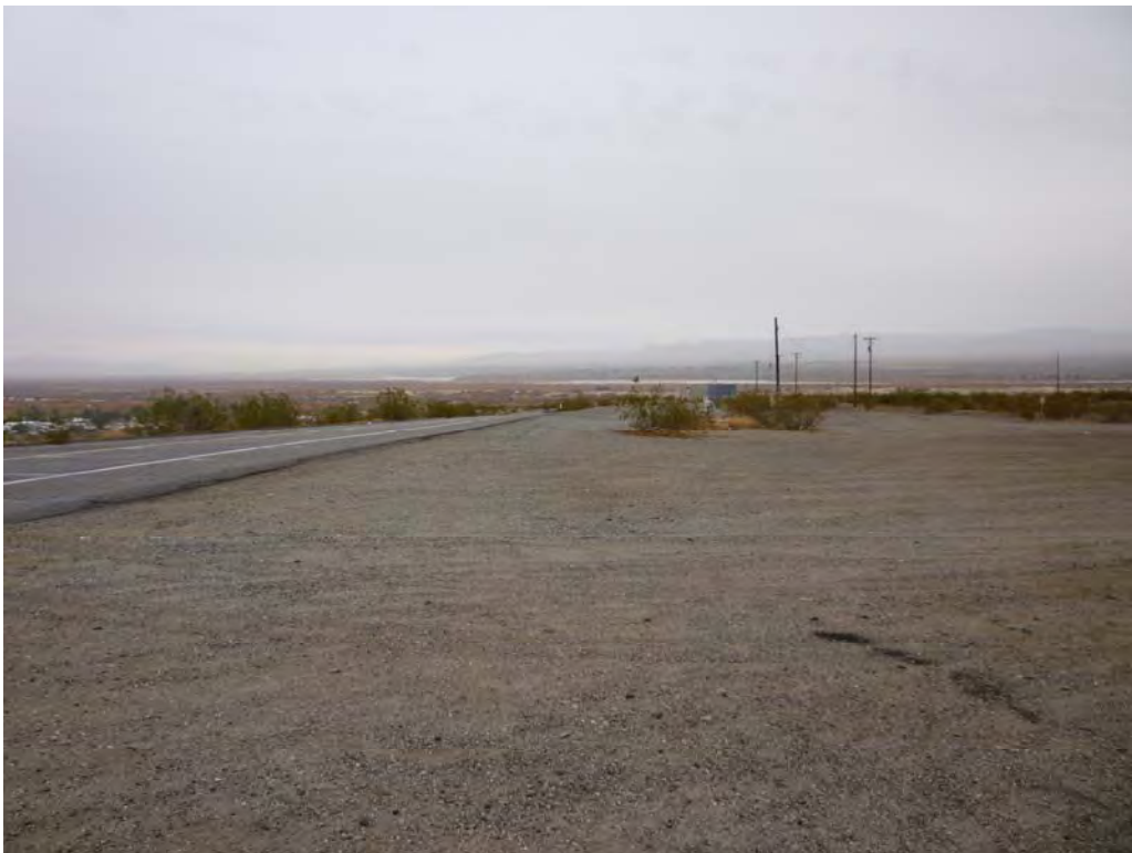
Photo 36: Post-construction view of equipment staging area next to Park Moabi Road.
