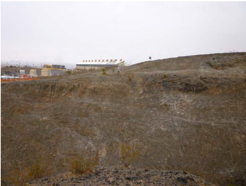
Photo 10: Post-construction view of AOC 4 from the south side of ravine.
