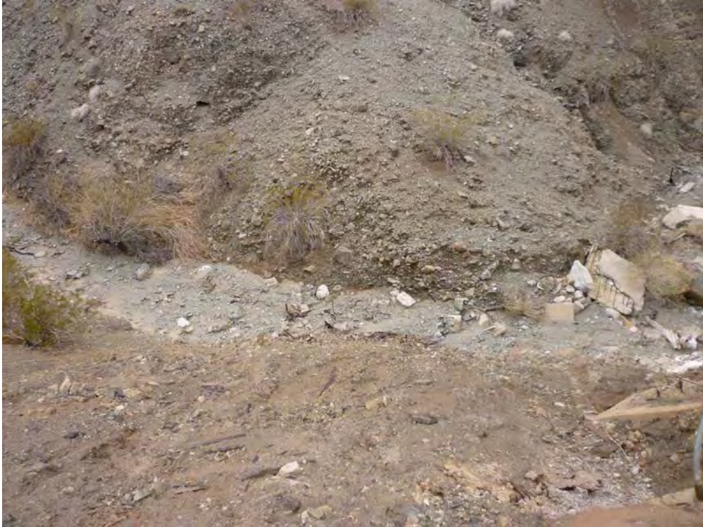
Photo 3: Pre-construction view of AOC 4 from the north side of ravine.
