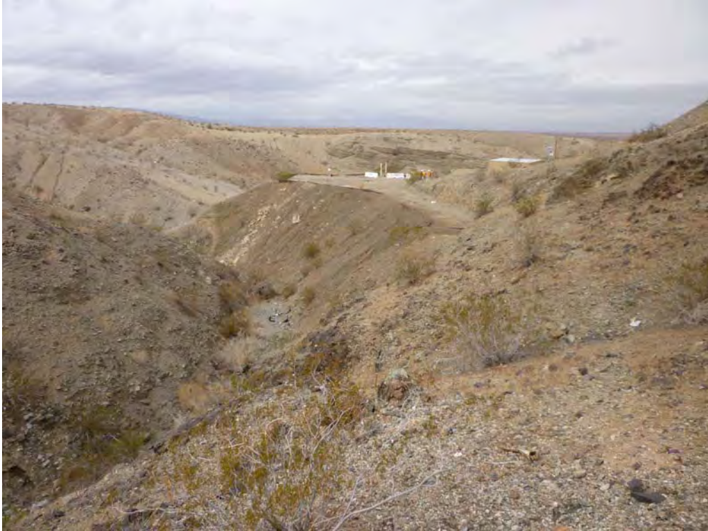
Photo 11: Pre-construction view of AOC 4 from the east side of ravine.
