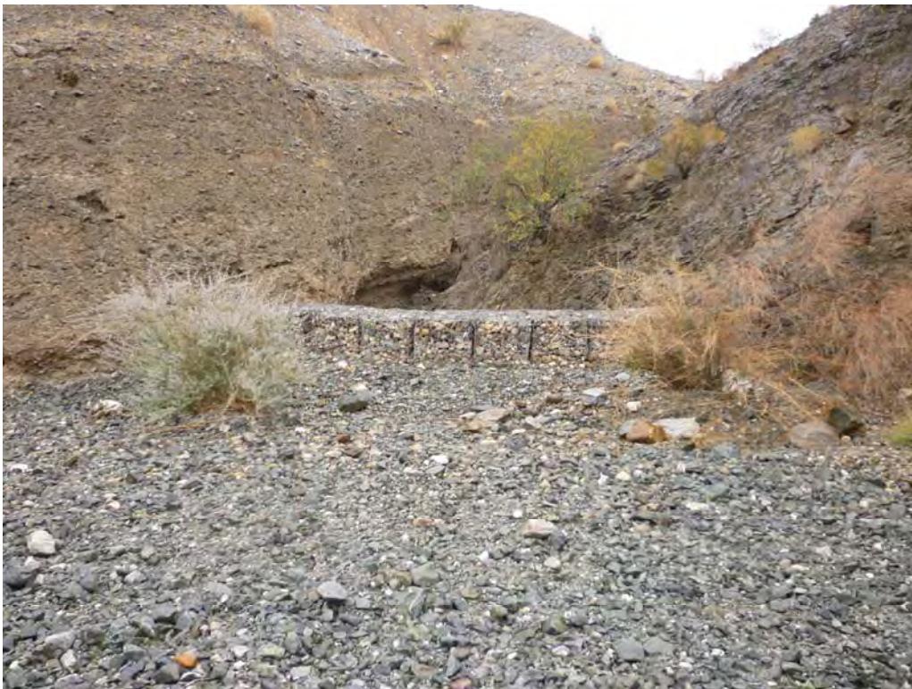
Photo 20: Post-construction view of the mouth to AOC 4 from Bat Cave Wash.
