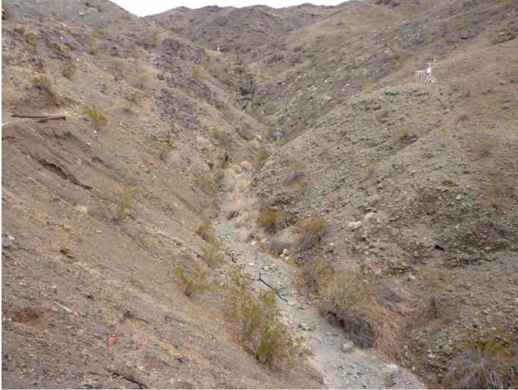
Photo 5: Pre-construction view of AOC 4 from the north side of ravine.
