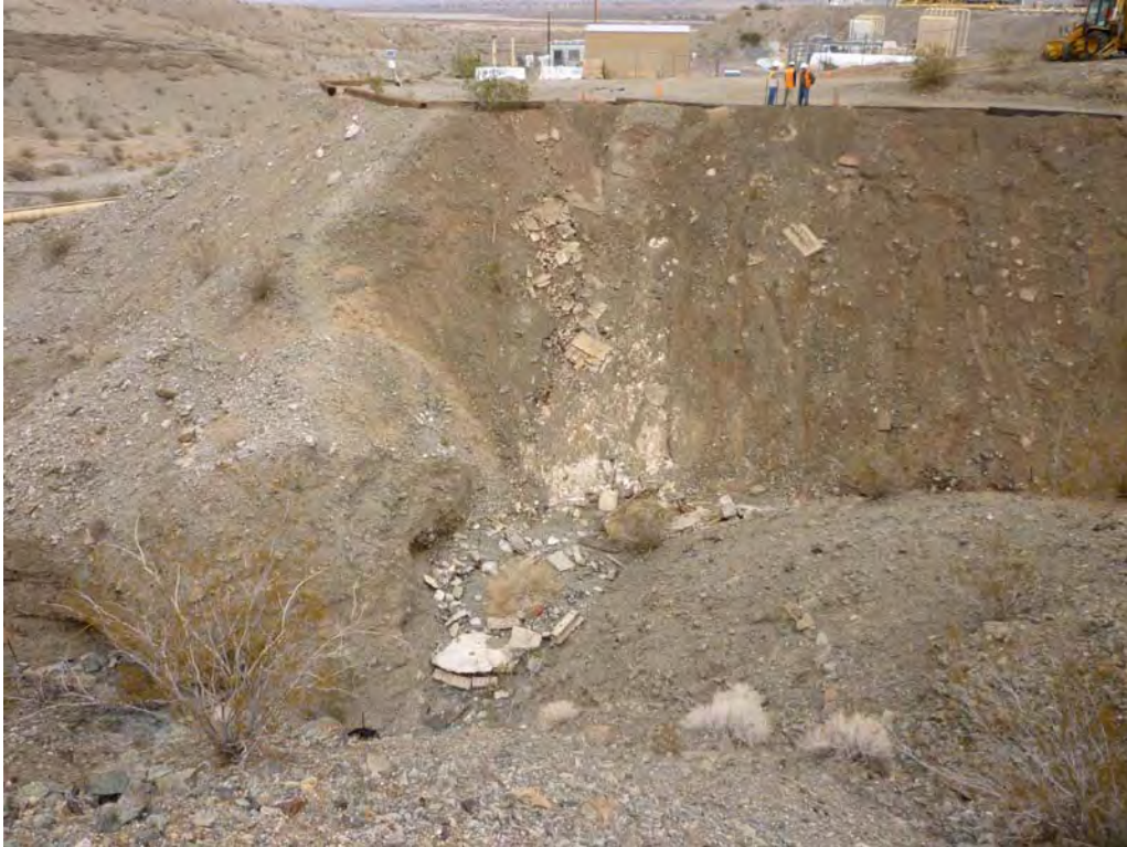
Photo 7: Pre-construction view of AOC 4 from the south side of ravine.
