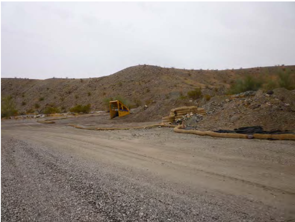
Photo 34: Post-construction view of equipment staging area at IM3.
