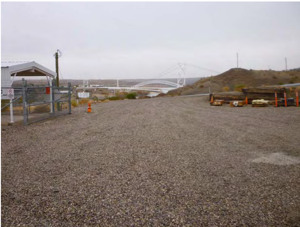
Photo 28: Post-construction view of waste management area.
