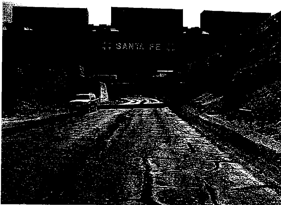
Photo No. 2 – Pavement distress cracking in SR 66 near the primary access to the MW-20 bench.
