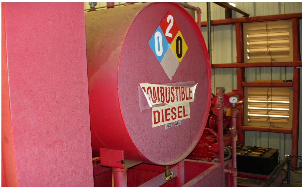
Photo 24 – Diesel Above Ground Storage Tank for Fire Water Pump
