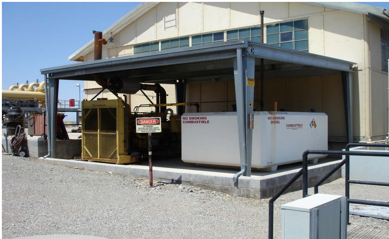
Photo 23 – Diesel Fuel Above Ground Storage Tank for Emergency Generator
