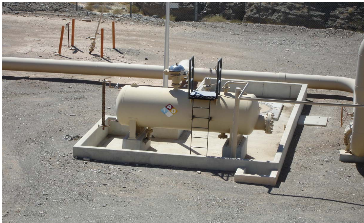
Photo 31 – Transwestern Interconnect Pipeline Fluids Above Ground Storage Tank
