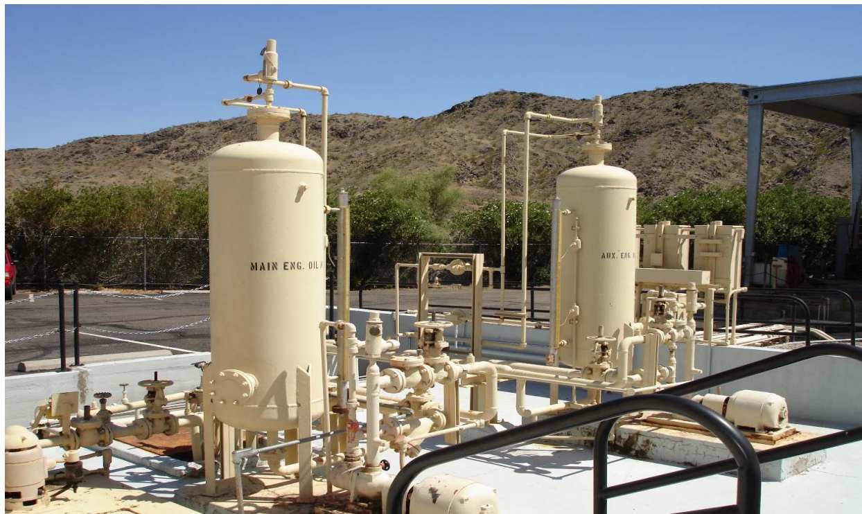
Photo 27 – Oil Transfer Tanks
