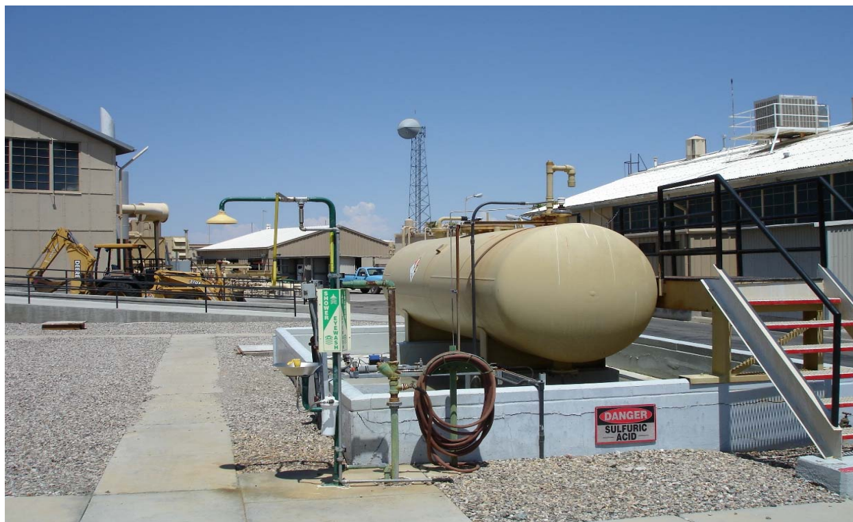
Photo 28 – Sulfuric Acid Storage Above Ground Storage Tank
