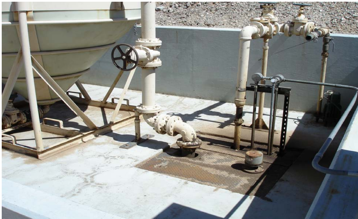
Photo 19 – Oil/Water Separator System Grit Tank Sump
