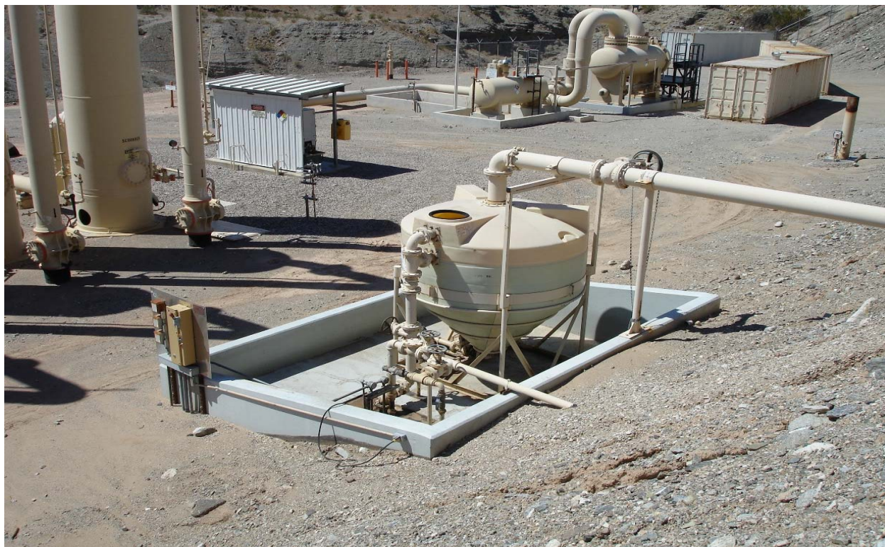
Photo 20 – Oil/Water Separator System Above Ground Grit Tank
