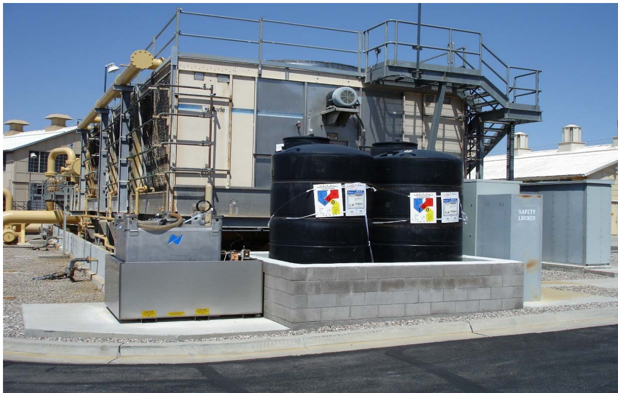
Photo 33 – Water Treatment Chemical Storage Above Ground Storage Tanks
