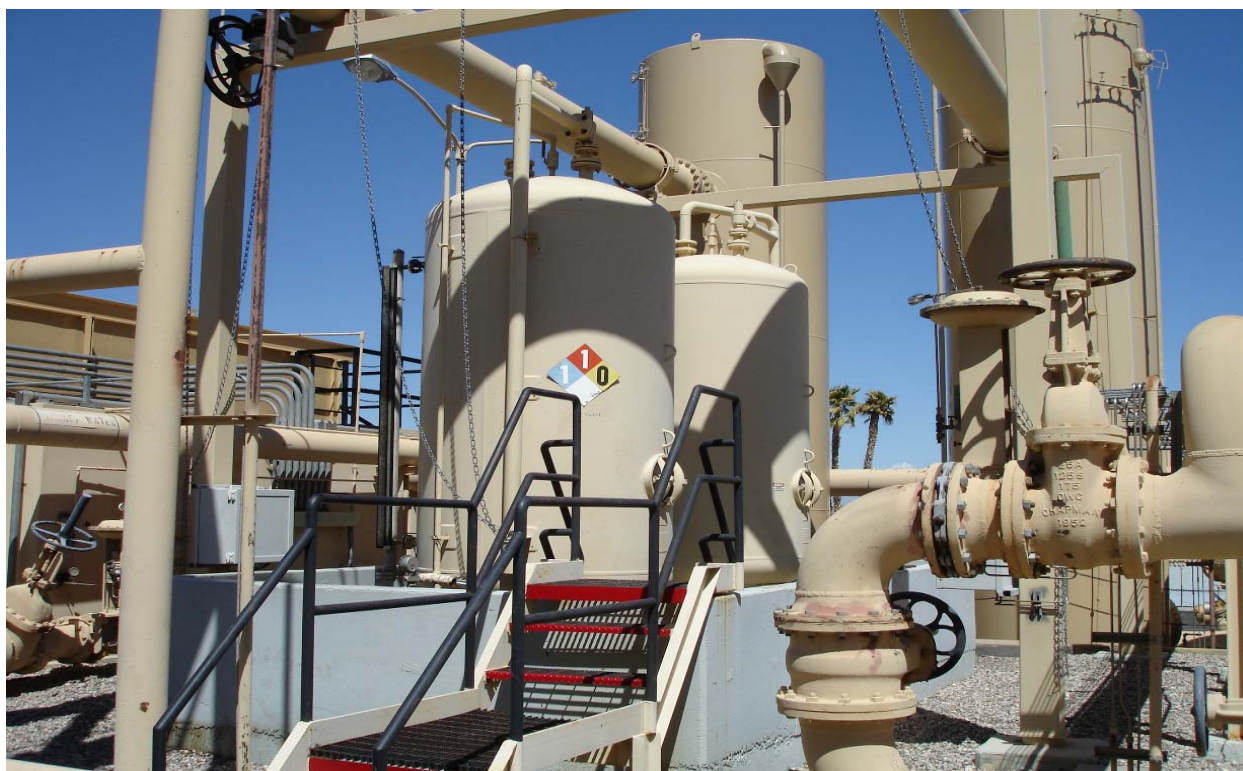
Photo 26 –Temporary Compressor Engine Oil Holding Above Ground Storage Tanks
