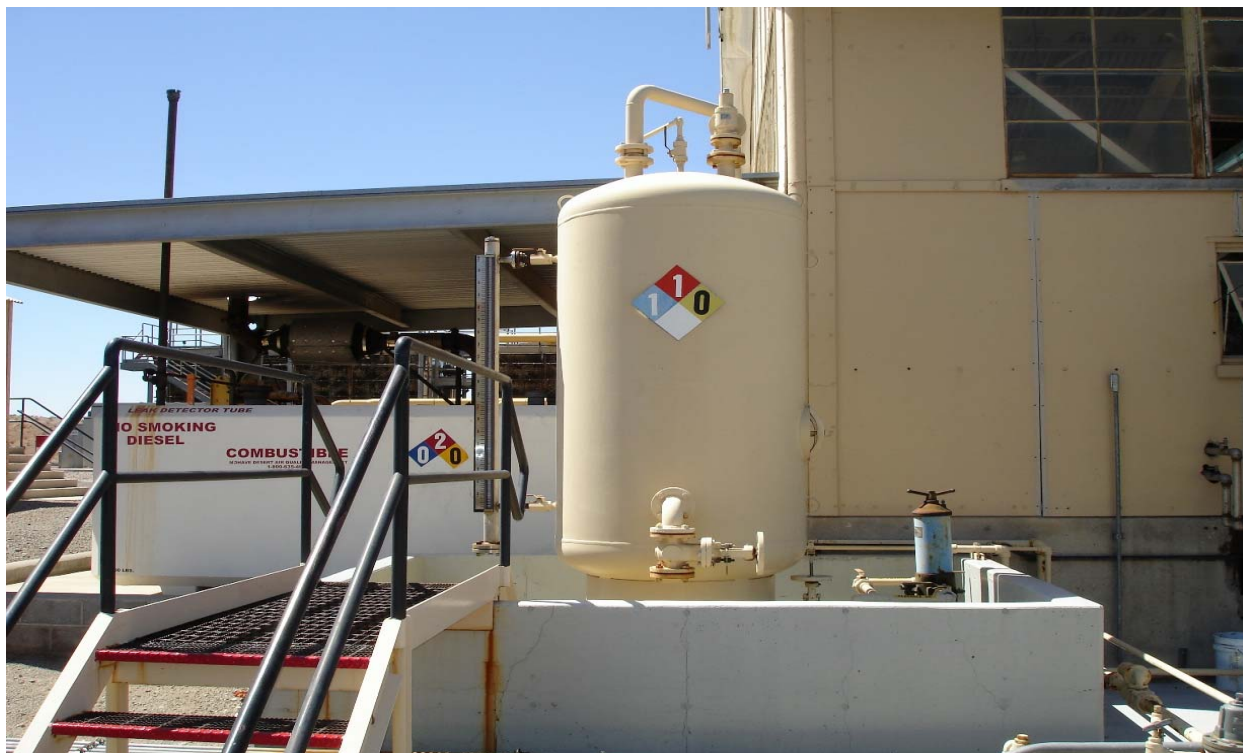
Photo 25 –Temporary Generator Engine Oil Holding Above Ground Storage Tank
