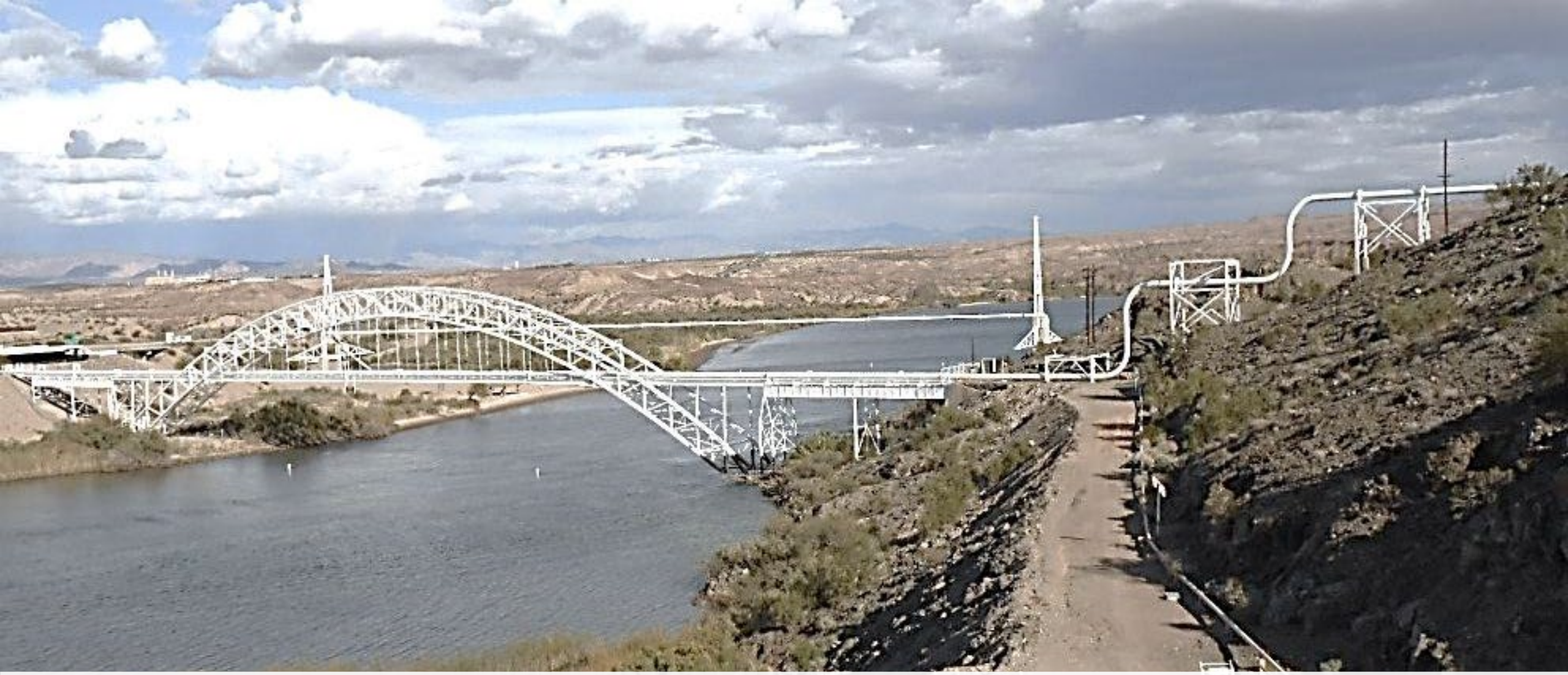
Route 66 with Old Trails Arch Bridge
