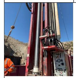
8/20/2022 – TWB-03: Installing 316L Stainless Steel, 18-slot Wire Wrap Screen (#2)
