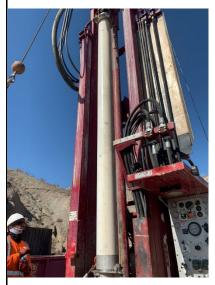
8/20/2022 – TWB-03: Installing Shur-Grip SDR-17 PVC casing (#3)
