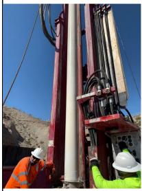
8/20/2022 – TWB-03: Installing Shur-Grip SDR-17 PVC casing (#5)
