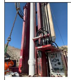
8/20/2022 – TWB-03: Centralizer set at approximately 38 ft. bgs. on Shur-Grip SDR-17 PVC casing (#4)
