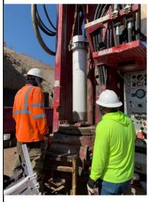
8/20/2022 – TWB-03: Installing stainless steel endcap and Shur-Grip SDR-17 PVC sump (#1)
