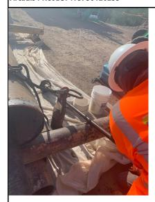
8/21/2022 – TWB-03: Swab tool used to swab screen for approximately 30 minutes in order to promote settling of the filter
