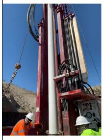
8/20/2022 – TWB-03: Installing Shur-Grip SDR-17 PVC casing (#4)
