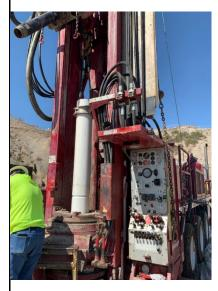
8/20/2022 – TWB-03: Installing temporary PVC Shur-Grip SDR-17 PVC stickup
