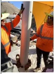
9/27/2022 – TWB-03: Conducting the "Dummy Tool" alignment test
