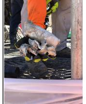
Core Depth: 17 to 27 SCH 80 PVC removed by overdrilling Date: 8/16/2022
