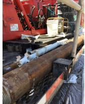
Core Depth: 44 to 54 Description: TWB-01-Temp Well 2-inch diameter SCH 80 PVC removed by overdrilling Date: 8/17/2022
