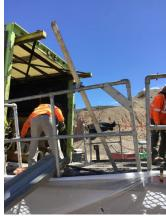
Core Depth: 27 to 34 Description: TWB-01-Temp Well 2-inch diameter SCH 80 PVC removed by overdrilling Date: 8/16/2022
