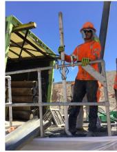
Core Depth: 17 to 27 Description: TWB-01-Temp Well 2-inch diameter Description: TWB-01-Temp Well 2-inch diameter SCH 80 PVC removed by overdrilling Date: 8/16/2022
