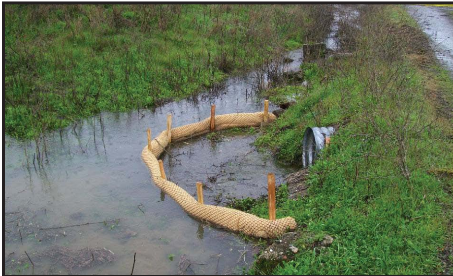
Fiber roll protecting a discharge from a construction site.
