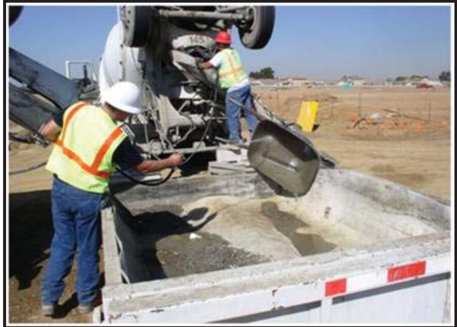
Self contained concrete washout.
