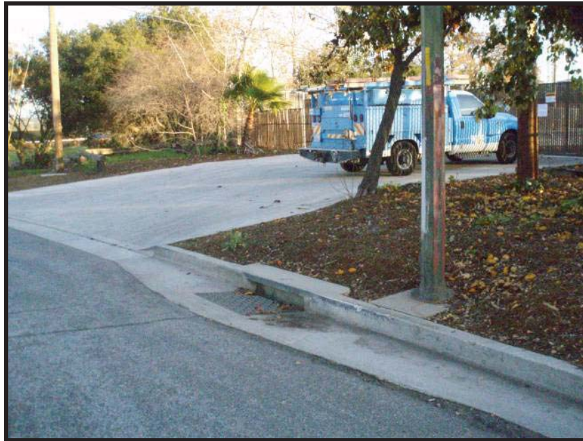
Wood mulch applied to exposed soil areas along with vegetation plantings.
