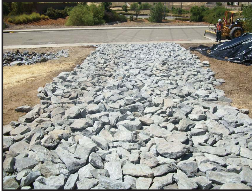
Gravel over geotextile fabric (tracking control).
