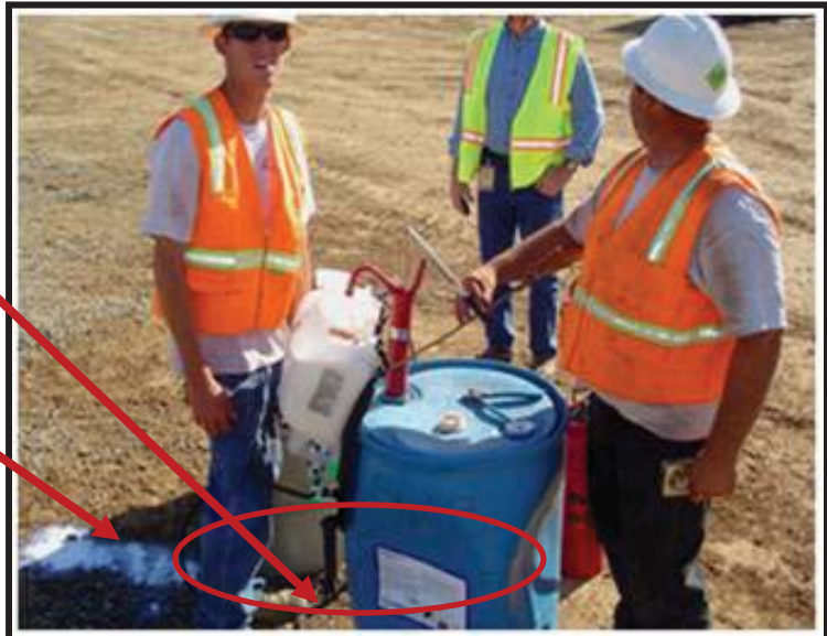
Example of improper use of materials. Missing secondary containment and spill kit.
