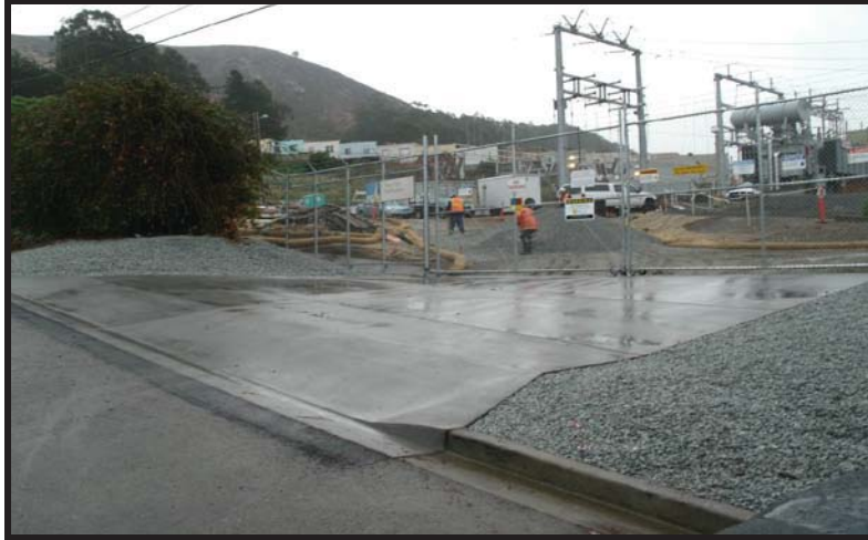
Clean and well maintained construction entrance/exit.
