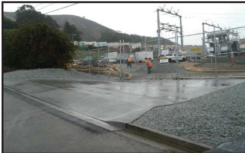
Clean and well maintained construction entrance/exit.
