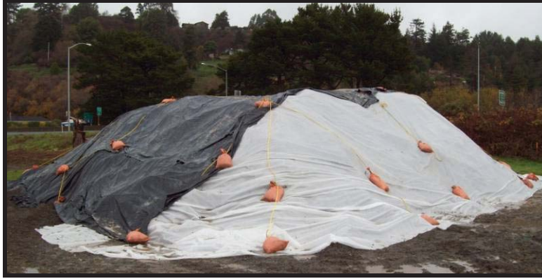
Proper securing of plastic sheeting.
