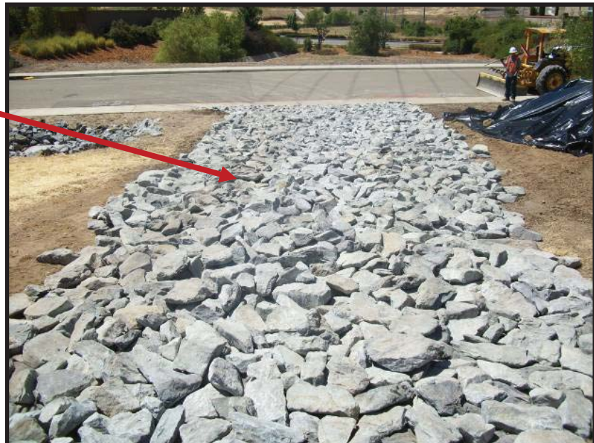
Traditional rocked construction entrance/exit.
