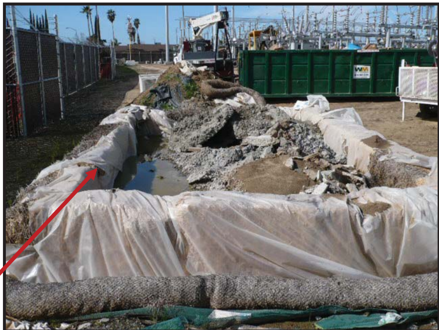
Lined concrete washout.
