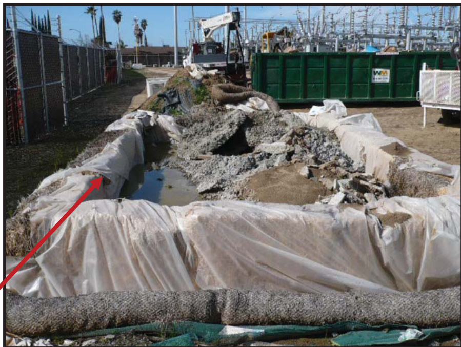
Lined concrete washout.
