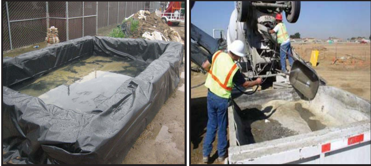
Two alternatives for containing concrete washout water.
