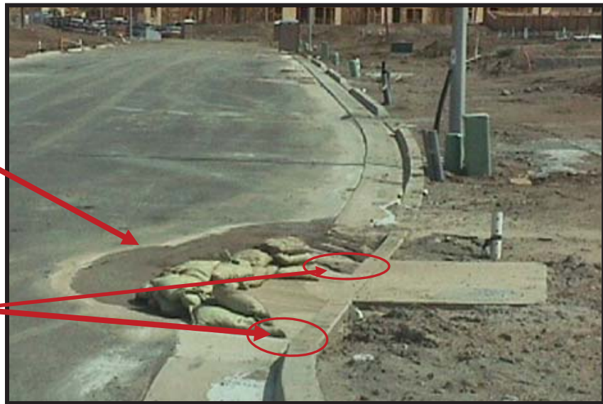
Gravel bag inlet protection slows flow and filters sediment from drainage.
