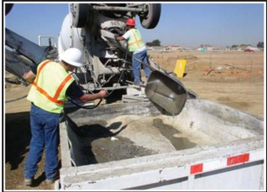
Self contained concrete washout.
