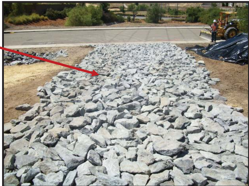
Traditional rocked construction entrance/exit.
