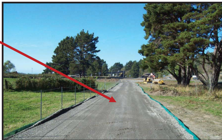
Stabilized construction road.
