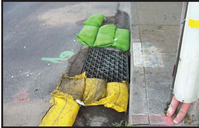
Gravel bags applied for storm drain inlet protection.
