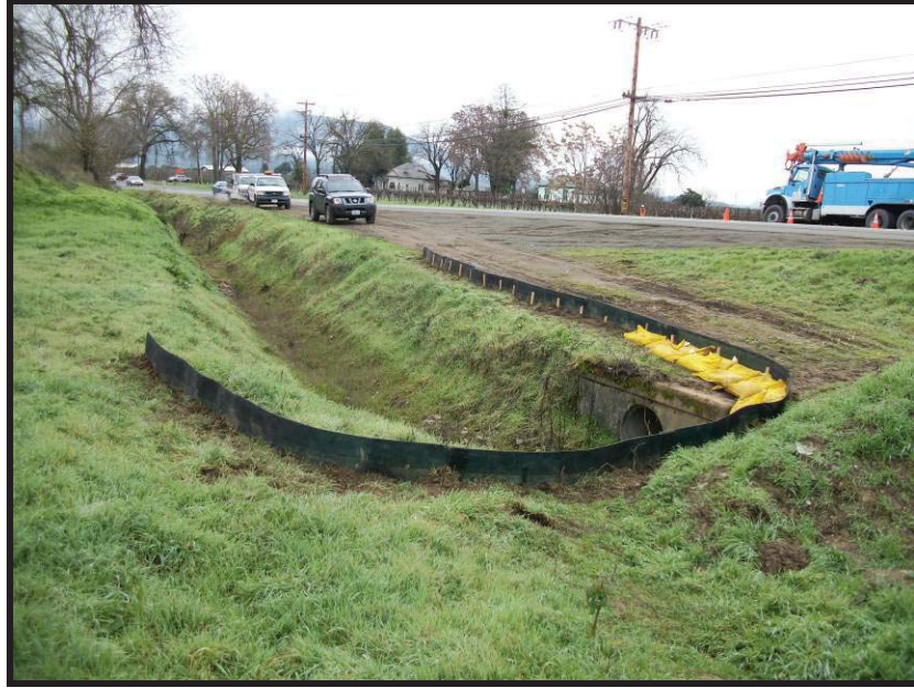
Silt fence protecting a drainage channel.
