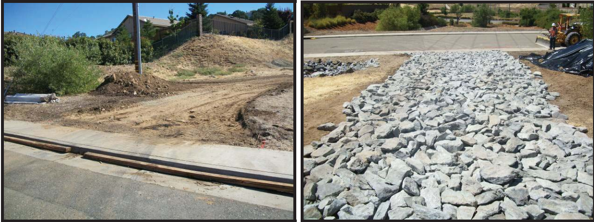
Construction entrance/exit before and after installation of gravel over geotextile fabric tracking control.
