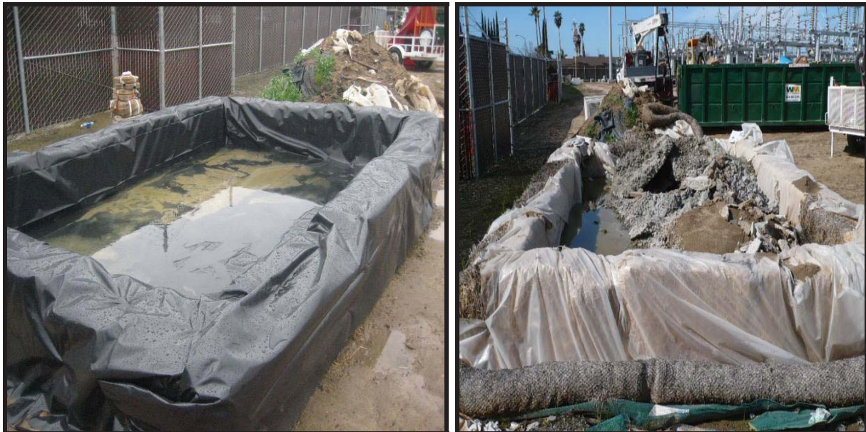
Properly implemented concrete waste management containments.
