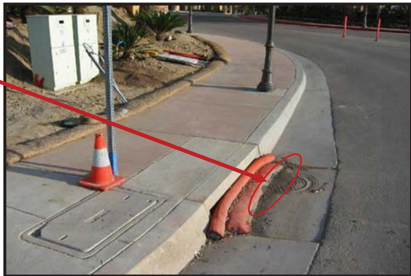
Curb inlet protection that blocks flow is good for preventing non-storm water discharges from entering the drain.
