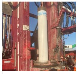
6/25/2022 – TCS-01: 10-inch Shur-Grip SDR-17 PVC casing stickup installation (#17)
