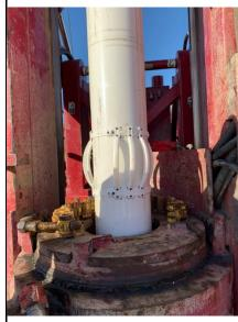
6/25/2022 – TCS-01: 10-inch Shur-Grip SDR-17 PVC casing installation centralizer set at approximately 120' bgs (#10)
