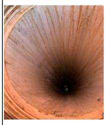
7/9/2022 – TCS-01: Inside of well checked after boulder fell into borehole, no issues/damage observed
