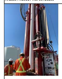
6/25/2022 – TCS-01: 10-inch Shur-Grip SDR-17 PVC casing installation (#14)
