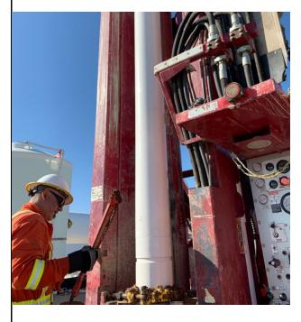
6/25/2022 – TCS-01: 10-inch Shur-Grip SDR-17 PVC casing installation (#15)
