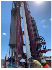
6/24/2022 – TCS-01: 10-inch Shur-Grip SDR-17 PVC casing installation (#8)
