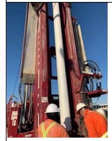
6/25/2022 – TCS-01: 10-inch Shur-Grip SDR-17 PVC casing installation (#9)
