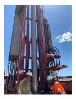
6/24/2022 – TCS-01: 10-inch 18-slot Stainless Steel 316L Wire Wrap Screen installation (#4)
