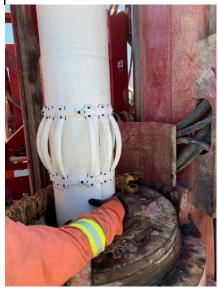
6/24/2022 – TCS-01: 10-inch Shur-Grip SDR-17 PVC casing installation with centralizer set at approximately 160' bgs (#8)
