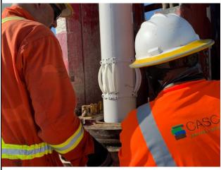
6/25/2022 – TCS-01: 10-inch Shur-Grip SDR-17 PVC casing installation with centralizer set at approximately 45' bgs (#14)
