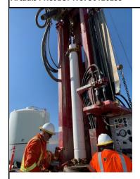
6/25/2022 – TCS-01: 10-inch Shur-Grip SDR-17 PVC casing installation (#16)
