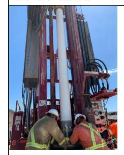
6/24/2022 – TCS-01: 10-inch Shur-Grip SDR-17 PVC casing installation (#5)
