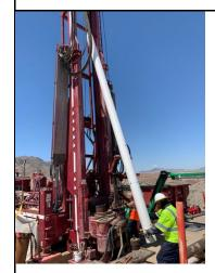
6/28/2022 – TCS-01: Hoisting "Dummy Tool" for preliminary alignment test
