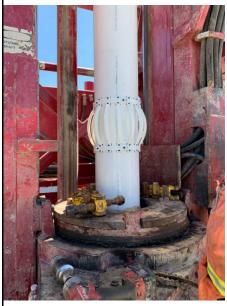
6/24/2022 – TCS-01: 10-inch Shur-Grip SDR-17 PVC casing installation with centralizer set at approximately 210' bgs, (#5)
