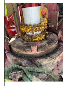
6/24/2022 – TCS-01: 10-inch Shur-Grip SDR-17 PVC casing installation (#6)
