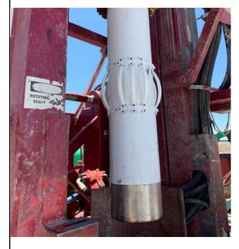
6/24/2022 – TCS-01: End cap and sump with centralizer set at approximately 272' bgs (#1)
