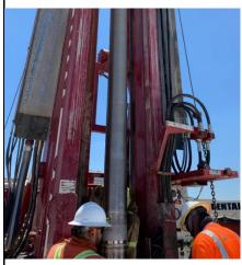
6/24/2022 - TCS-01: 10-inch 18-slot Stainless Steel 316L Wire Wrap Screen installation (#3)
