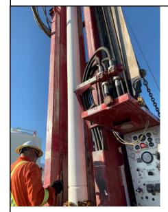
6/25/2022 – TCS-01: 10-inch Shur-Grip SDR-17 PVC casing installation (#12)
