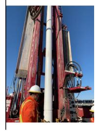
6/25/2022 – TCS-01: 10-inch Shur-Grip SDR-17 PVC casing installation (#13)
