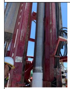
6/24/2022 – TCS-01: 10-inch 18-slot Stainless Steel 316L Wire Wrap Screen installation (#2)
