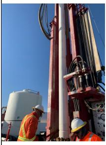
6/25/2022 – TCS-01: 10-inch Shur-Grip SDR-17 PVC casing installation (#10)
