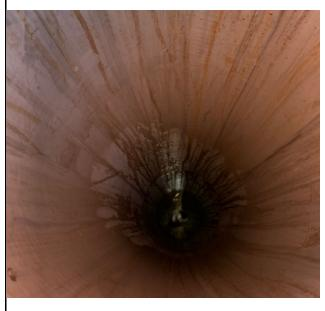
7/9/2022 – TCS-01: Inside of well checked after boulder fell into borehole, no issues/damage observed
