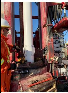
6/25/2022 – TCS-01: 10-inch Shur-Grip SDR-17 PVC casing installation with centralizer set at approximately 80' bgs (#12)
