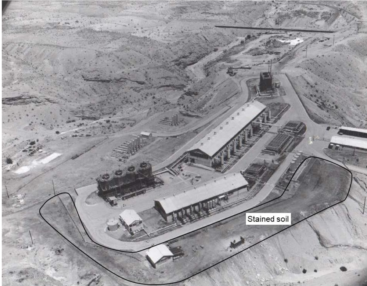
Photograph 4.2.10-1: May 19, 1955, Aerial Photograph 2, Topock Compressor Station Note: Facing northwest. Dark staining visible on eastern side of the TCS.
