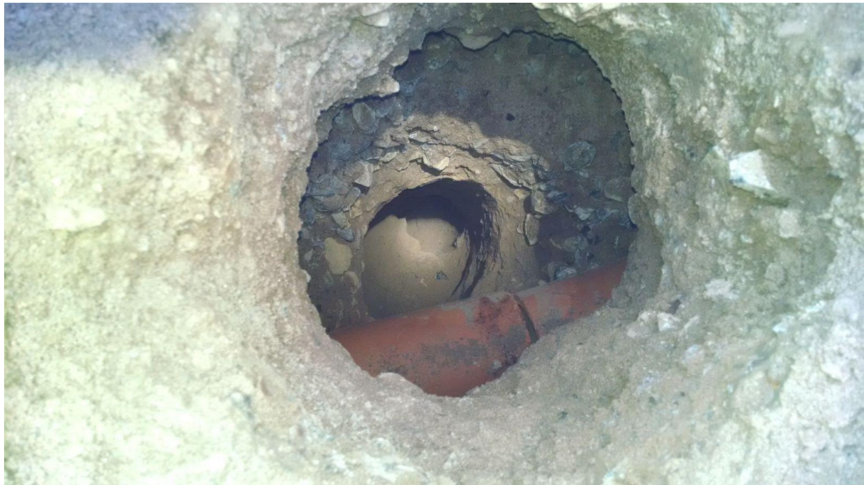
Photograph 4.2.13-4: December 2015 Photograph of Leach Lines Located Approximately 4 feet bgs.
