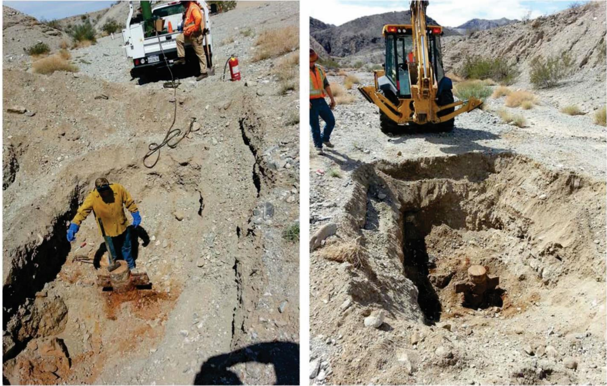
Photographs 4.1.1-5 and 4.1.1-6: September 2013 TCS-4 Excavation
