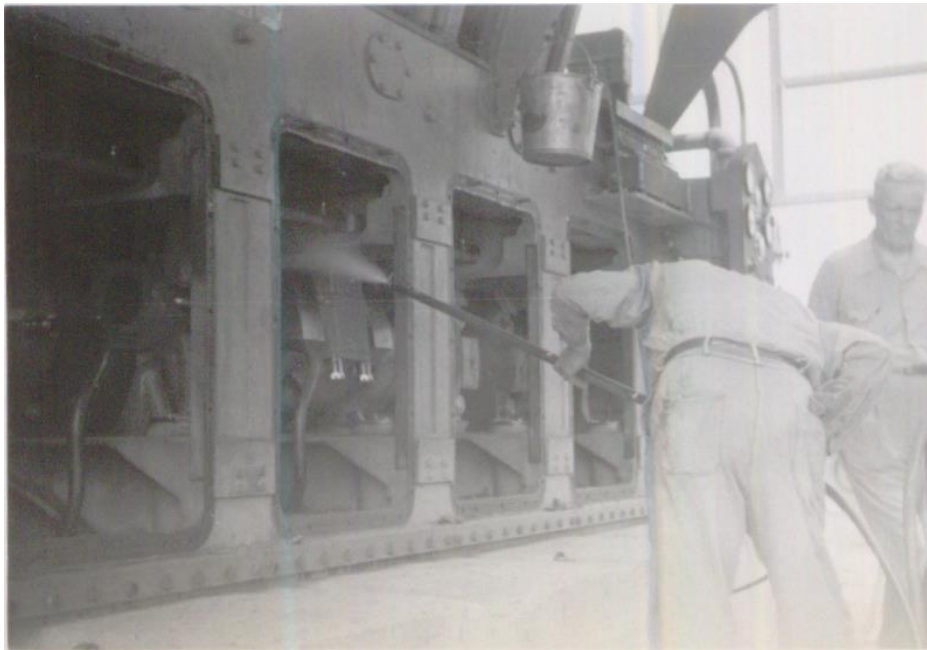
Photograph 4.2.21-6: August 1, 1951, Construction Photograph, Engine Cleaning
