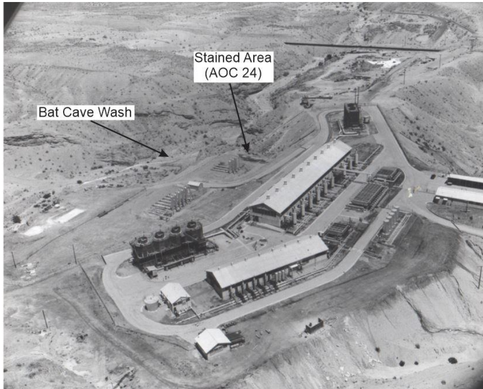
Photograph 4.2.20-1: May 19, 1955, Aerial Photograph 2, AOC 24 Note: Facing northwest. Elongated area of staining visible in AOC 24.
