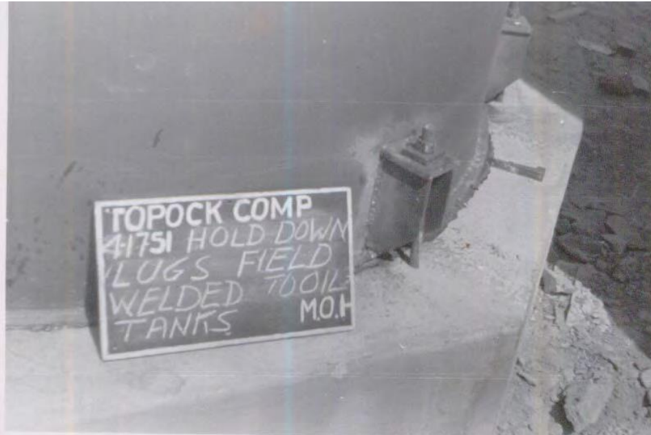
Photograph 4.2.23-2: April 17, 1951, Foundation of an Oil Storage Tank at Installation.
