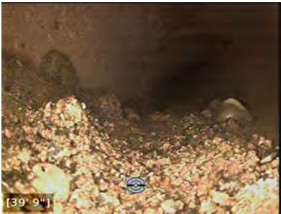
Debris Red clay pipe.
