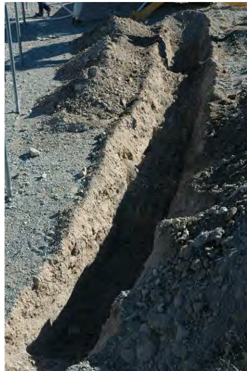
Photo 3: AOC12B-T1 central view west
