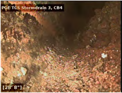
Photo coming out of pipe.
