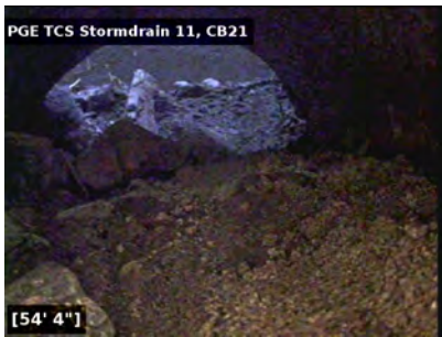
Debris inside pipe downstream of Catch Basin 22.
