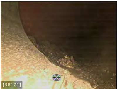
Transition from red clay pipe to gray PVC.
