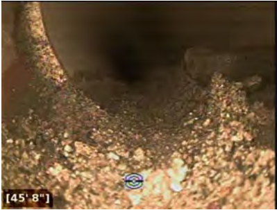
Transition back to red clay pipe (there is a similar photo above when the camera was moving towards CB-22).
