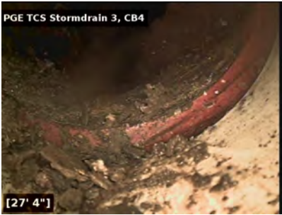
Transition from 4" red clay pipe to white PVC pipe.
