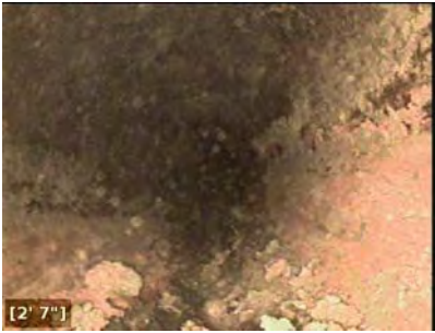
Pipe is 8" diameter red clay pipe.
