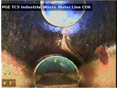
View looking back towards the cleanout access and north down the "main line". The main line is believed to be capped ~3' north of the cleanout.
