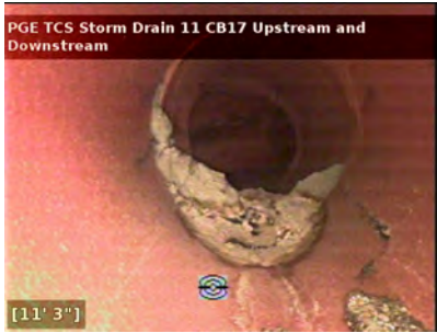
Clay pipe with grout intruding into pipe.
