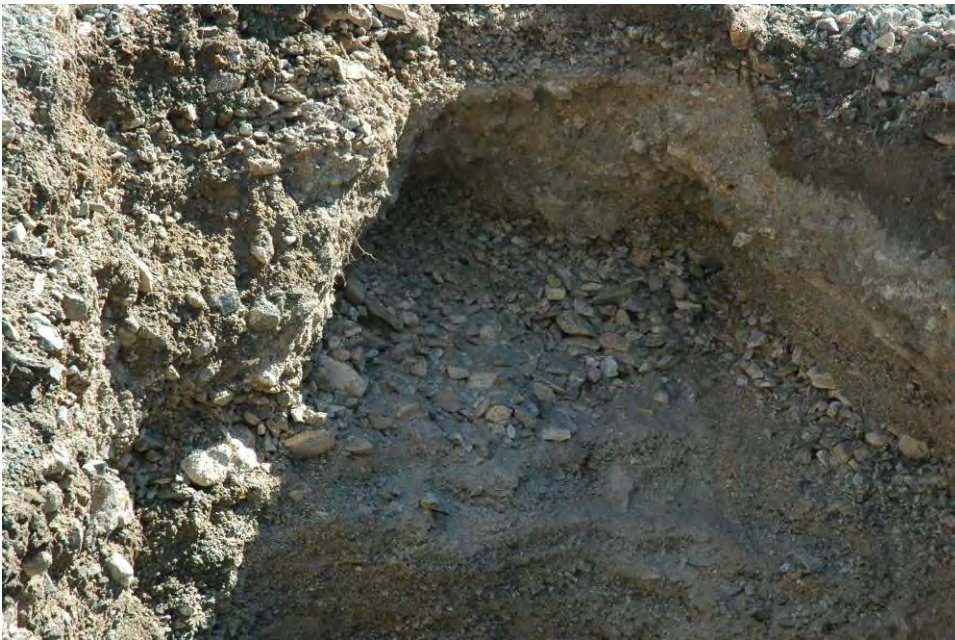
Photograph 16: Trench SWMU1-WP-5h trench top
