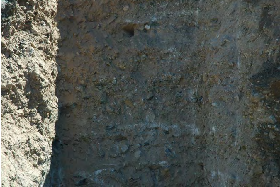
Photograph 5: SWMU1-WP-1h trench middle
