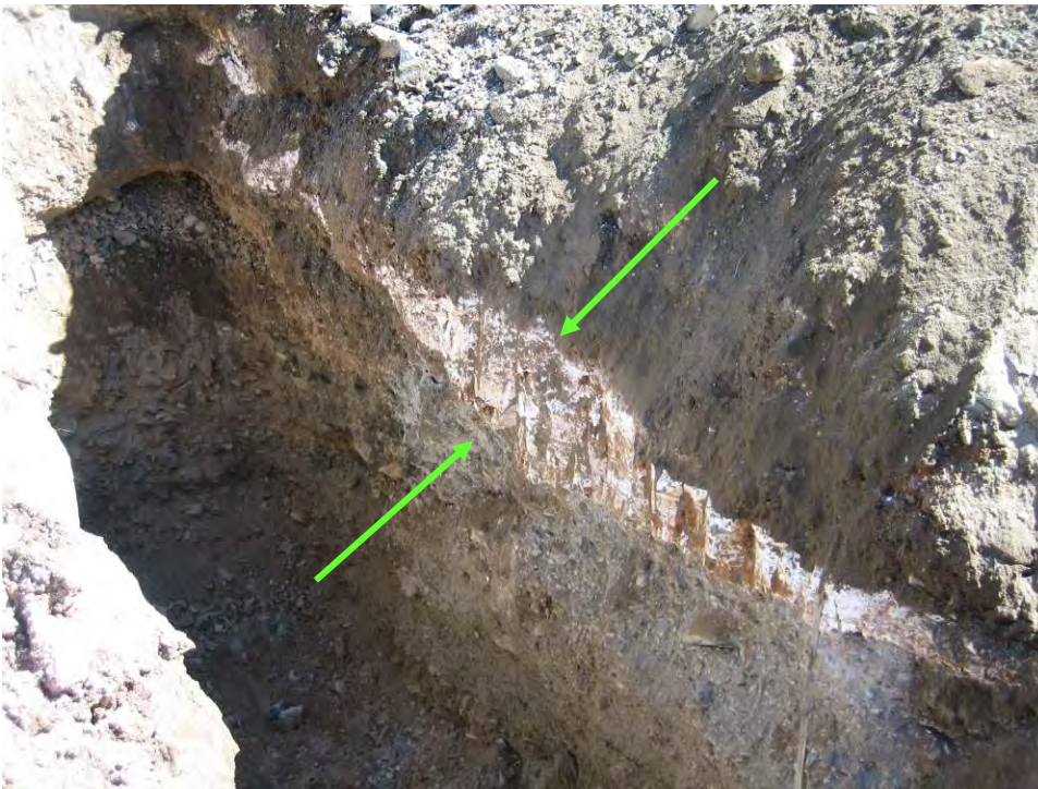
Photograph 20: Trench SWMU1-WP-7 south sidewall. Note white chalky material.
