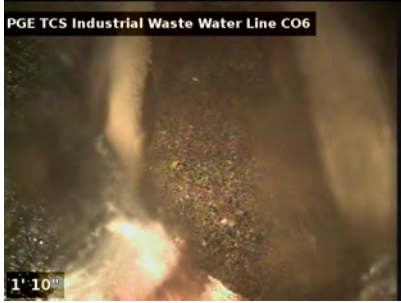
View of camera entering the "main line".
