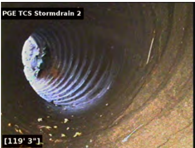
A "45" junction near the outfall.
