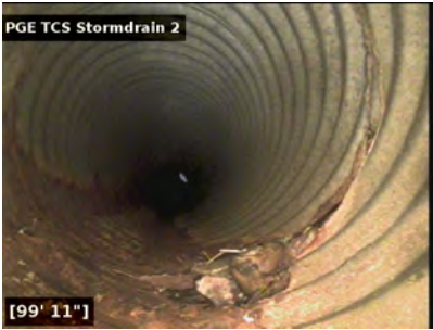
Corroded steel pipe with possible holes at the bottom of the pipe.
