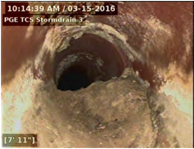
Small debris for very short distance.
