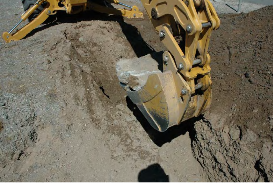
Photo 7: AOC12c-T1 east part of trench concrete chunk
