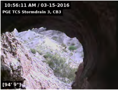
Storm Drain 3 outfall.
