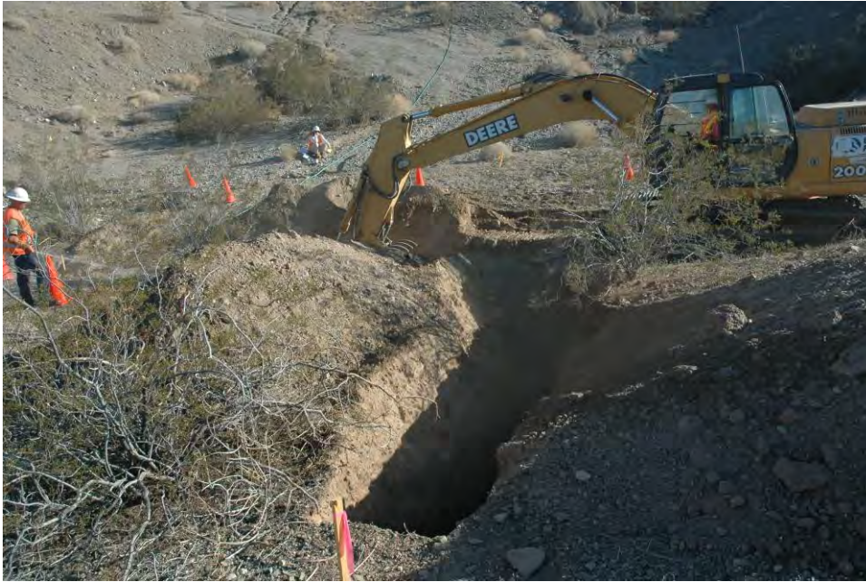
Photo 1: Digging central region of AOC12a-T1 with AOC12a-T2 in foreground
