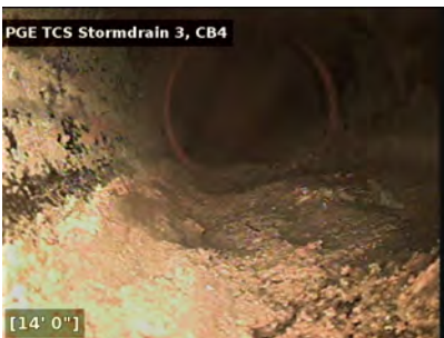
Red clay pipe, free of debris.
