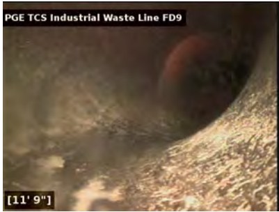
Elbow that directs flow towards the main line, in a north direction.
