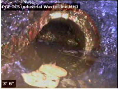
View as camera was removed from downstream pipe.
