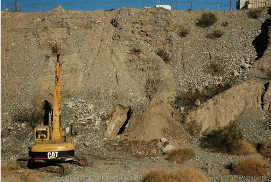
Photograph 27: Trench SWMU1-WP-10 Trench
