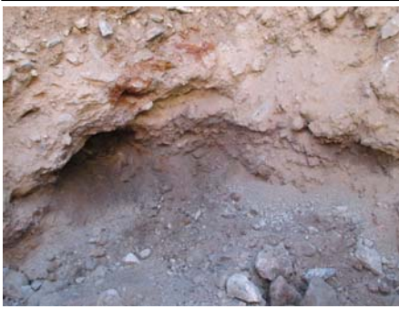
Debris at Trench AOC14-14.
