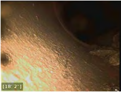
Pipe free of debris.
