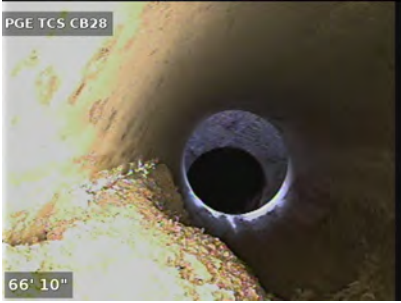
View of outfall from CB28 pipe into CB30.
