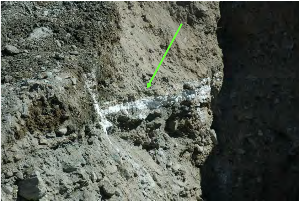
Photograph 10: Trench SWMU1-WP-3h North sidewall. Note white powdery material.
