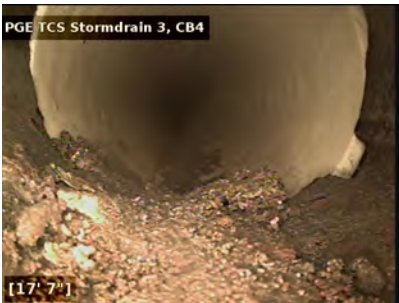
Transition from PVC to red clay pipe.
