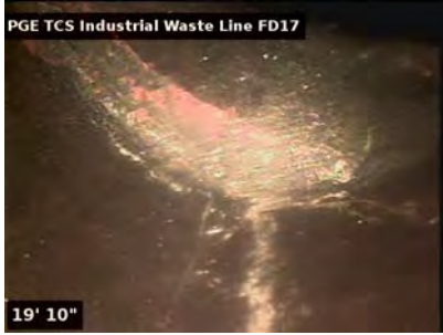
View of main line. End of survey.
