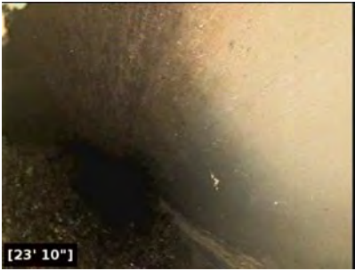
Sand and gravel debris.
