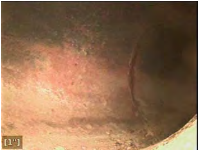
Camera traveling through the sharp right, westward turn towards CB-25.
