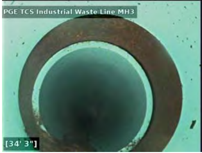
PVC/steel elbow
