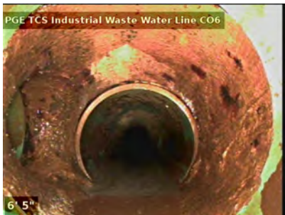
"T" junction where the north floor drain of the south cooling tower discharges into the main line.
