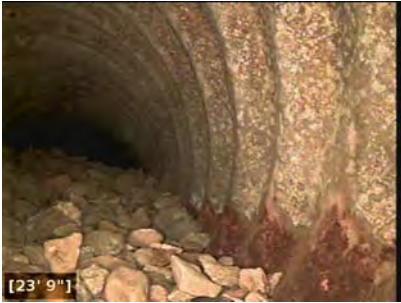
End of the survey due to the gravel inside of the pipe.
