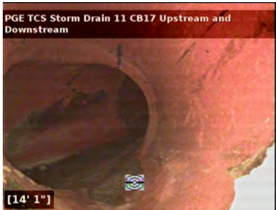
Location where CB17 line discharges into the "main line" of Storm Drain 11, as a "Y".
