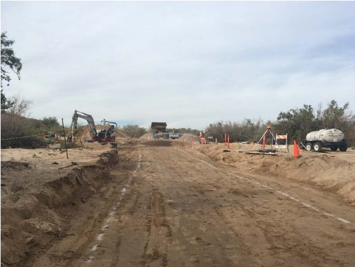
Placement of bedding sand along C5/C7 trench
