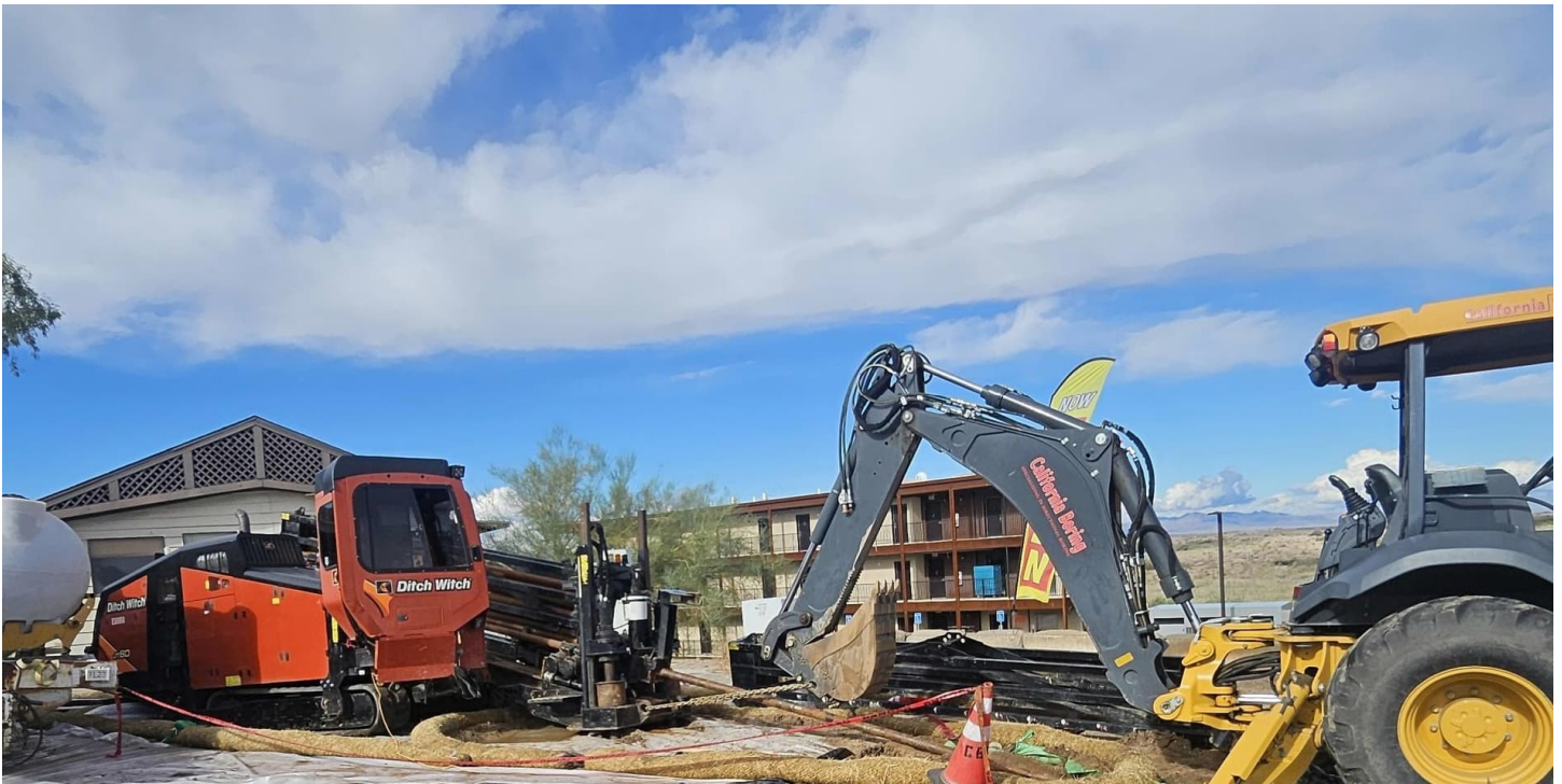
Photo showing drill rig setup at Bore Pit #2 for Pipeline B installation using HDD technology.
