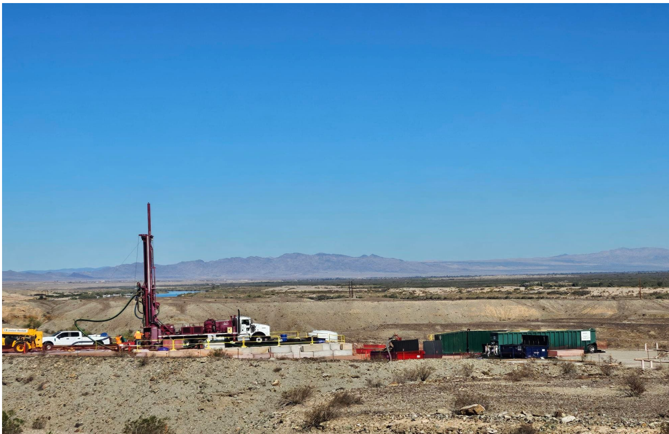
Photo showing dual rotary rig at FW-01.
