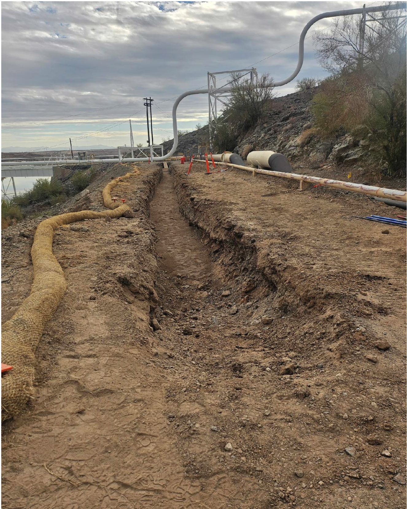
Photo showing trench for installation of Pipeline B in California.
