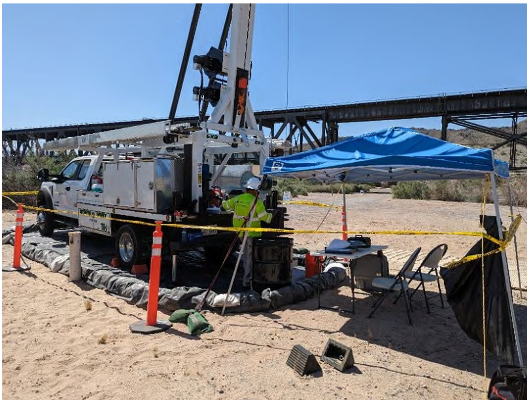
Photo showing well redevelopment at MW-30-30.
