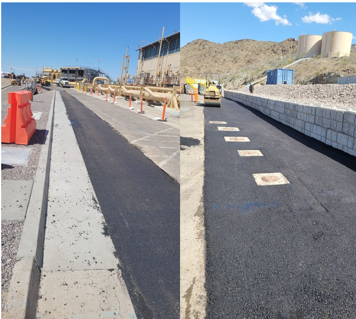
Photos showing asphalt placement atop remedy pipelines inside TCS.
