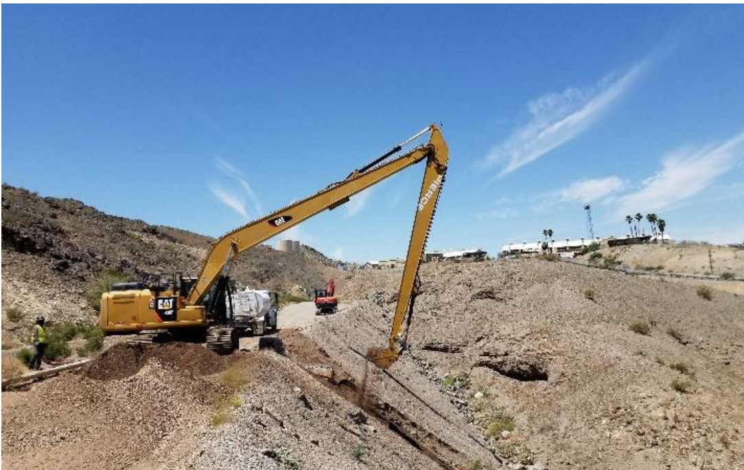
Photo showing repair of stormwater erosion control measures along Pipeline B access road.
