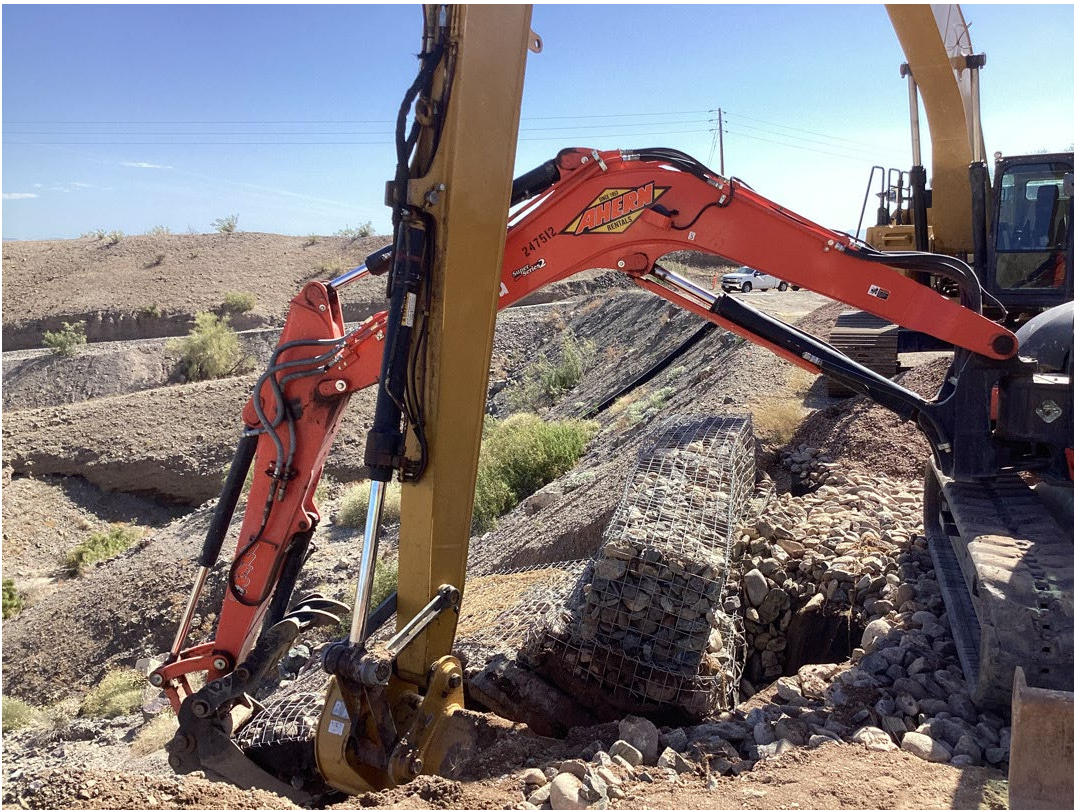
Photo showing the use of excavators to lift and adjust the damaged gabions along Pipeline B access road.
