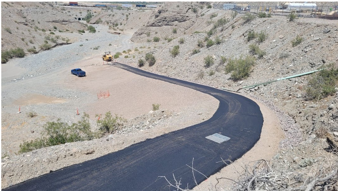
Photo showing asphalt placement on Pipeline I2 access road from TCS to Bat Cave Wash.
