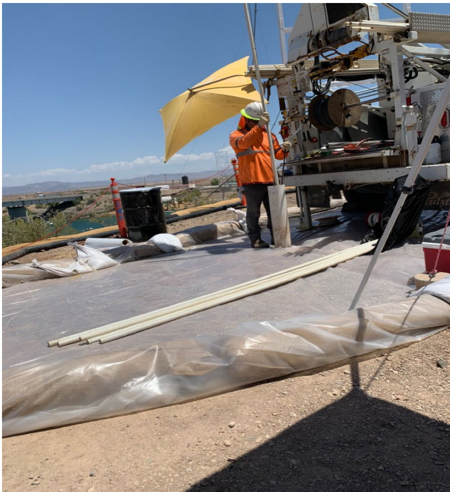
Photo showing installation of downhole equipment at well ER-3.
