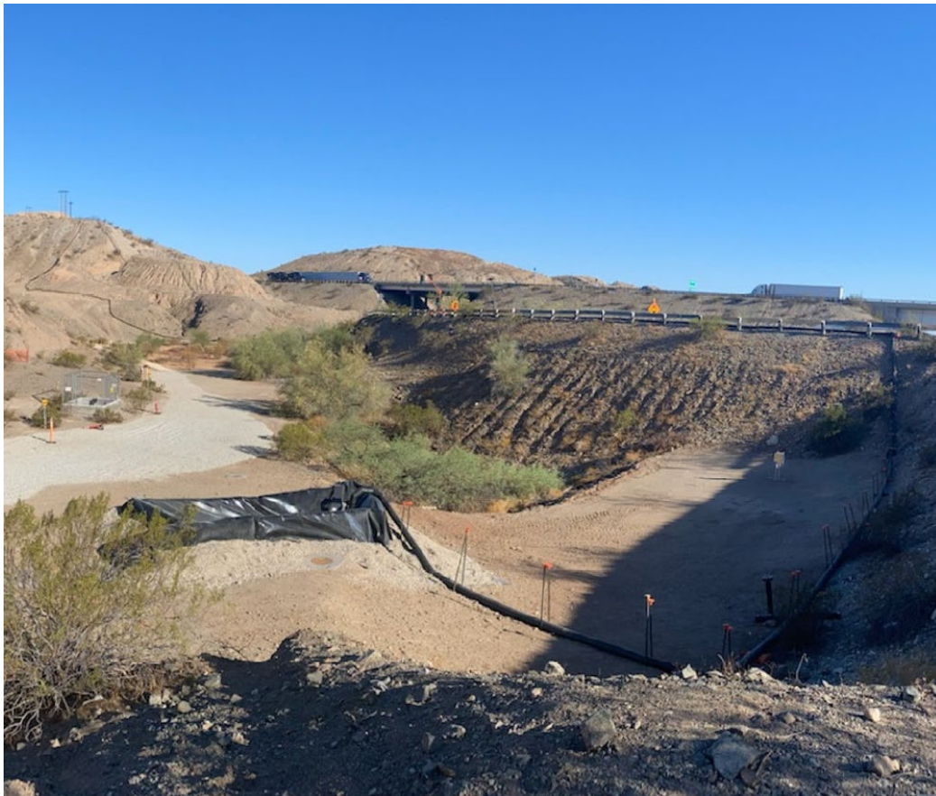
Photo showing temporary TW-01 pipeline from TCS to a connection point prior to the Jack and Bore (foreground). The pipeline will convey extracted water from well TW-1 (located in TCS) to the MW-20 Bench and ultimately to the IM-3 treatment plant.
