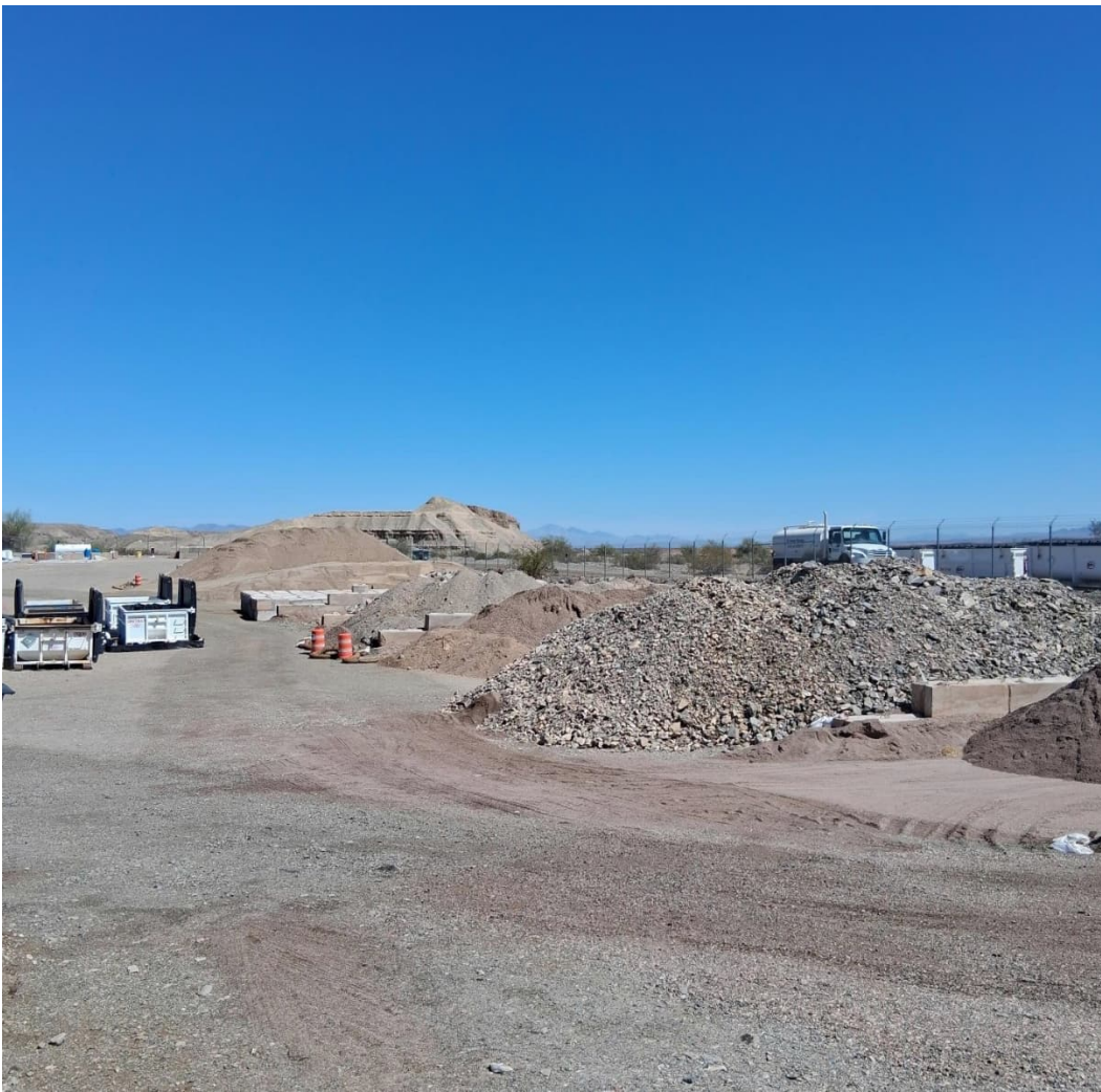
Photo showing the Soil Processing Yard.
