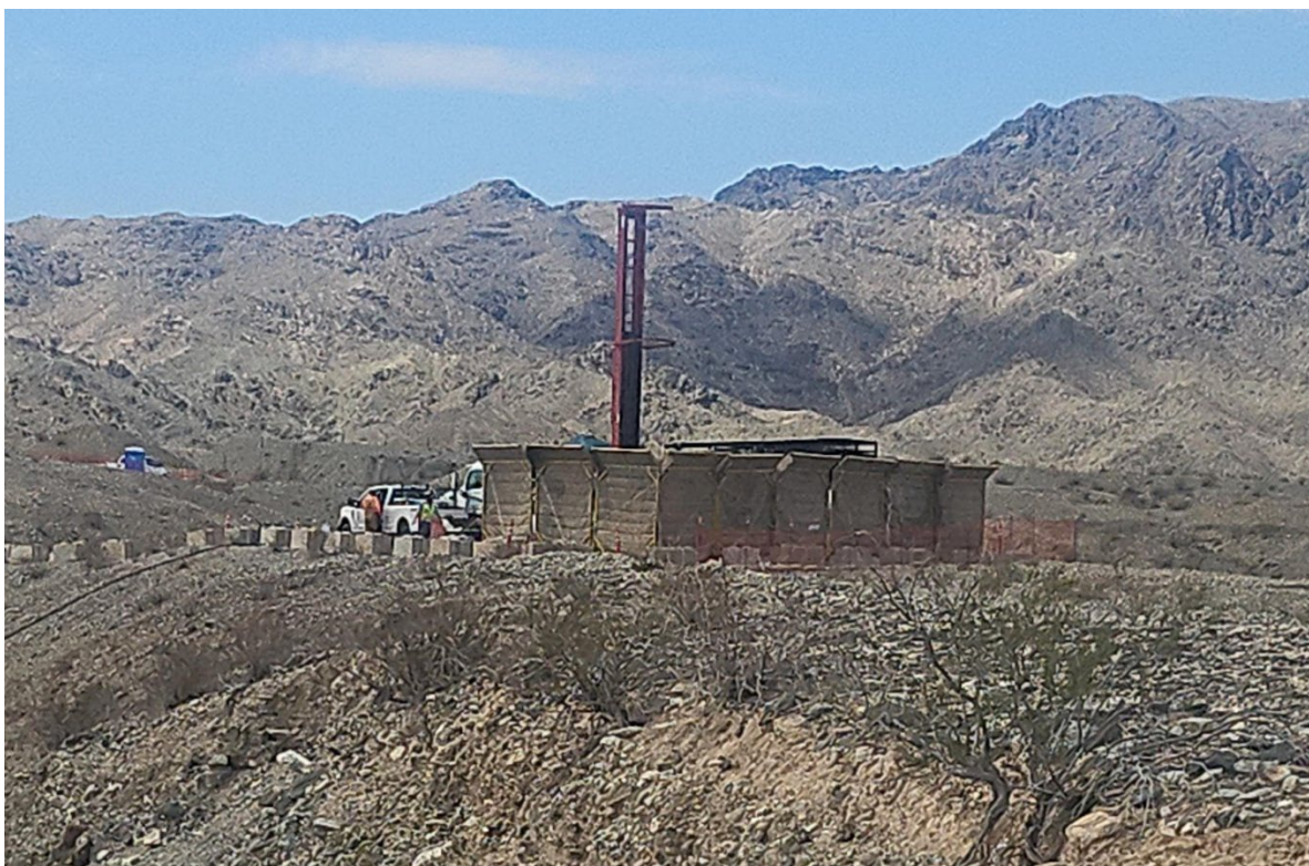
Photo showing sonic rig at MW-100D with sound barrier in the foreground.
