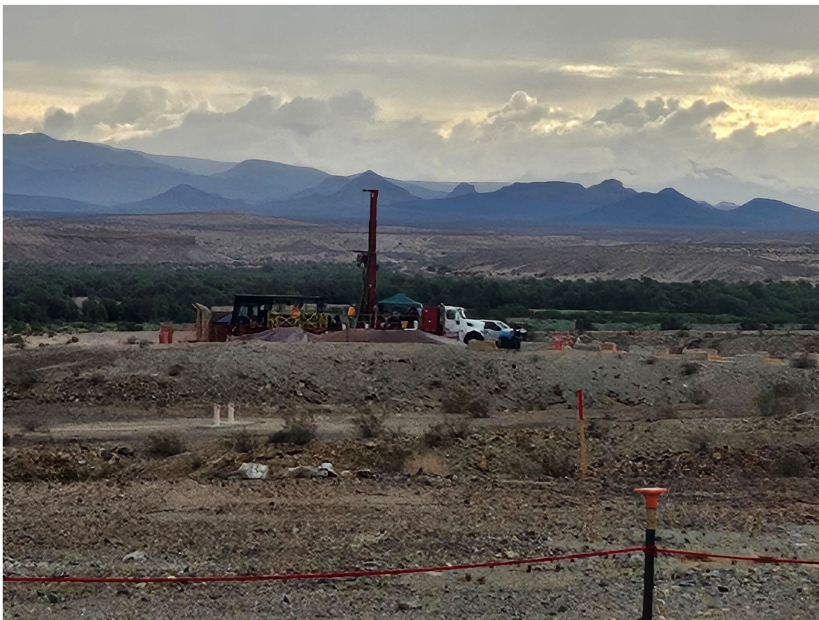
Photo showing sonic rig at MW-100D.
