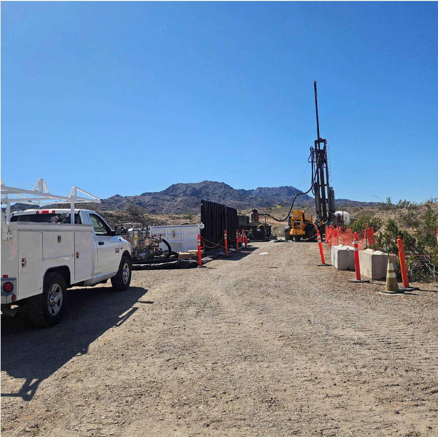
Photo showing drill rig setup at IRL-03.
