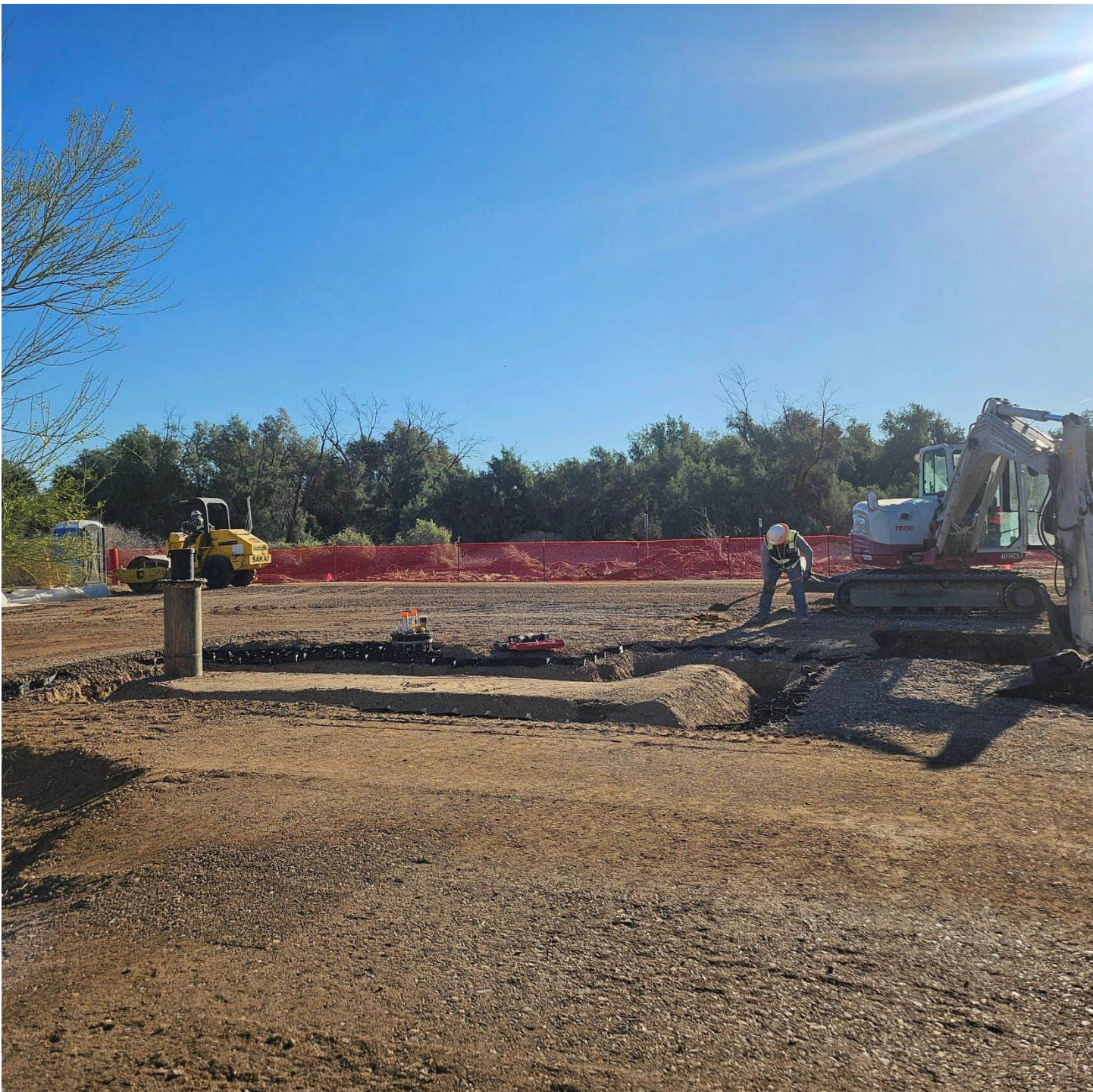
Photo showing excavation of HNWR-1A concrete pad
