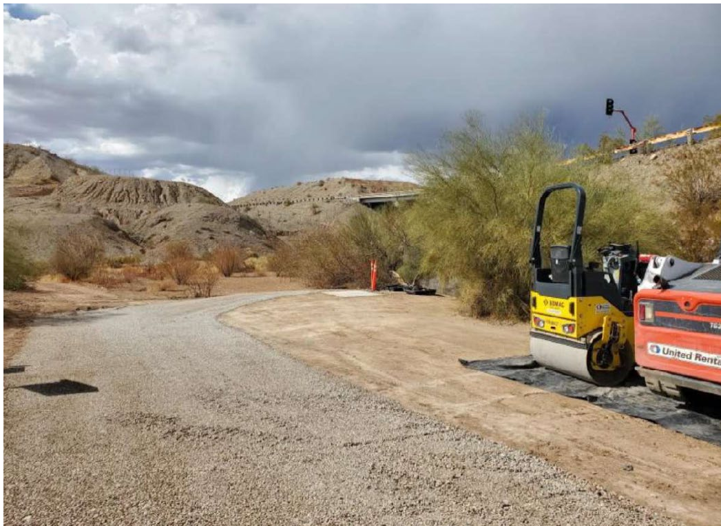
Photo showing earthfill and crushed rock installed at IRZ-39.
