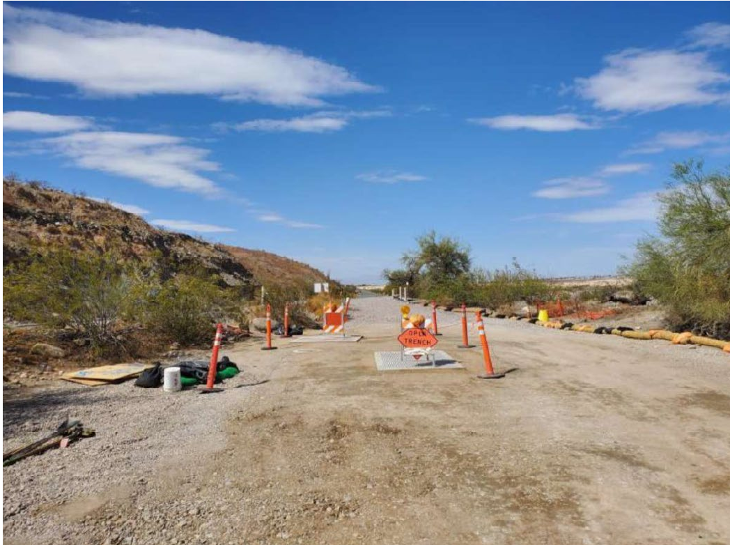
Photo showing lid and earthfill installation at IRZ-18.
