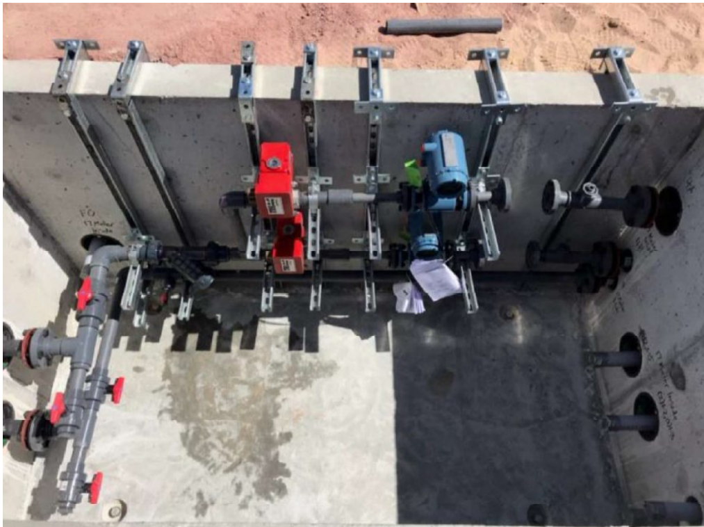
Photo showing prefabrication of IRZ dual screen cluster injection meter vault at IRZ-17.
