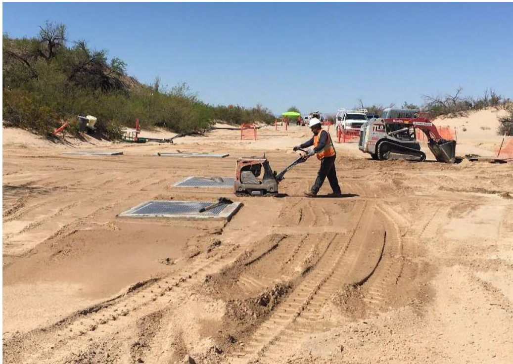
Photo showing backfill and compaction at IRZ-11.
