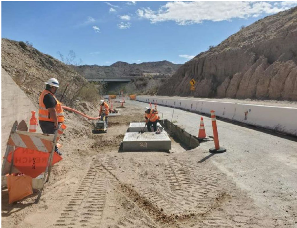
Photo showing lids and earthfill installation at IRZ-29.
