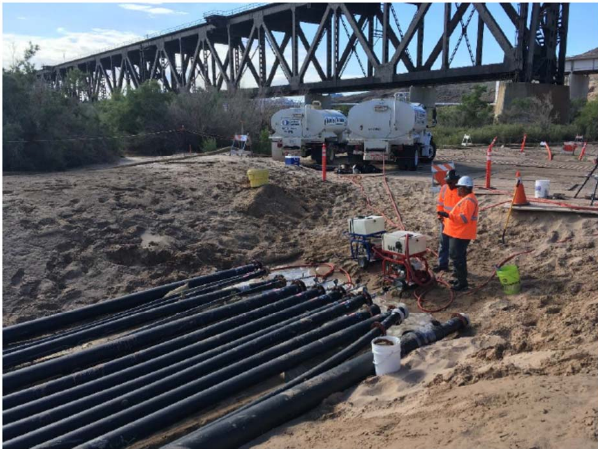
Filling and leak testing of HDPE pipelines at C5 pipeline end.
