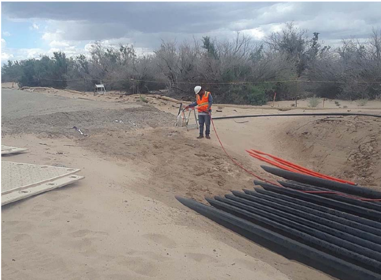
Freshwater used for hydrostatic testing discharged to ground, inside pipe trench, through a sock.
