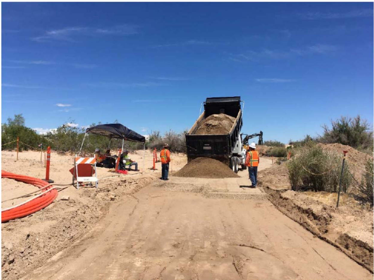
Delivery of aggregate base from SPY for IRZ access road installation north of Pipeline C3.
