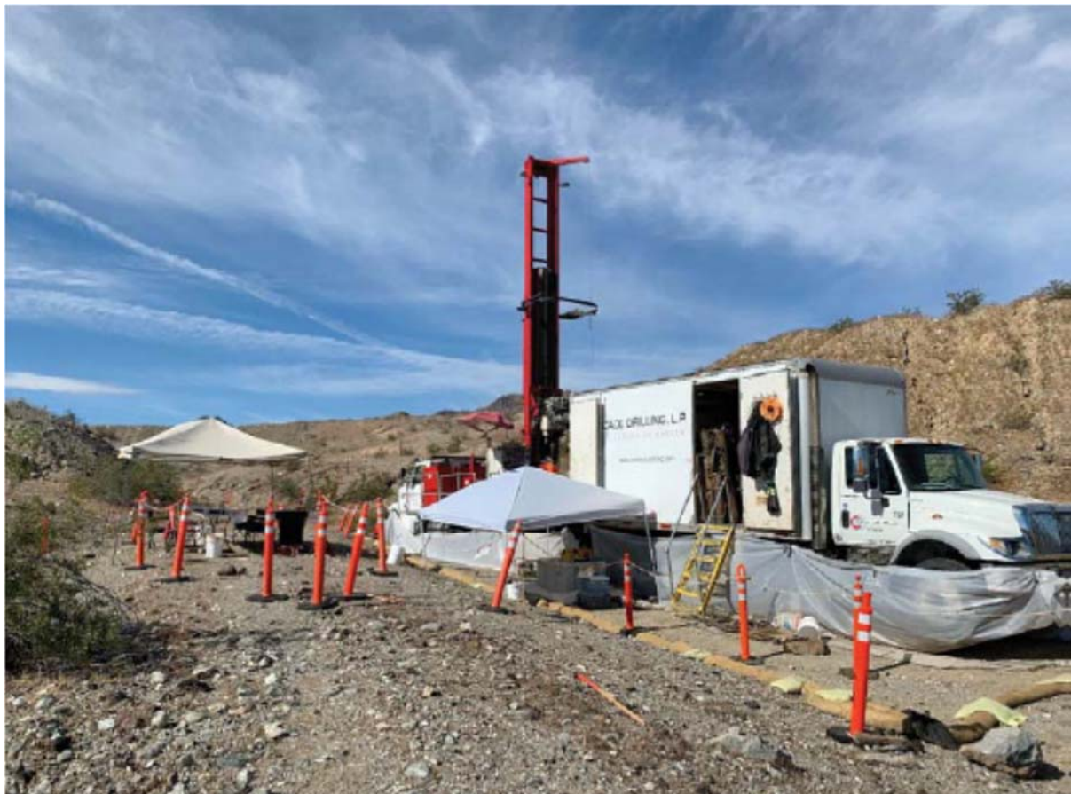
MW-R Well Installation.
