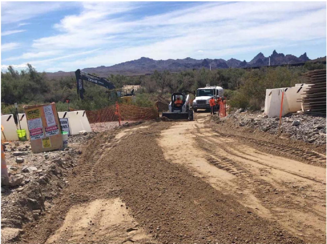
Placement of aggregate base along IRZ access road north of Pipeline C3
