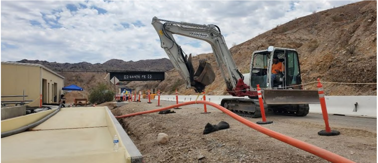
Photo showing crew moving pipe to allow backfill alongside of unloading pad.
