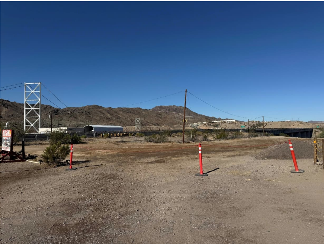
Photo showing the restored Staging Area 26 after completion of Pipeline B installation in Arizona.
