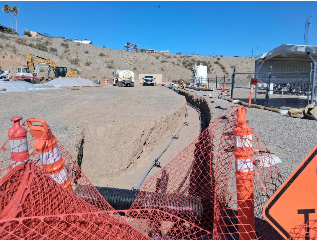
Photo showing the relocated Pipeline E alignment at the Transwestern Bench.
