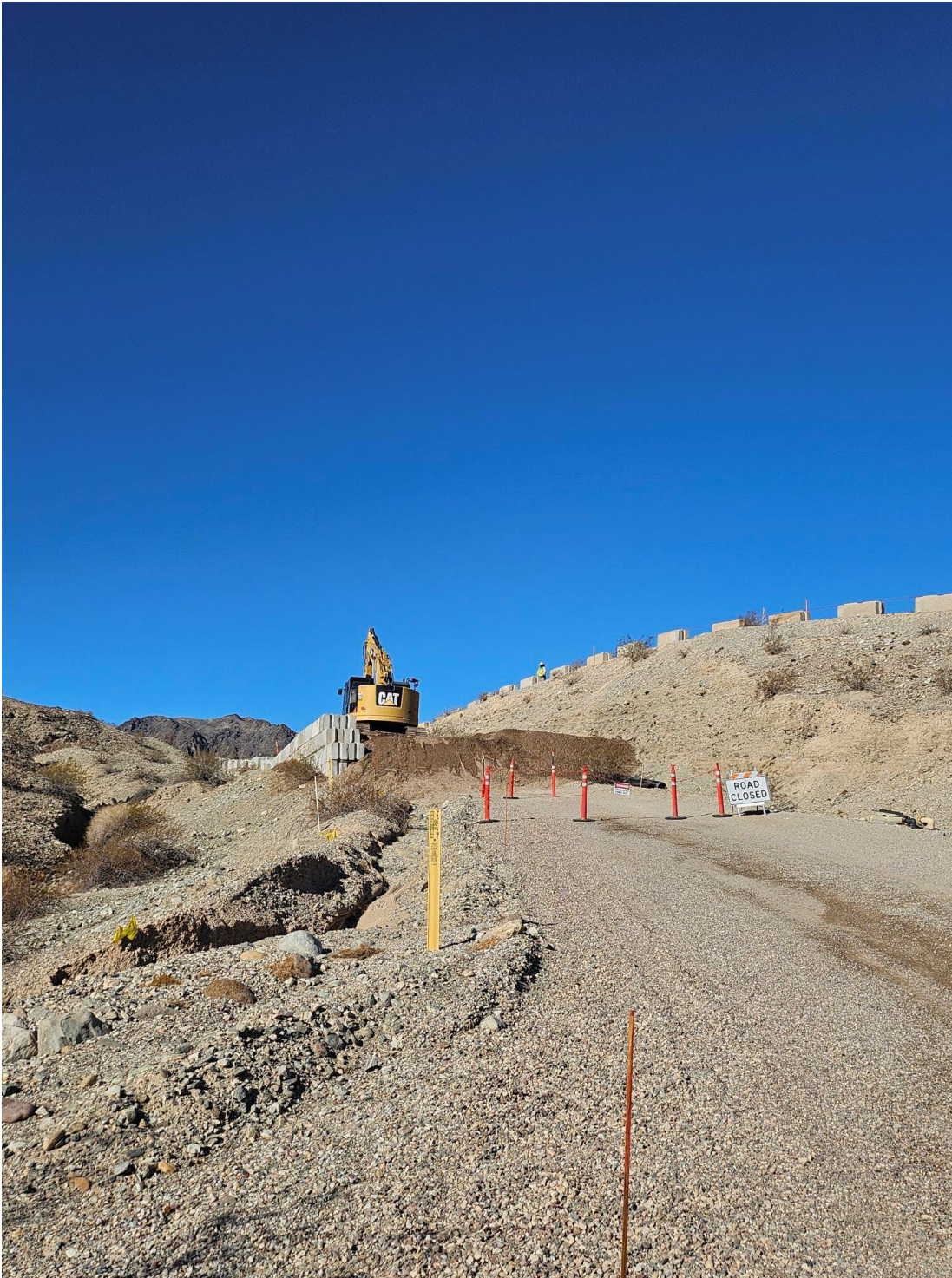
Photo showing construction of the drill pad for MW-103 (former MW-BB) on IM3 access road.
