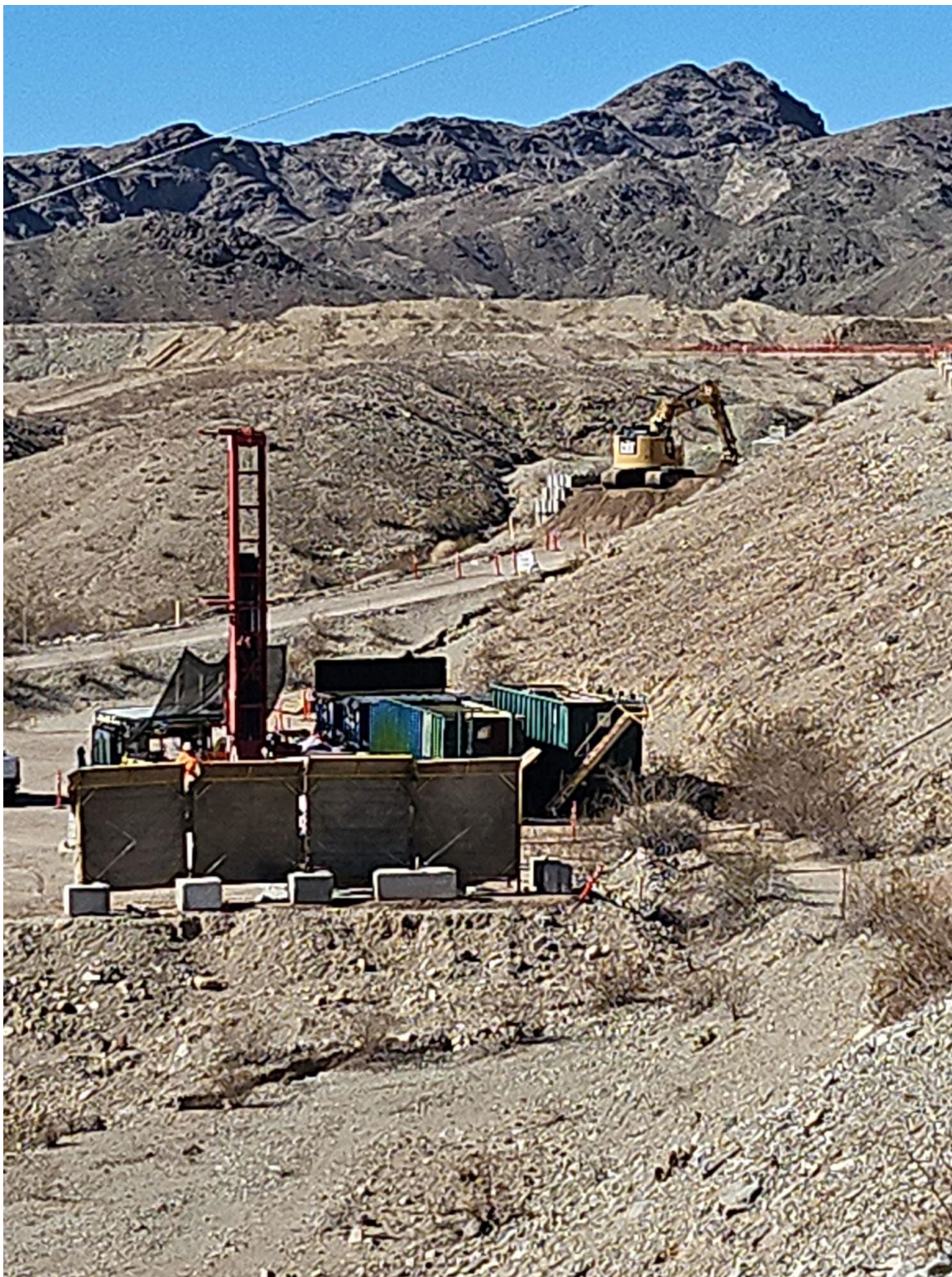
Photo showing drilling at MW-102 (former MW-AA) in the foreground and construction of MW-103 (former MW-BB) drill pad in the background.
