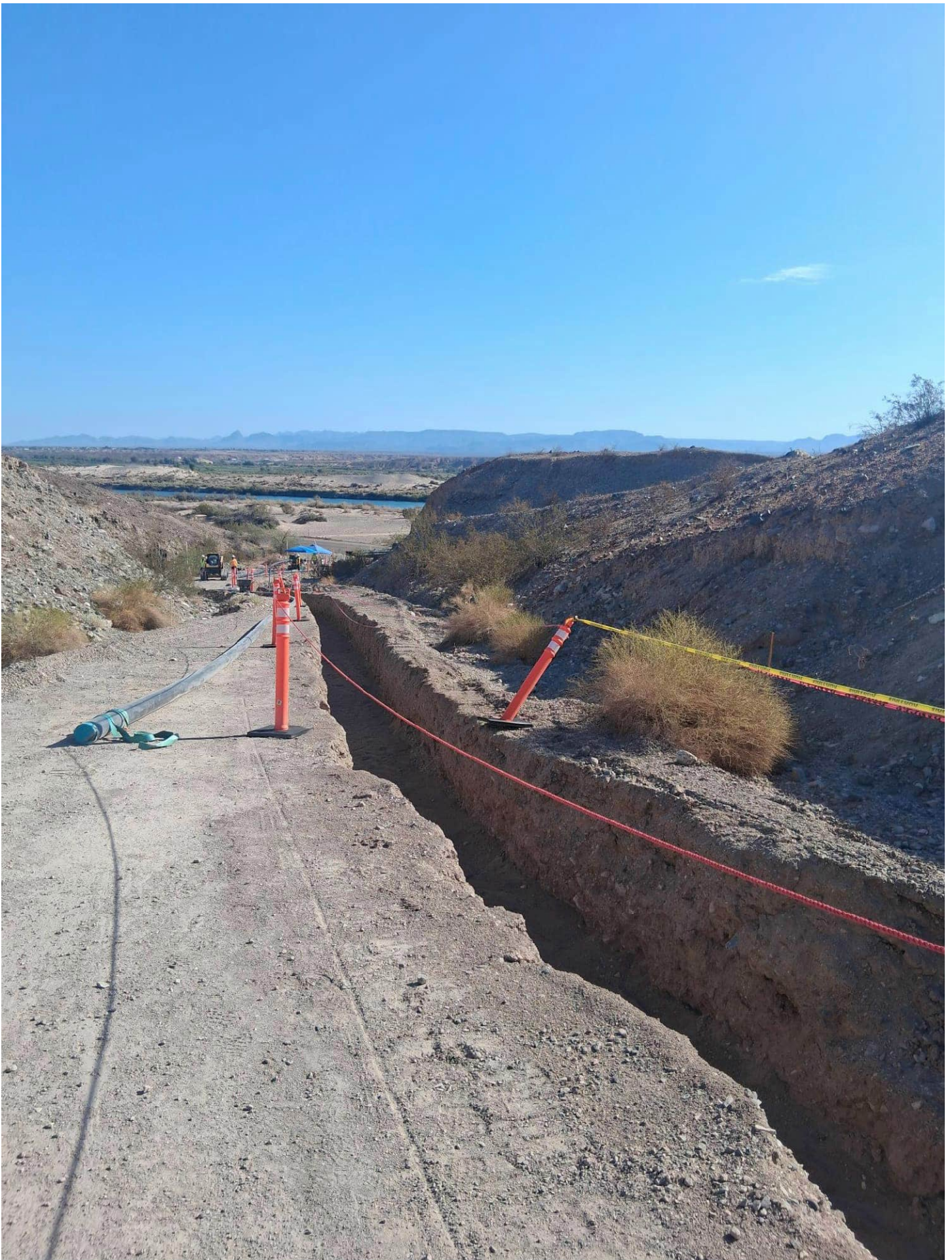
Photo showing Pipeline A near Station 44+80 towards National Trails Highway.
