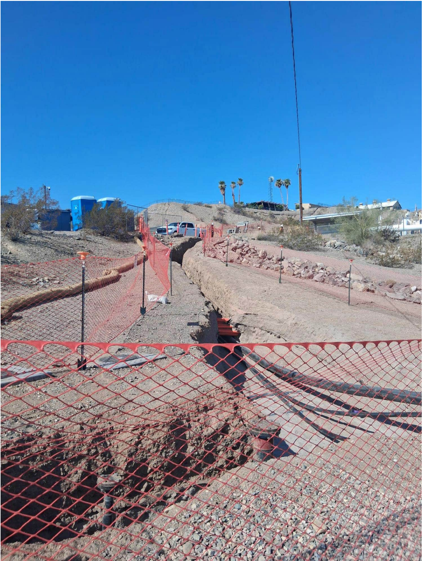
Photo showing the relocated Pipeline E from the Transwestern Bench to Pipeline F/J junction.
