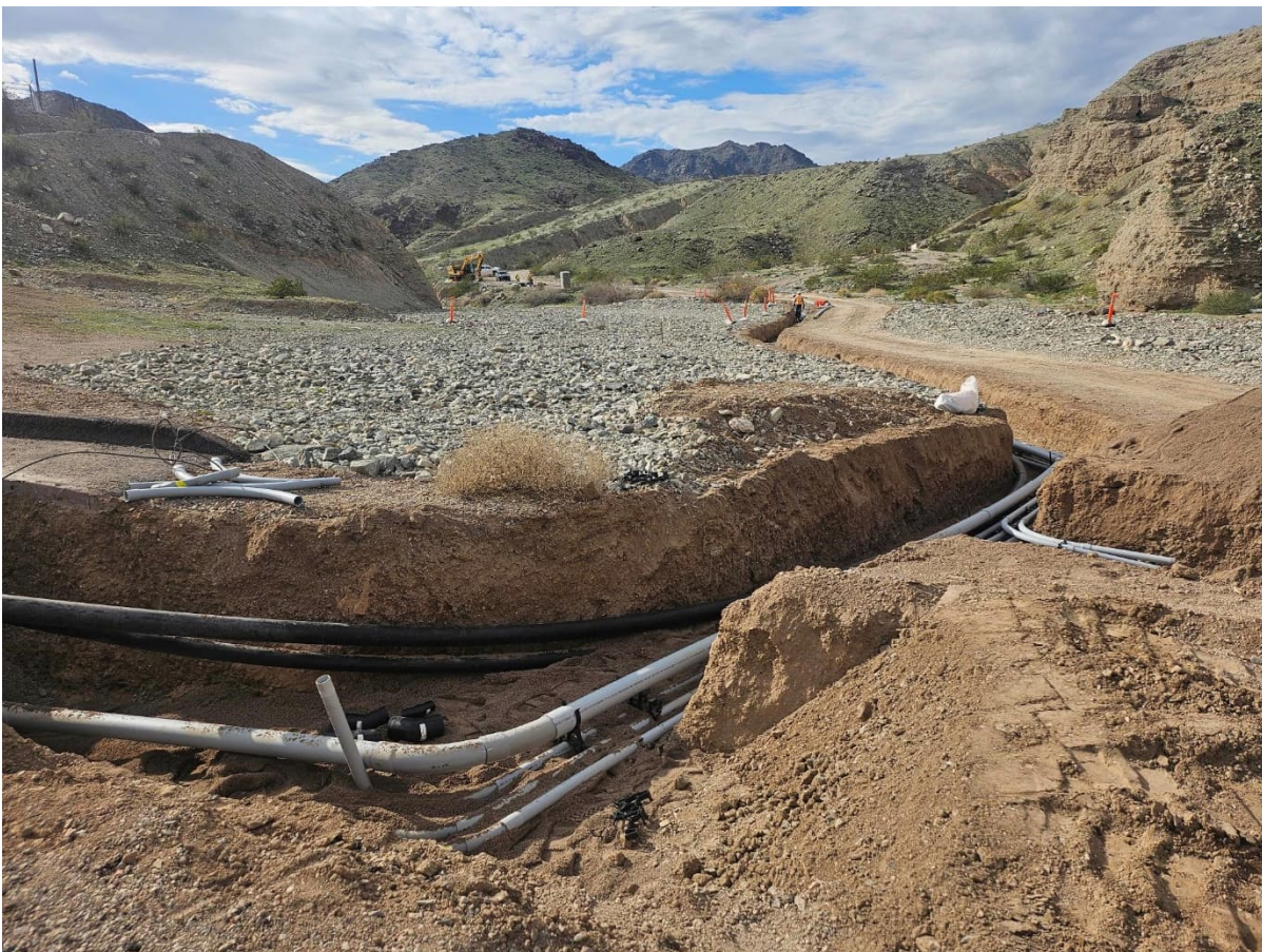
Photo showing pipes and conduits in trench (Pipeline I2).
