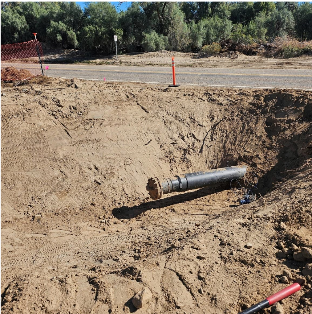
Photo showing the 12-inch water line in the HDD bore pit.
