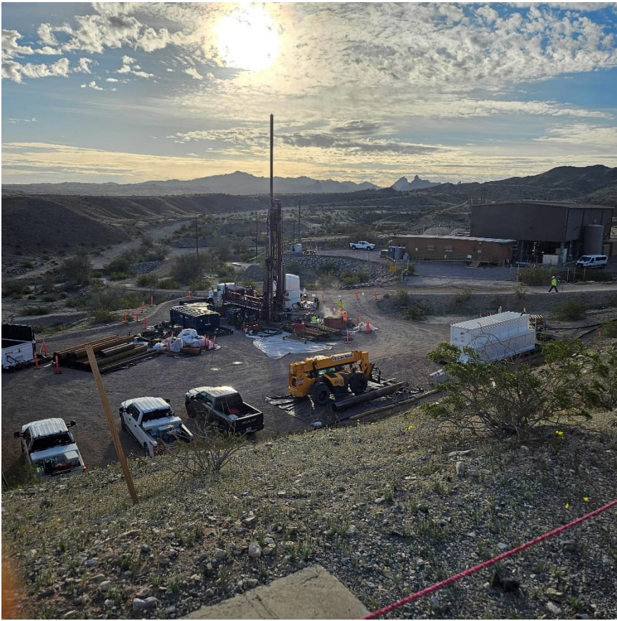
Photo showing drill rig setup at IRL-01.
