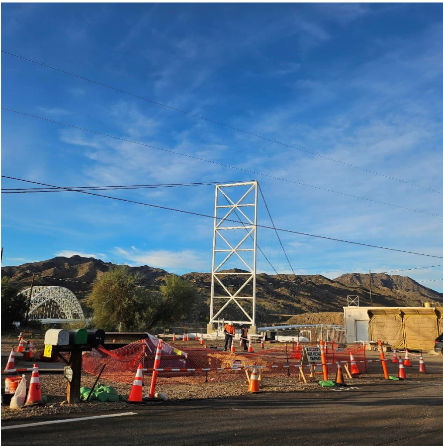
Photo showing Jack and Bore entrance pit work area.
