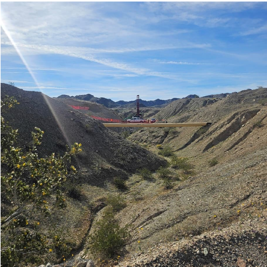
Photo showing drill rig setup at MW-109 (former MW-Q).
