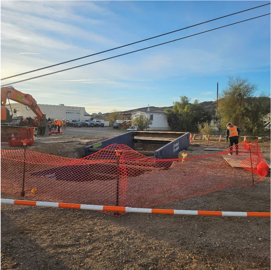
Photo showing a shoring box being placed in the entrance pit.
