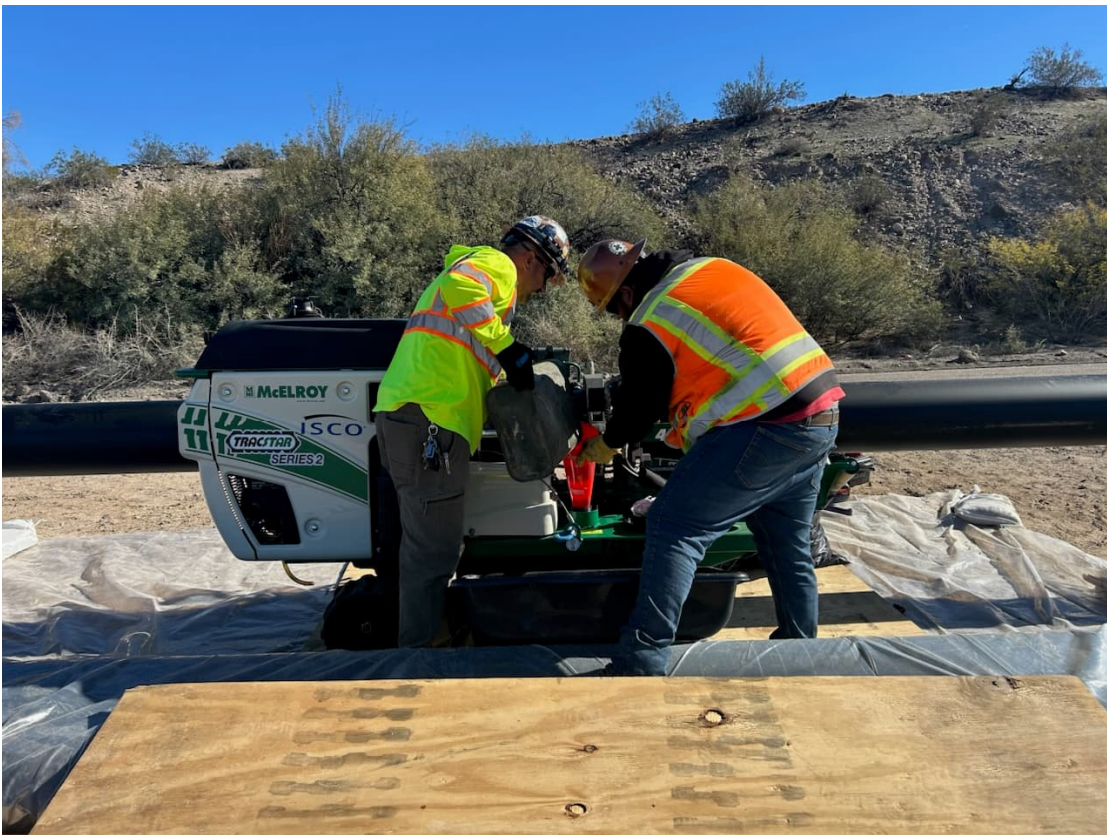
Photo showing refueling of HDPE fusing machine at Bore Pit #5 for Pipeline B installation in Arizona.
