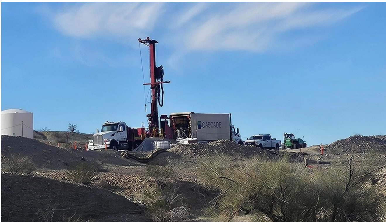
Photo showing sonic drilling at MW-J.
