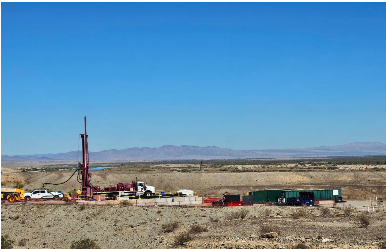
Photo showing dual rotary rig at FW-01.
