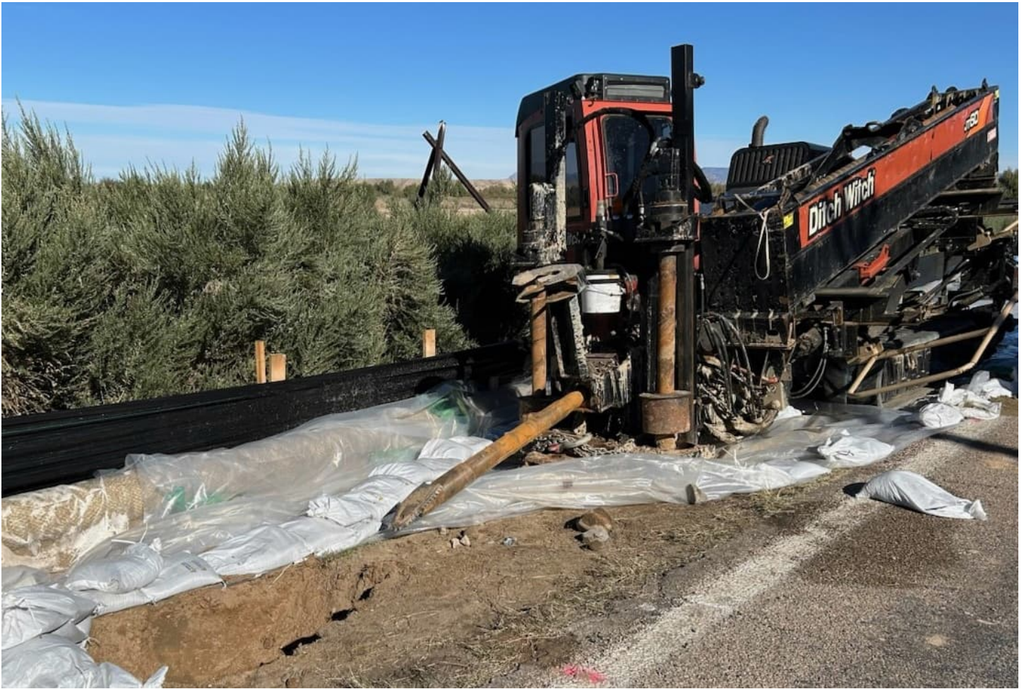
Photo showing drill rig setup at Bore Pit #4 for Pipeline B installation using Horizontal Directional Drilling (HDD).
