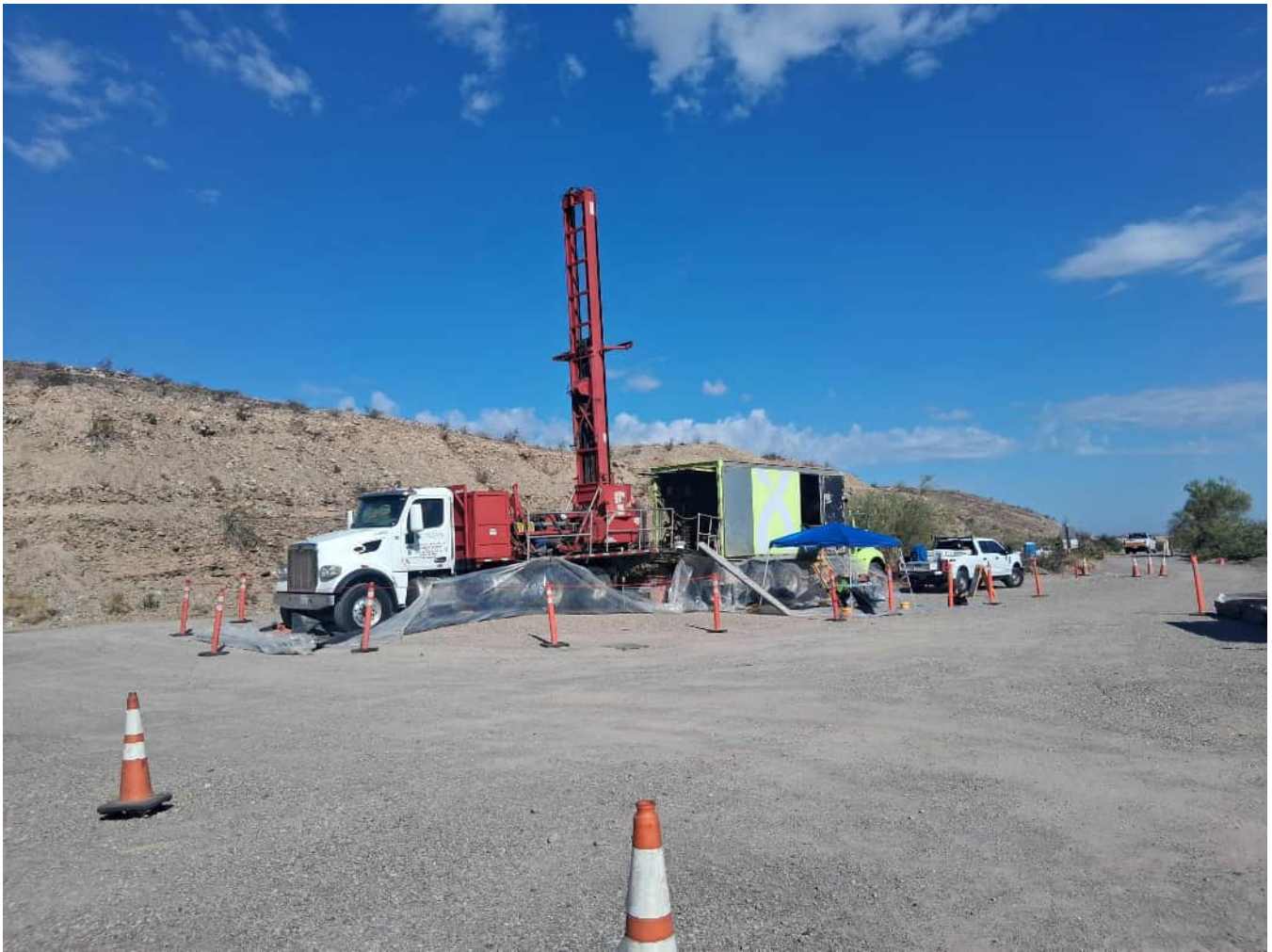
Photo showing drilling of the pilot borehole for IRZ-20 mid-depth well on the MW-20 Bench. Photo taken on September 2, 2026.
