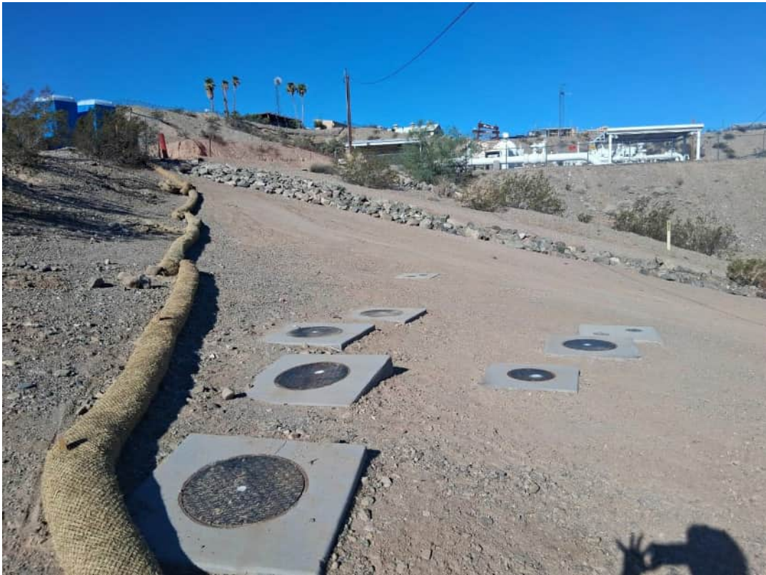
Photo showing the completed Pipeline E from the Transwestern Bench to Pipeline F/J junction. Photo taken on September 2, 2026.
