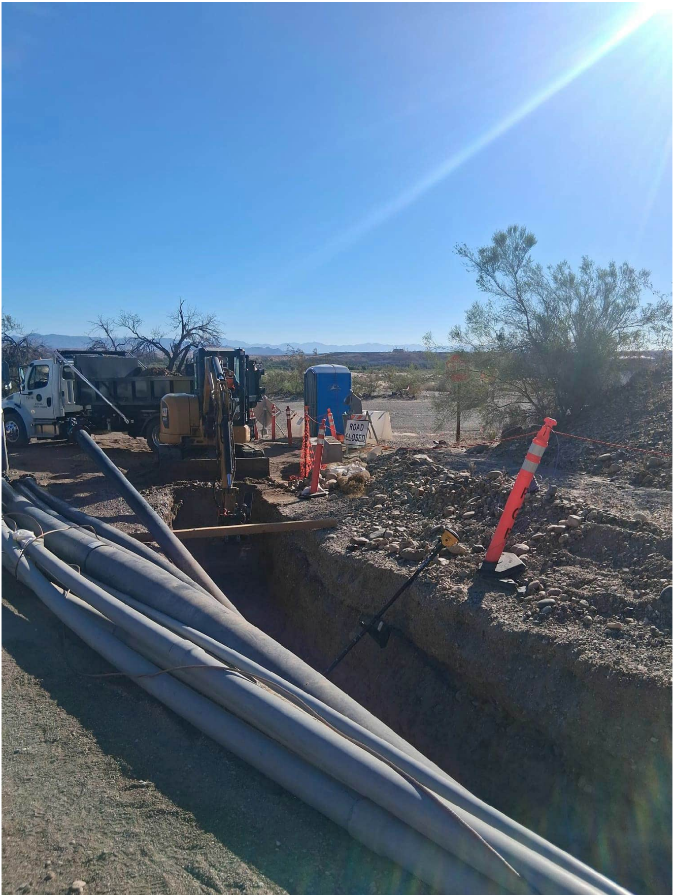
Photo showing preparation to flush and hydrostatic test Pipeline A near National Trails Highway. Photo taken on September 2, 2026.
