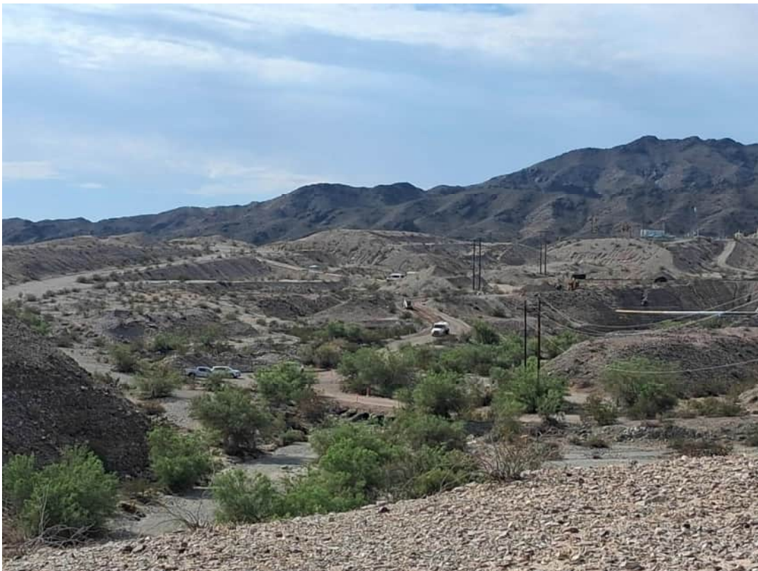
Photo showing repair of a portion of IM3 access road affected by the August 2026 storm event. Photo taken on September 2, 2026.
