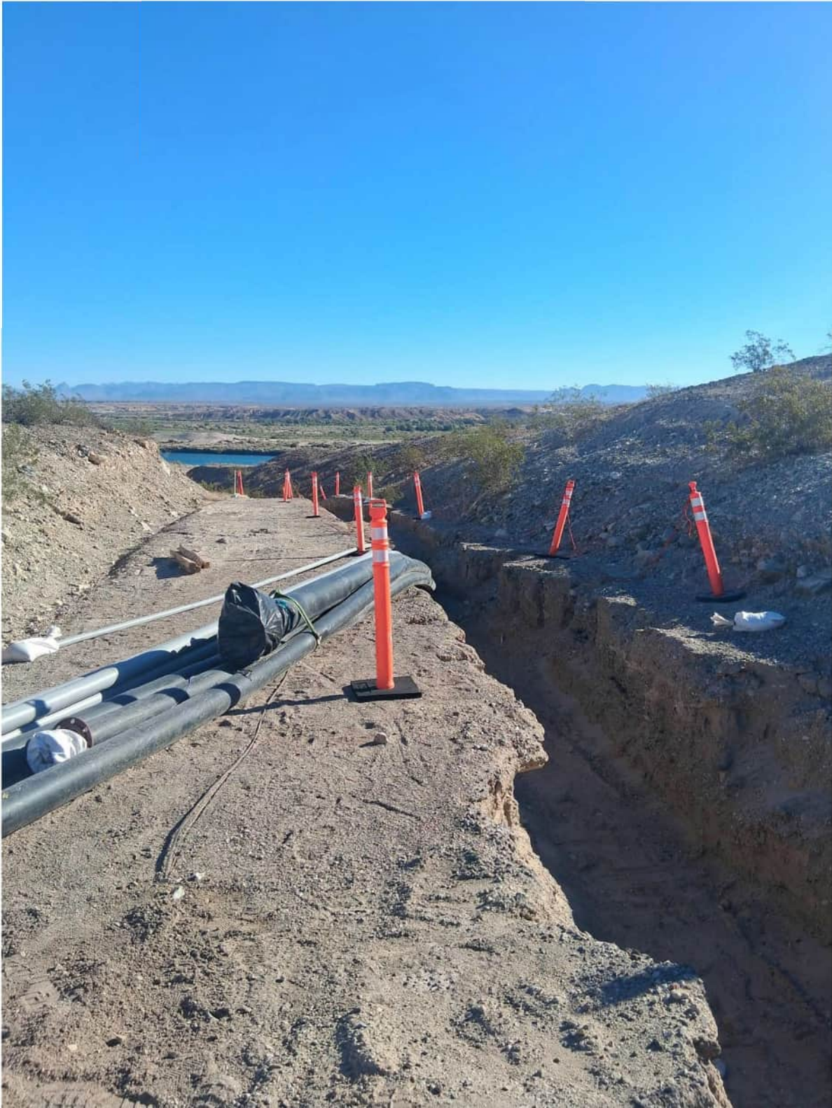
Photo showing preparation to flush and hydrostatic test Pipeline A near Station 44+75. Photo taken on September 2, 2026.
