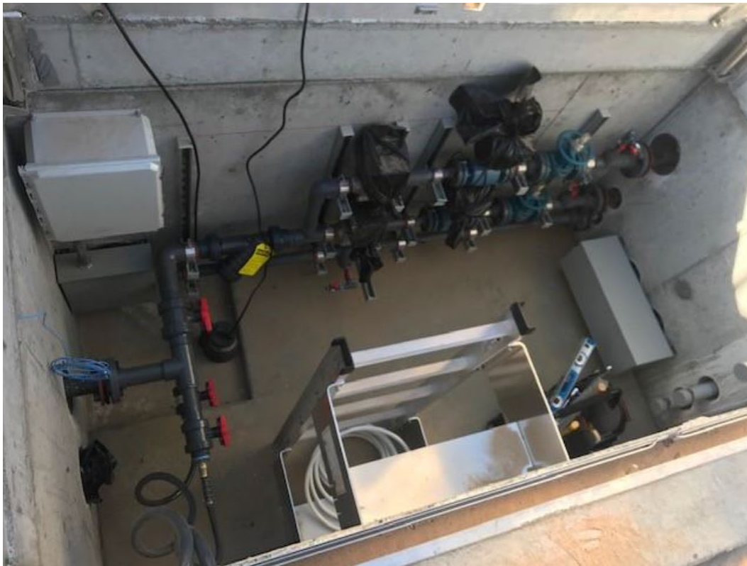
Hydrostatic leak test setup at IRZ-15 meter vault.
