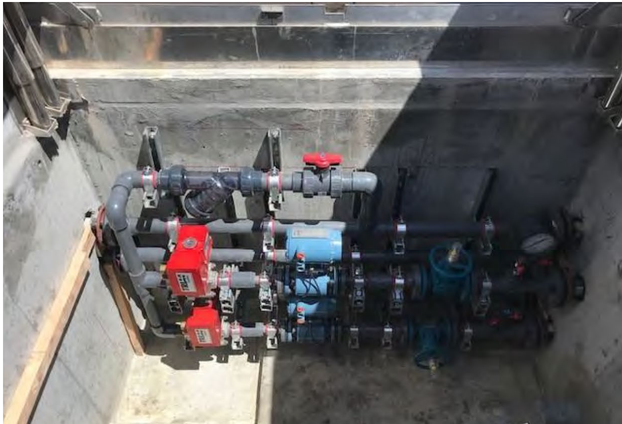
Completed installation of mechanical components at IRZ-33 meter vault.
