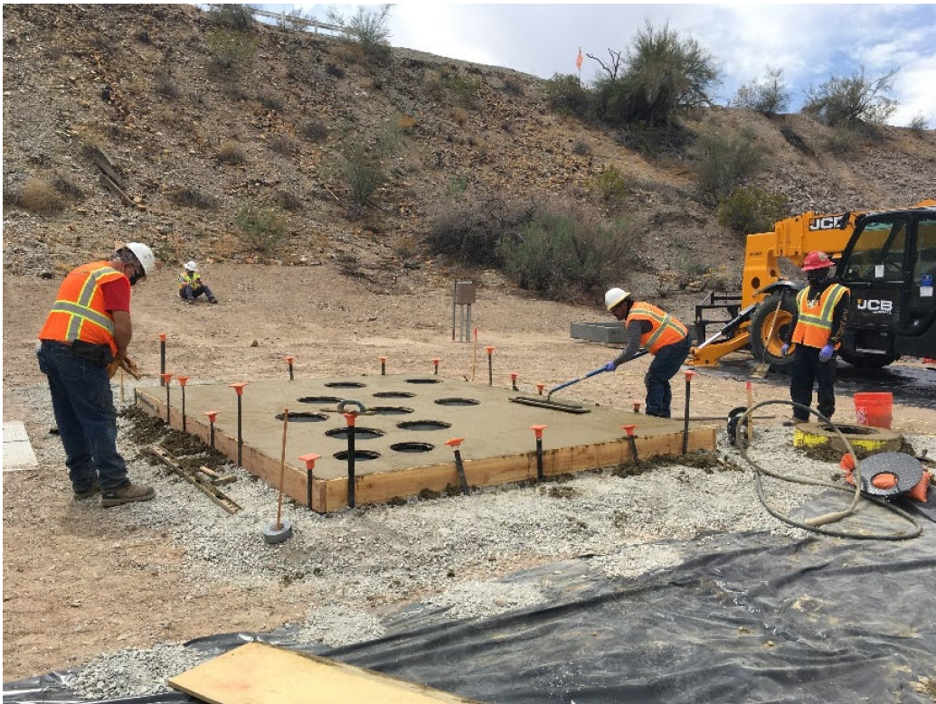
Photo showing concrete pad installation at C8alt/C9 cleanouts.
