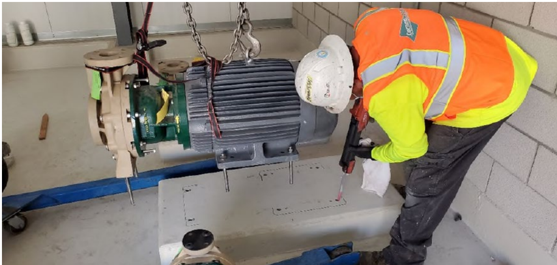
Photo showing a worker applying epoxy to set anchor bolts in place inside the Carbon Amendment Building.
