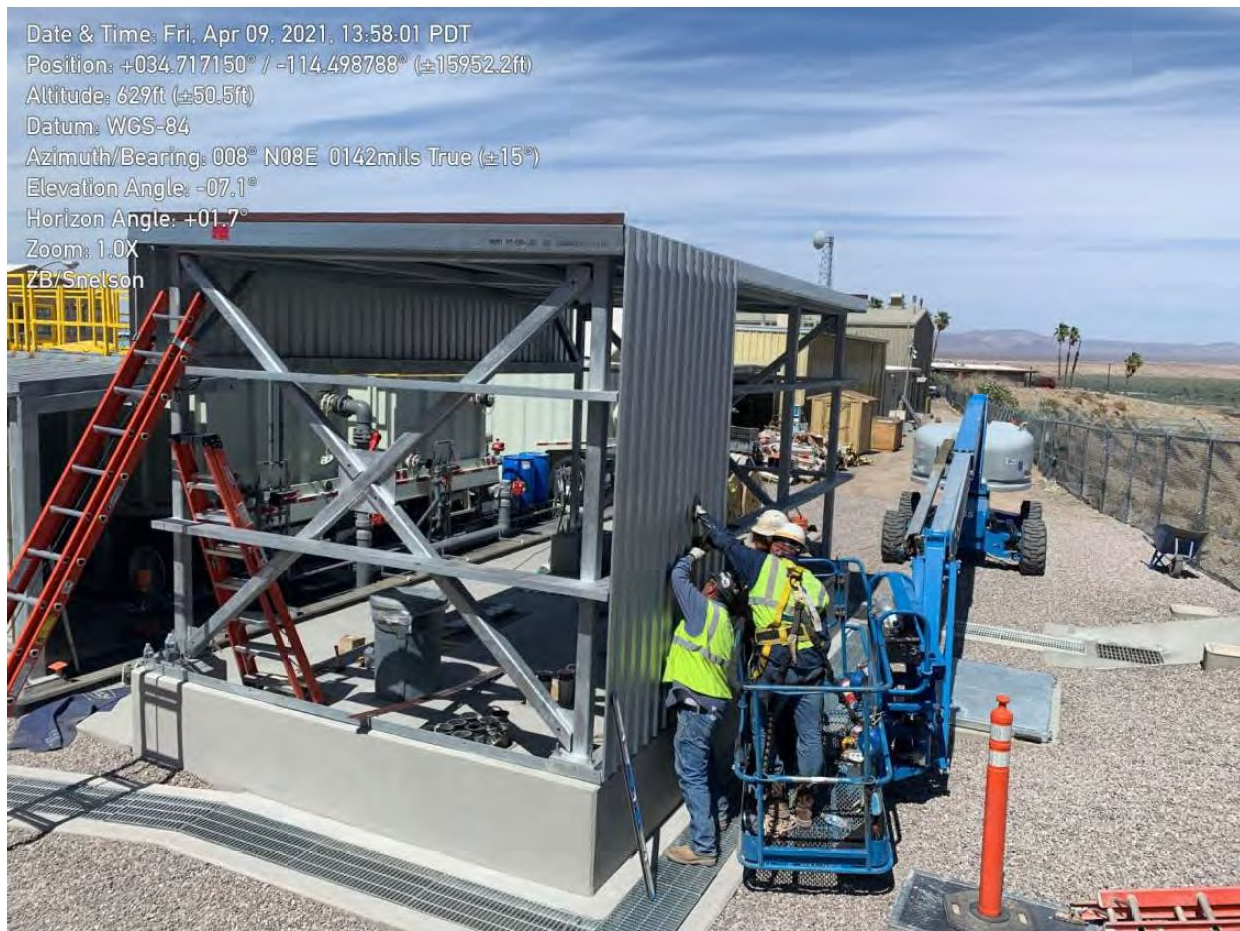
Photo showing installation of the canopy for the switch gear.
