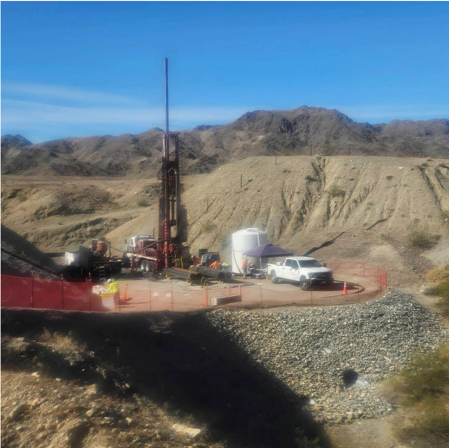
Photo showing drill rig at IRL-04.
