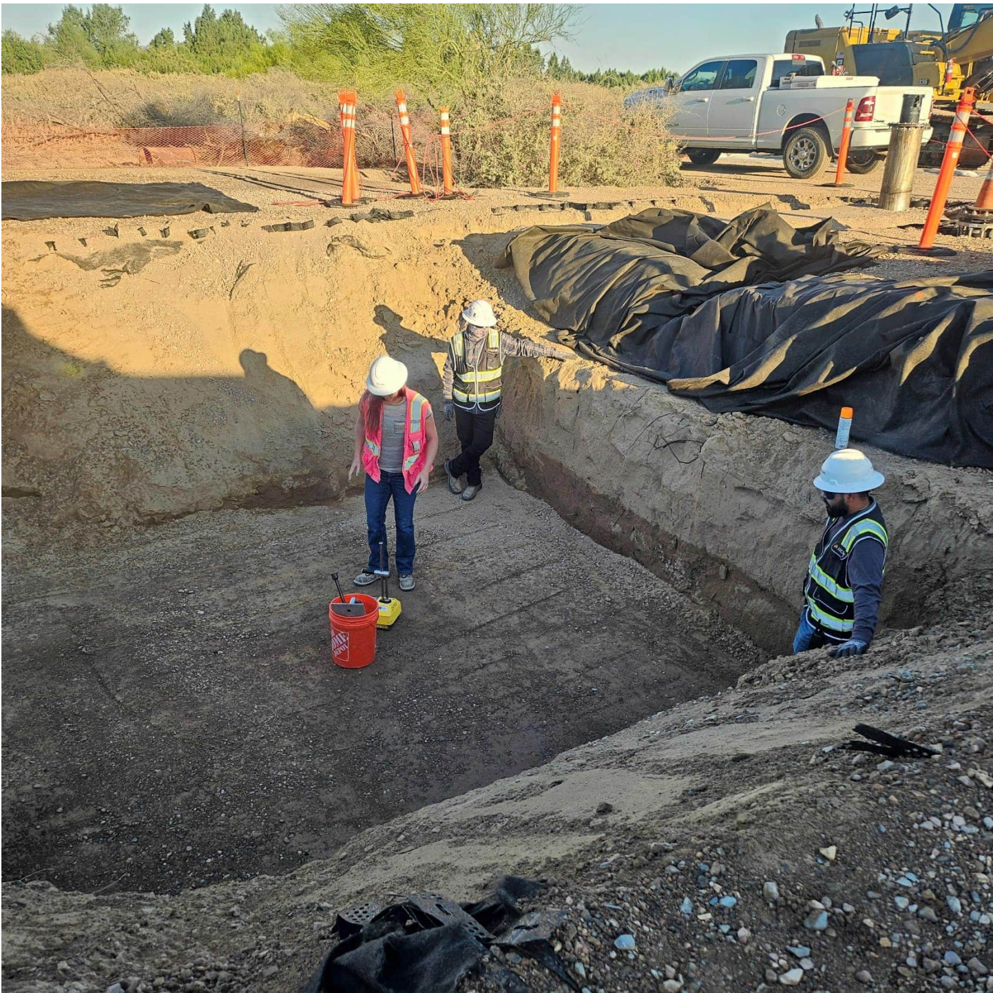
Photo showing geotechnical testing at HNWR-1A pad
