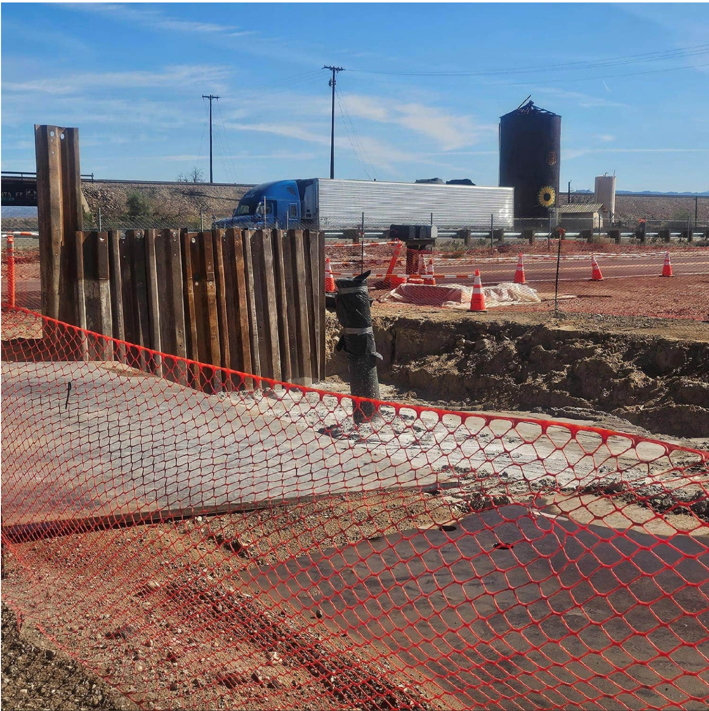
Photo showing the I-40 Jack and Bore entrance pit with CLSM.
