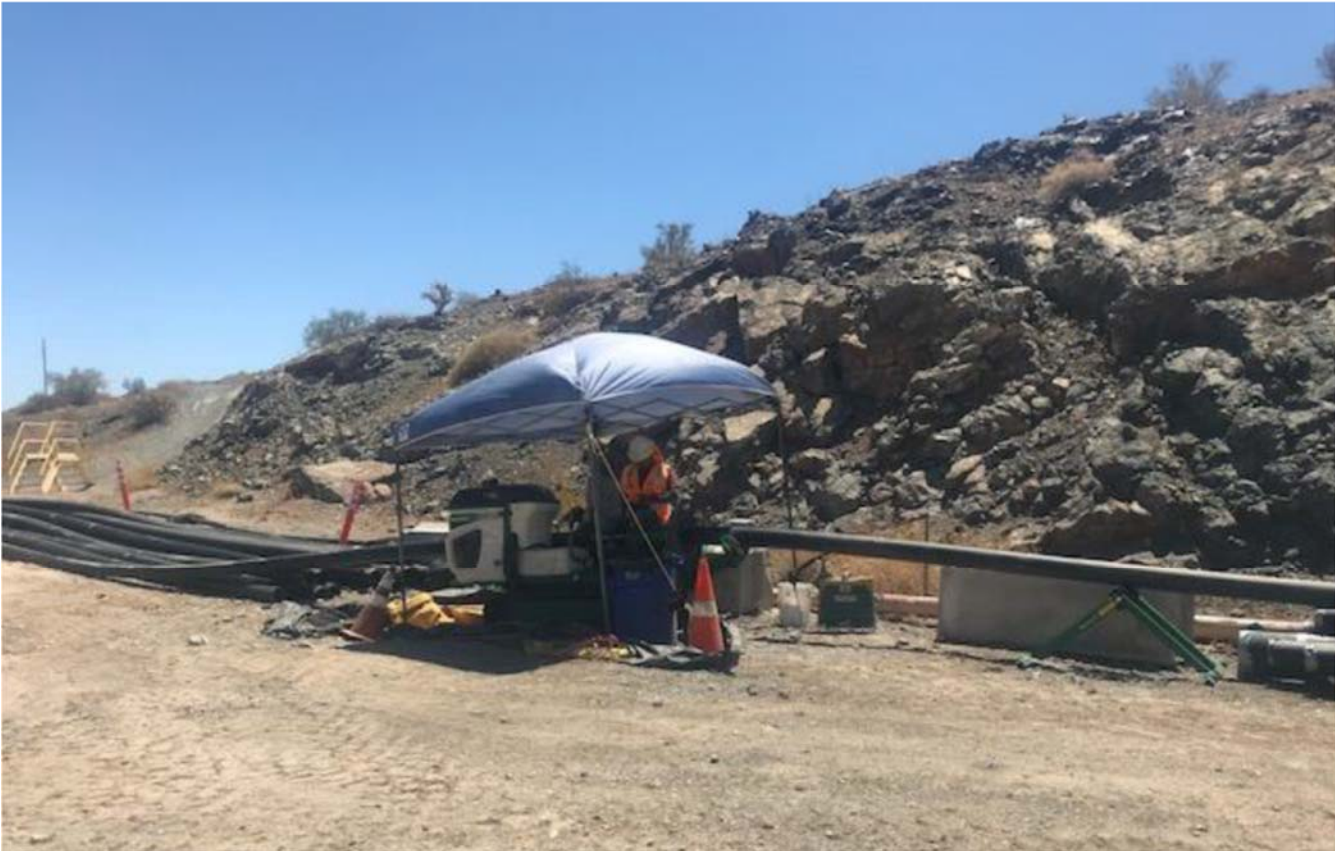
HDPE Pipe Fusing at Pipeline B Work Area
