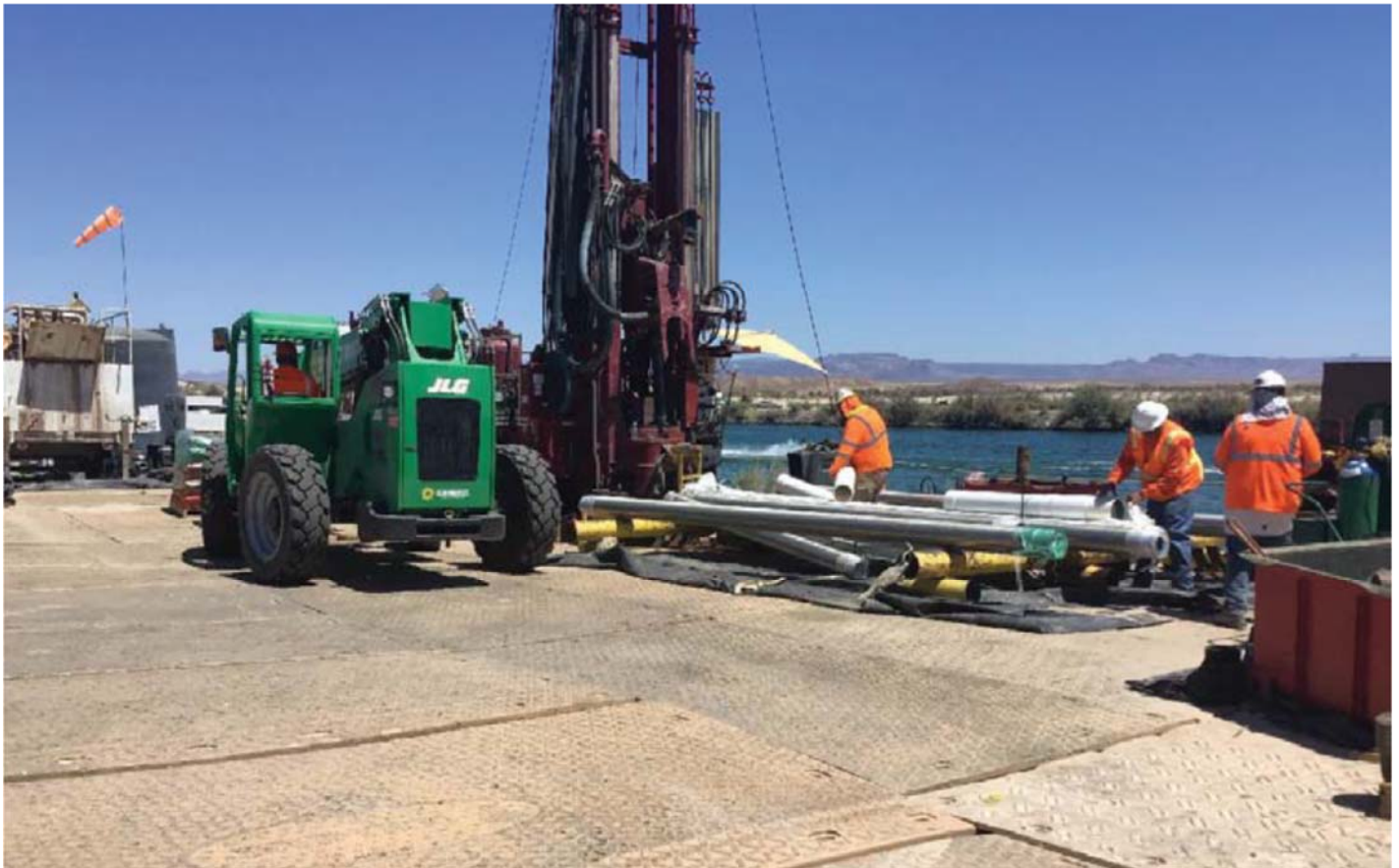
Remedy Well Installation at RB-4
