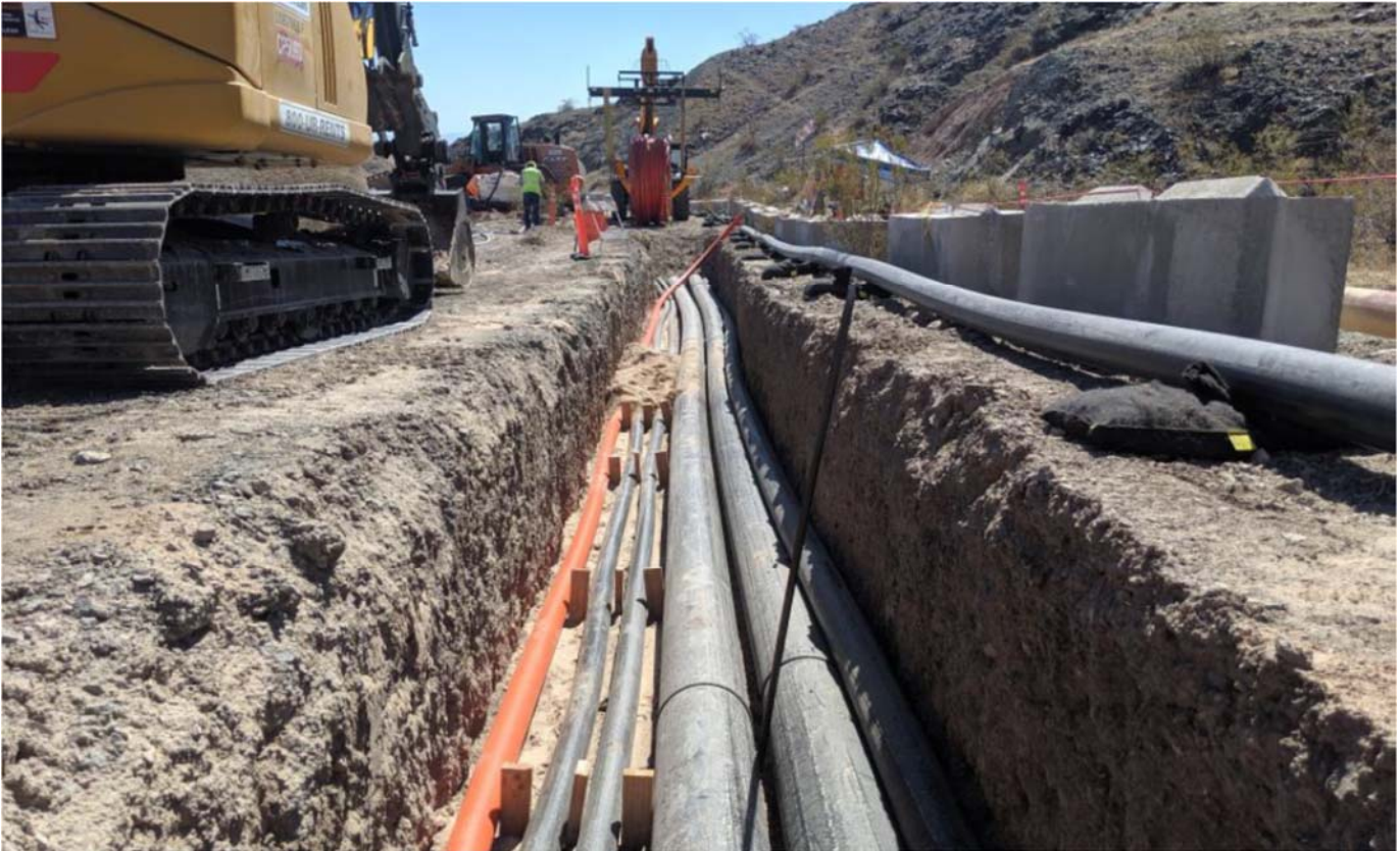
Installed HDPE piping within Pipeline B Trench
