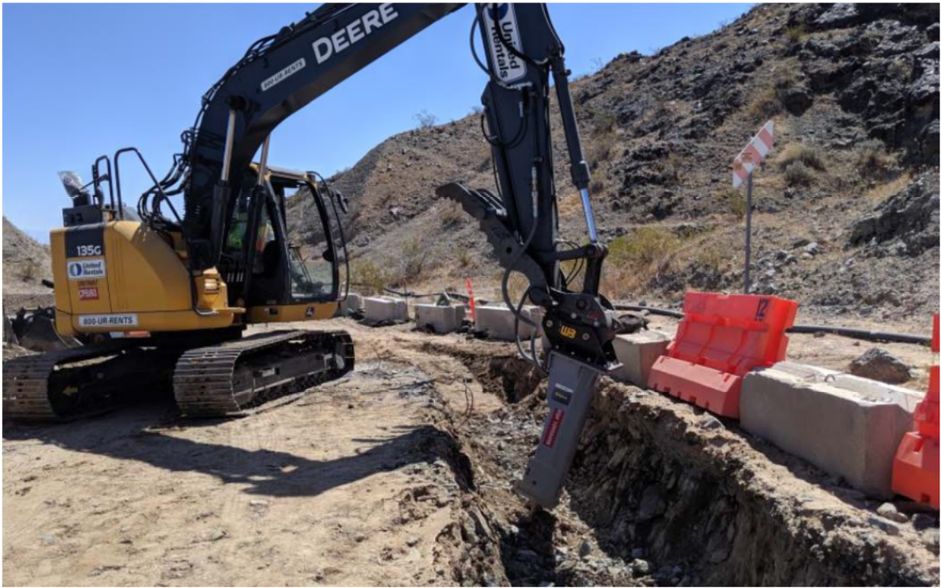
Breaking Dense Rock at Pipeline B
