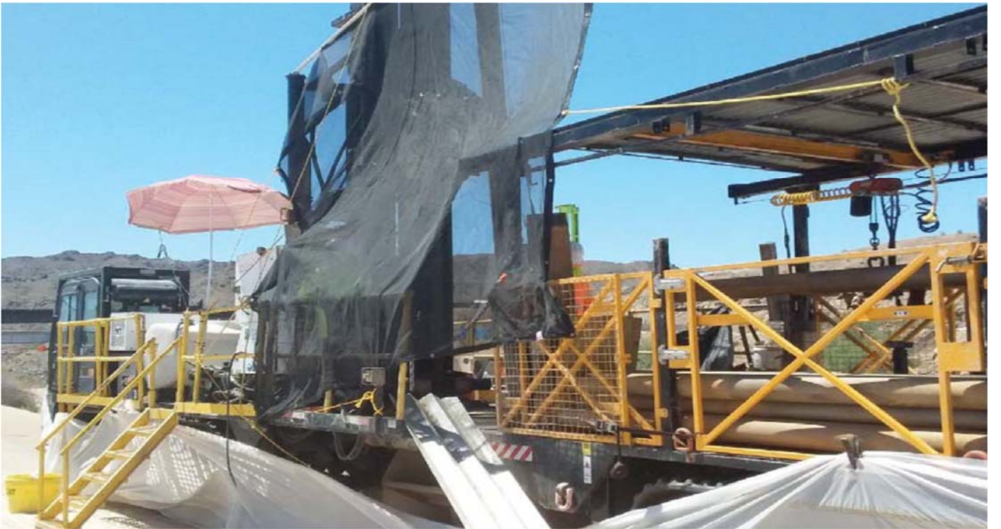
MW-H Well Installation
