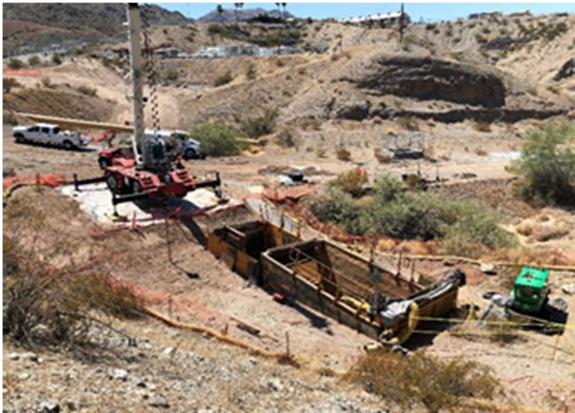
Photo showing jack and bore activities at the southern end of Pipeline C, Segment C9.
