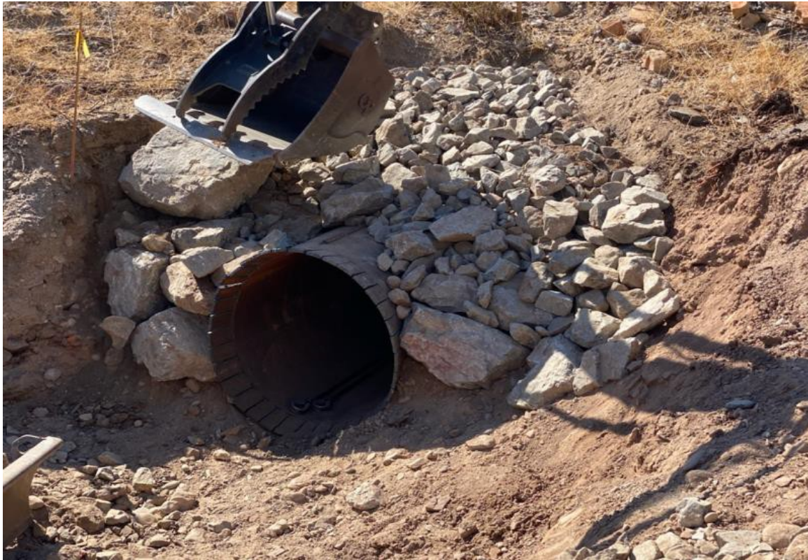
Photo showing rock placed at northern end of Pipeline C, Segment C9 for slope protection.
