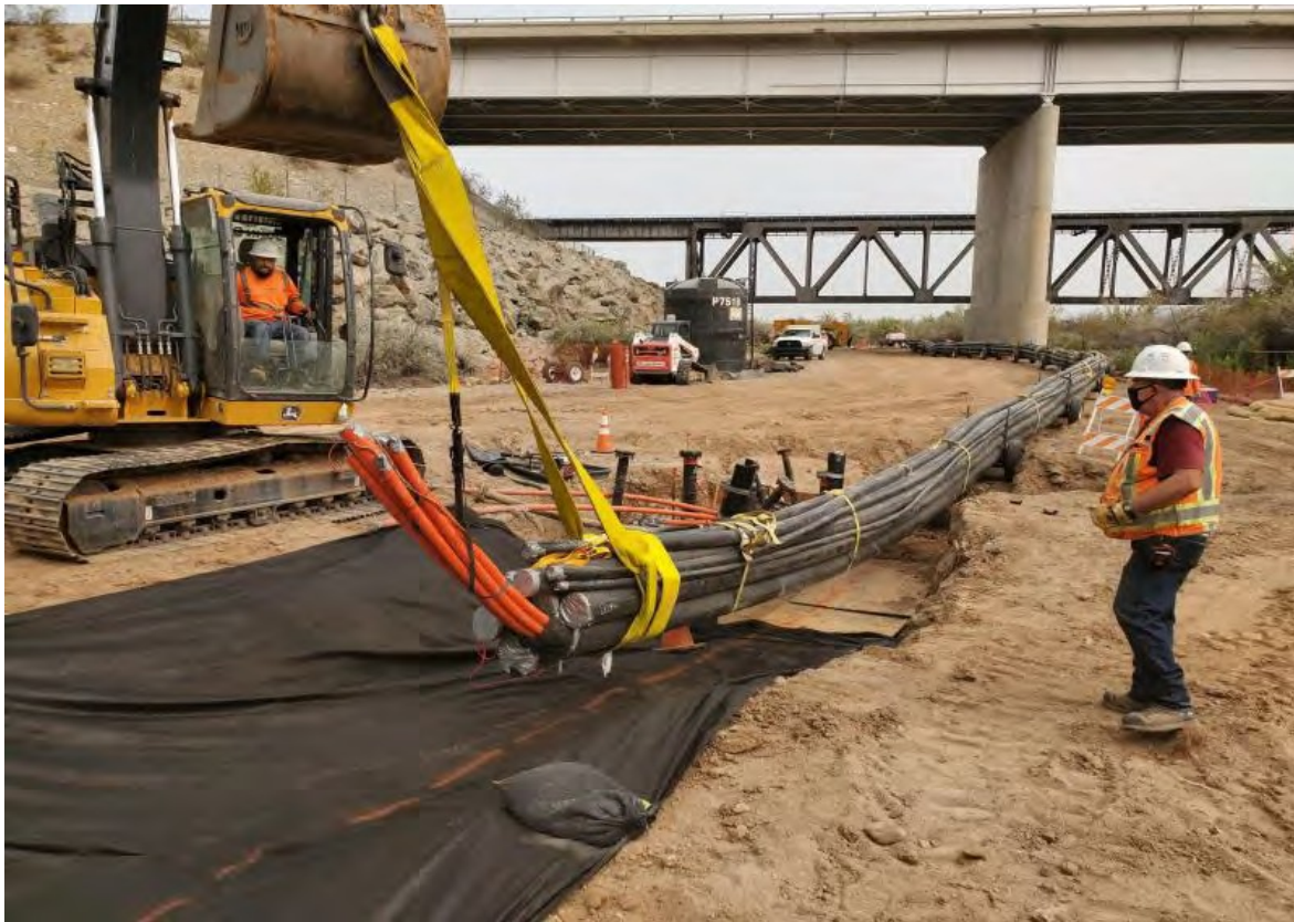
Photo showing pulling of bundled pipes up to the northern C9 carrier pipe.
