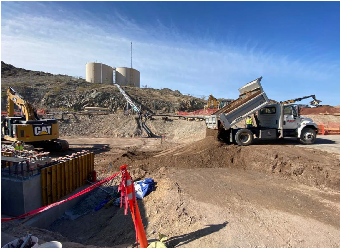
Photo showing earthwork to install the Remedy-produced Water Condition System tank pad inside the Compressor Station.
