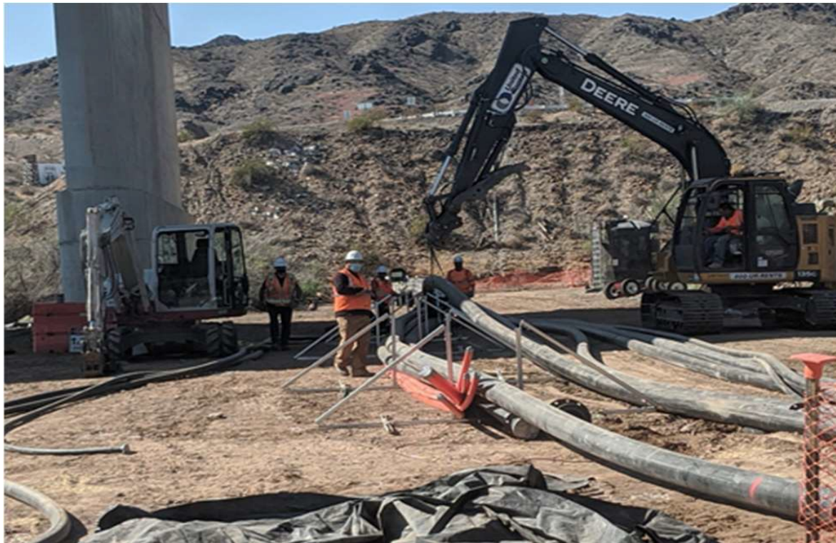
Photo showing pipe bundling at the northern end of Pipeline C, Segment C9.
