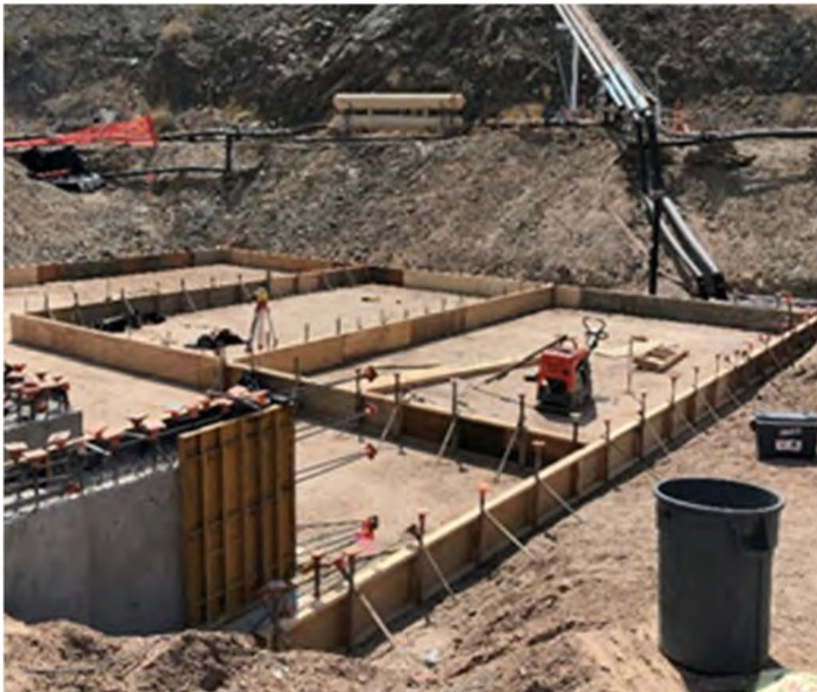
Photo showing earthwork to install the Remedy-produced Water Condition System tank pad inside the Compressor Station.
