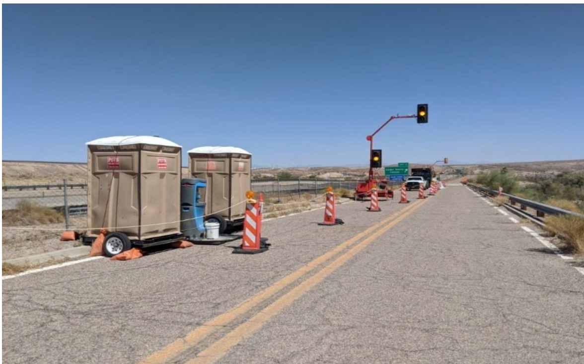
Photo showing set up of traffic control at the MW-99 well site, along the frontage road south of I-40
