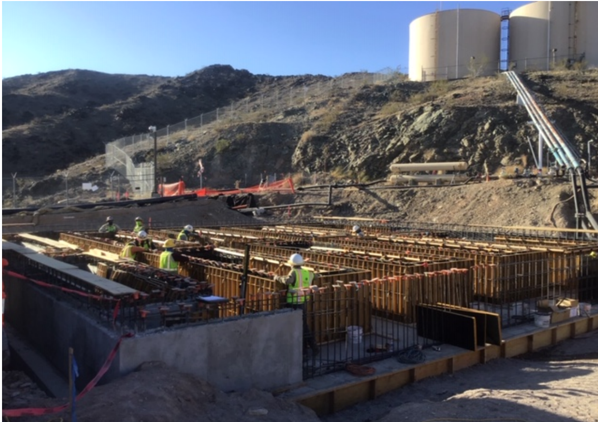
Photo showing forms removal after concrete pour at tank pad.
