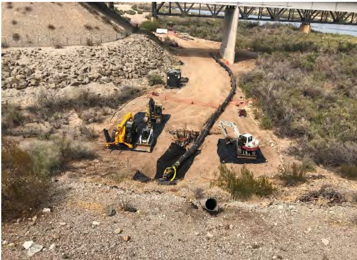
Photo showing pipe bundles aligned to the northern C9 carrier pipe.
