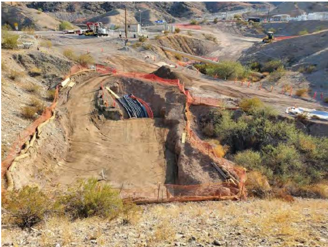
Soil Backfill at C9 South
