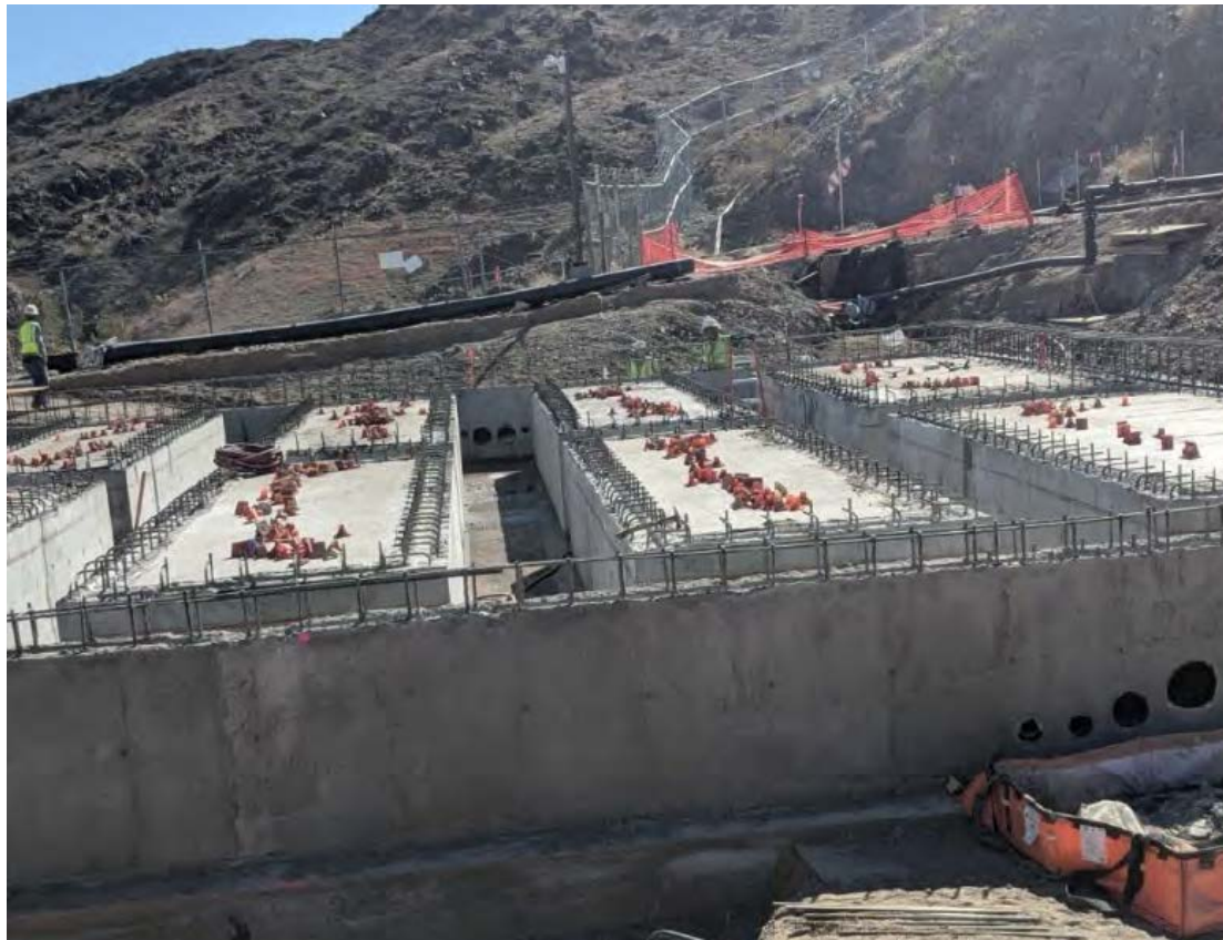
Concrete Pedestal for Wastewater Storage Tanks at the Remedy- Produced Water Tank Pad inside TCS
