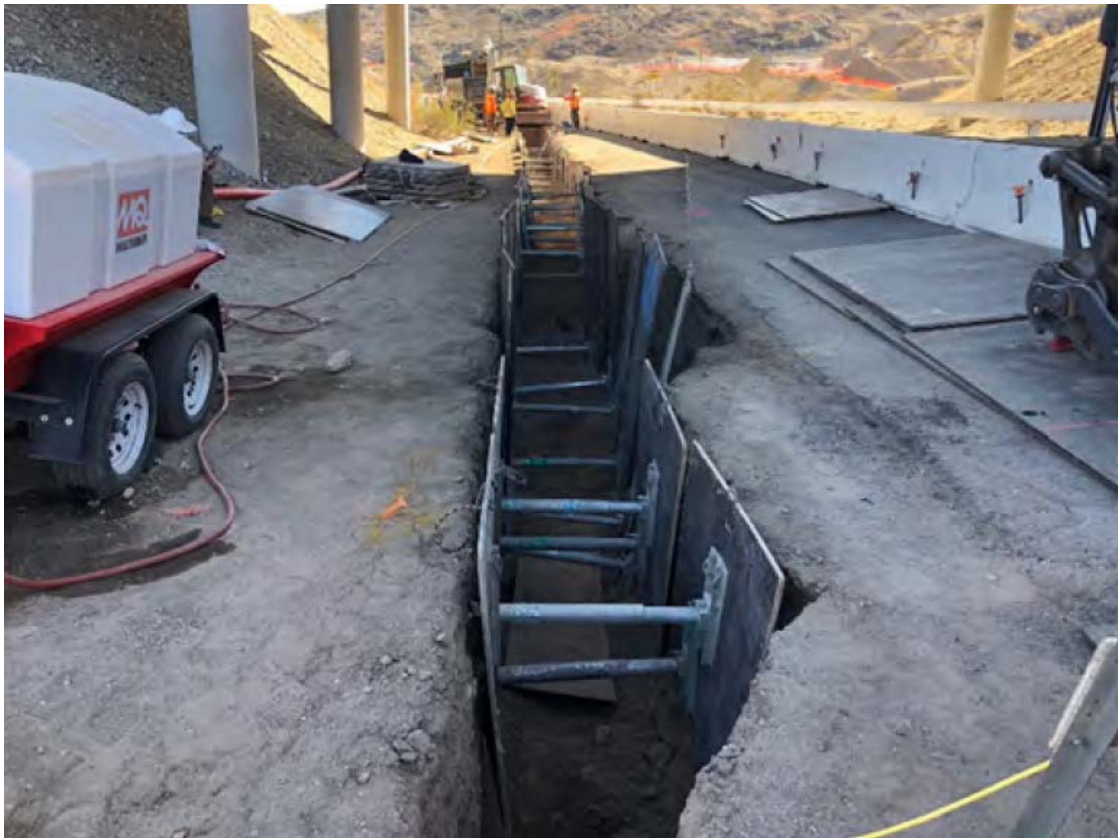
Two photos showing pipeline C16 trench with shoring plates and installation of a handhole along pipeline C15.
