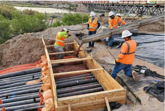
Photo showing placement of concrete at top of slope of Pipeline C6
