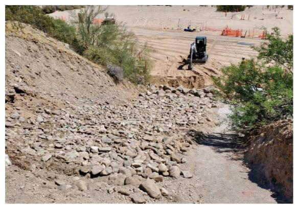
Photo showing backfill along slope of Pipeline C6
