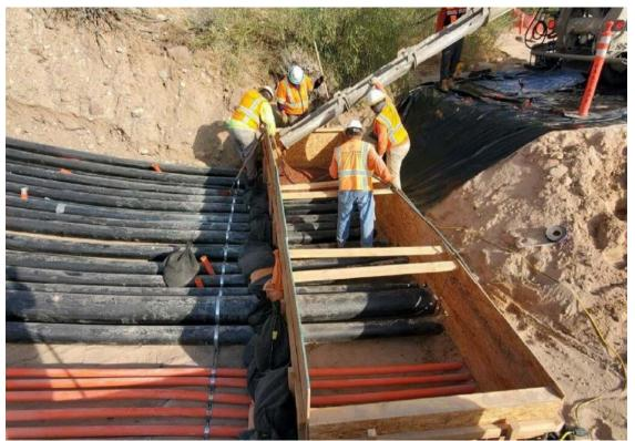
Photo showing placement of concrete at toe of slope of Pipeline C6
