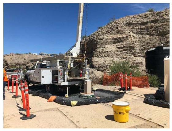
Photo showing well development rig setup at MW-95 (former MW-V)
