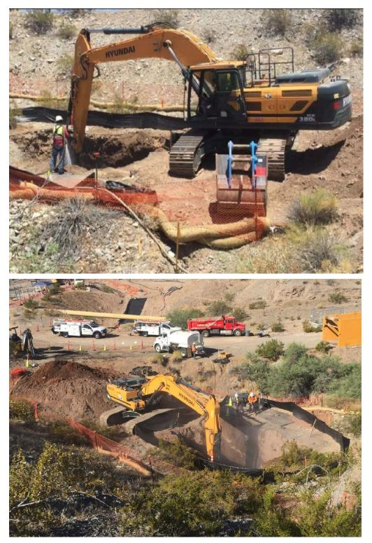
Two photos showing excavation of the southern jack and bore pit at Pipeline C9
