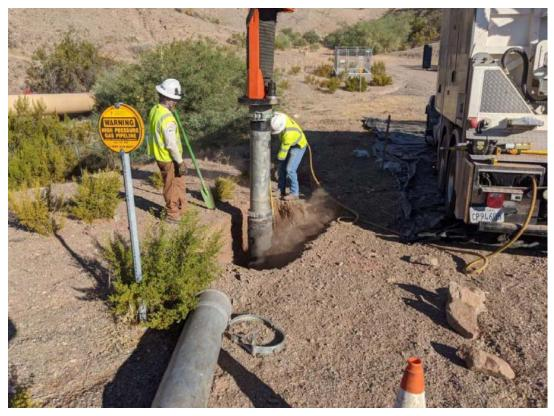
Photo showing air-vac operation to excavate for Kinder Morgan utility crossing at Pipeline F1
