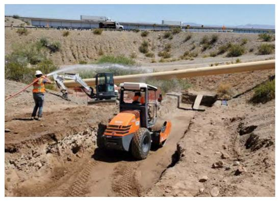
Photo showing compaction of subgrade at Pipeline F1
