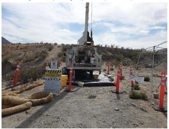
Photo showing well development rig set up at MW-93 (former MW-Z)
