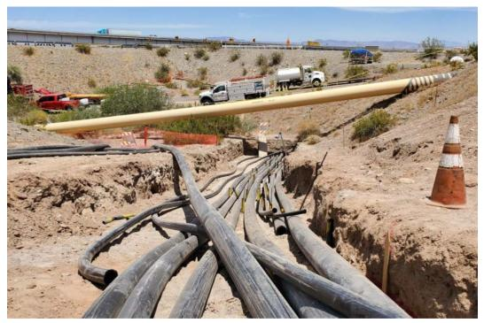
Photo showing HDPE piping at Pipeline F1
