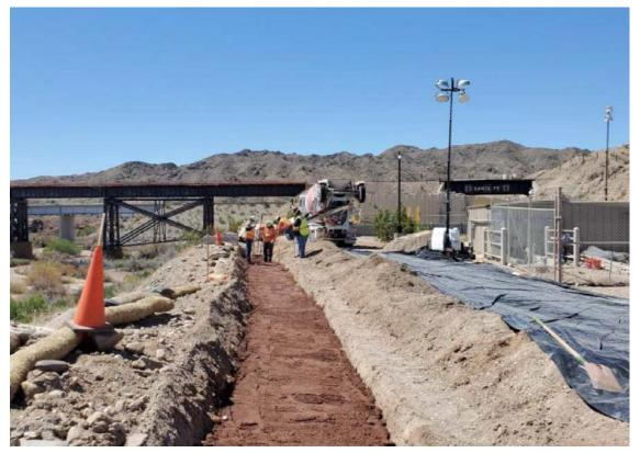
Photo showing placement of slurry mix with utility red dye along conduit duct bank of Pipeline C6
