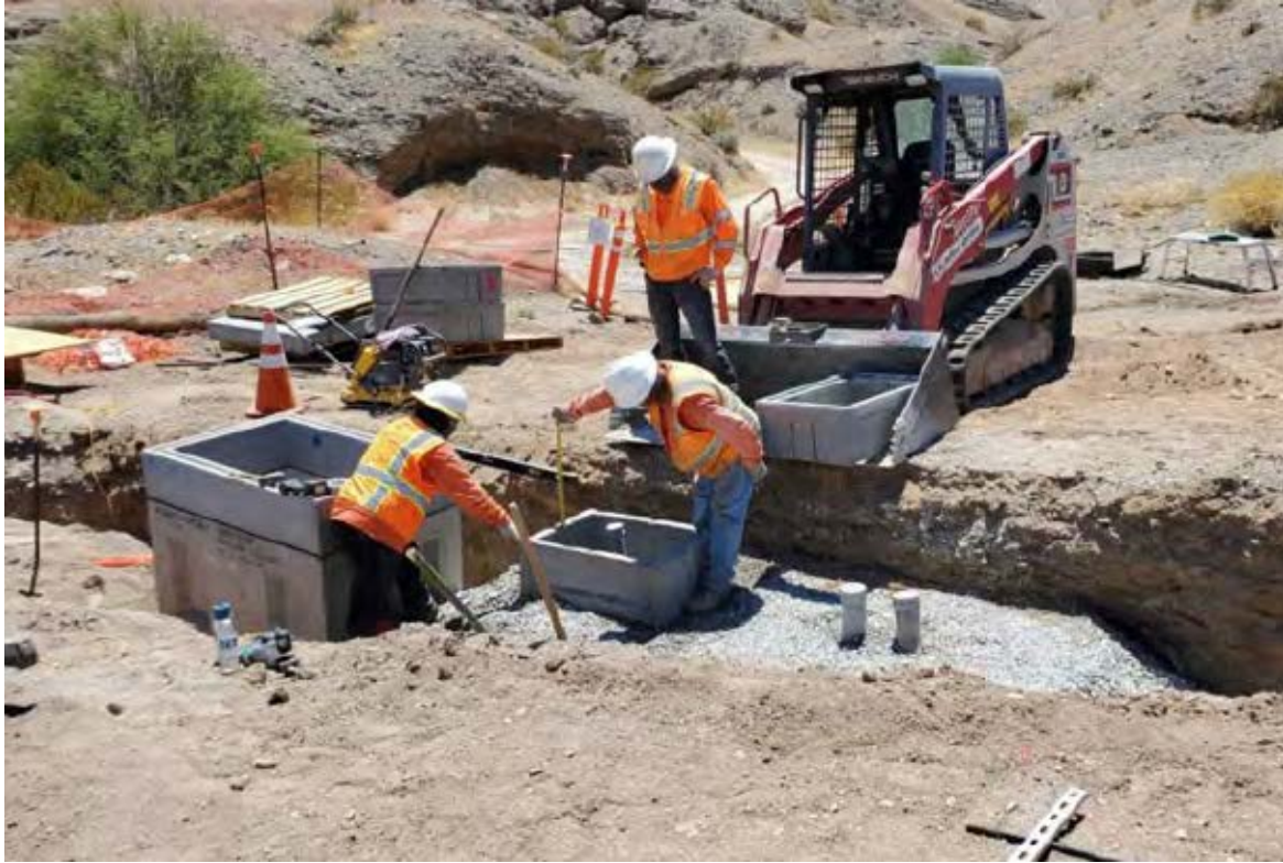
Photo showing pull box installation at Pipeline J Segment J3 South.
