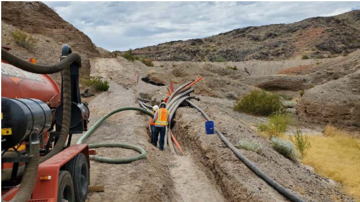
Photo showing repair of Pipeline J Segment J2 (removal of eroded fill material).
