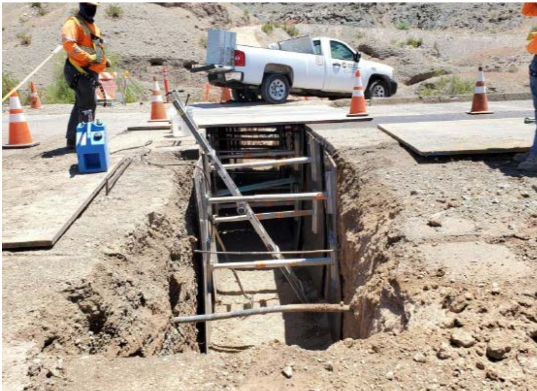
Photo showing excavation and shoring at Pipeline J Segment J4.
