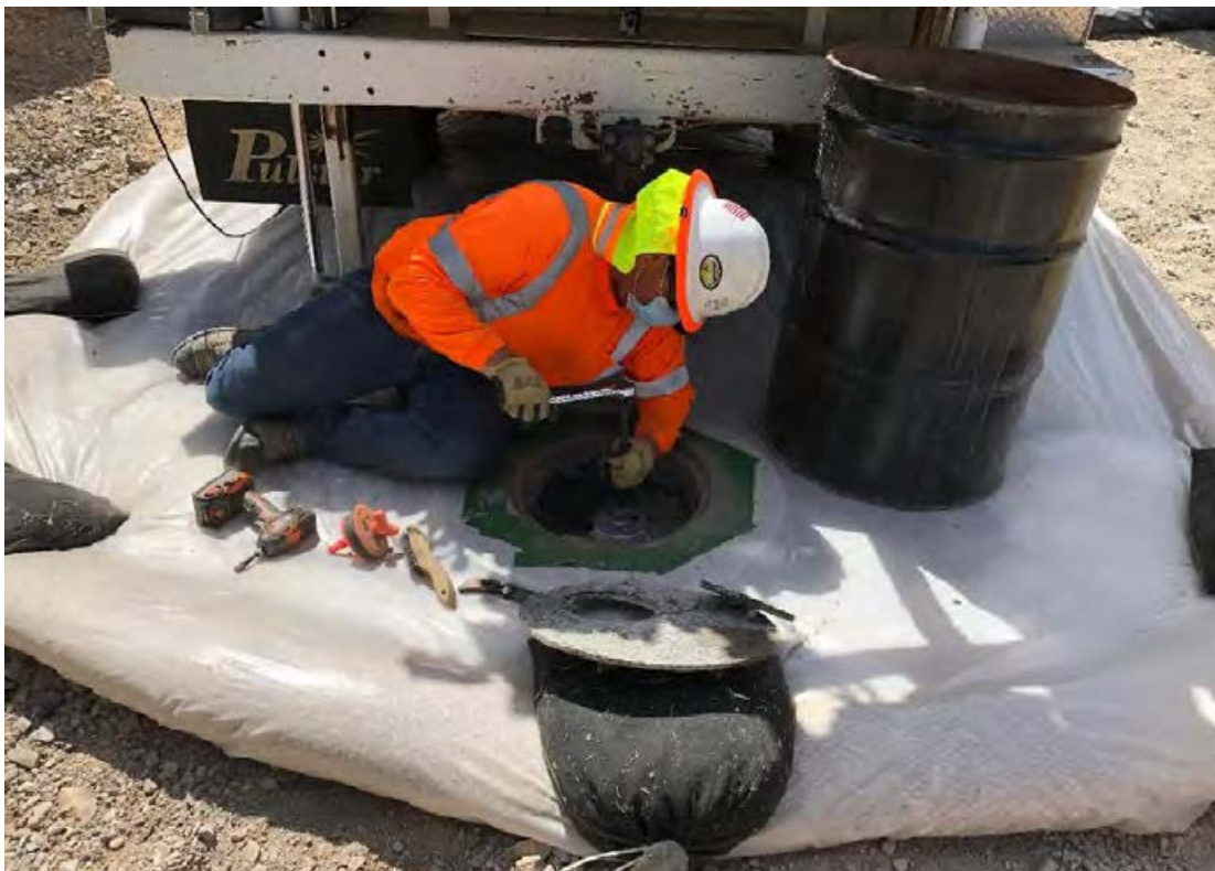
Photo showing driller cutting down PVC casing at MW-70BR.
