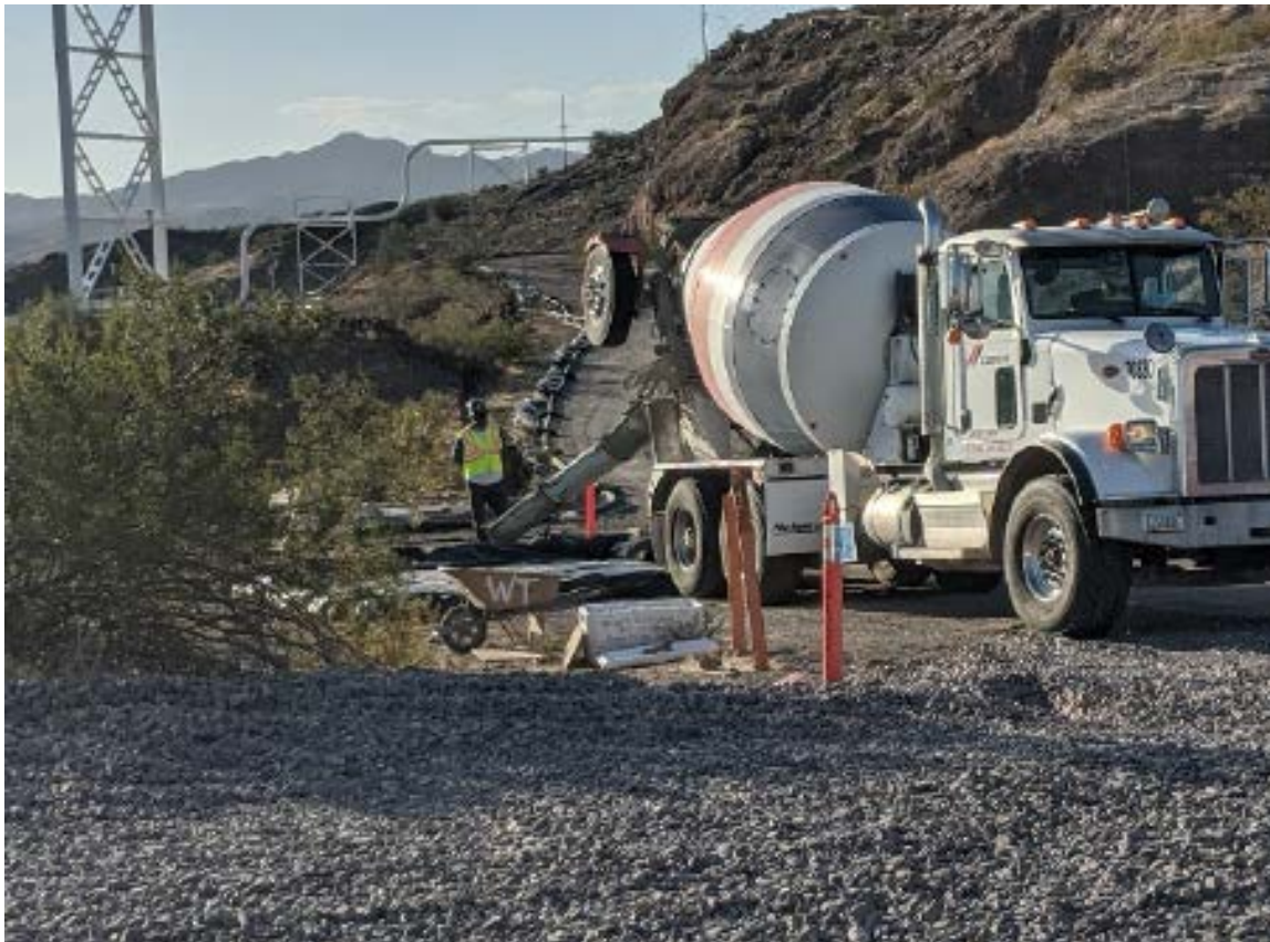
Photo showing concrete washout after a pour at Pipeline F/J.
