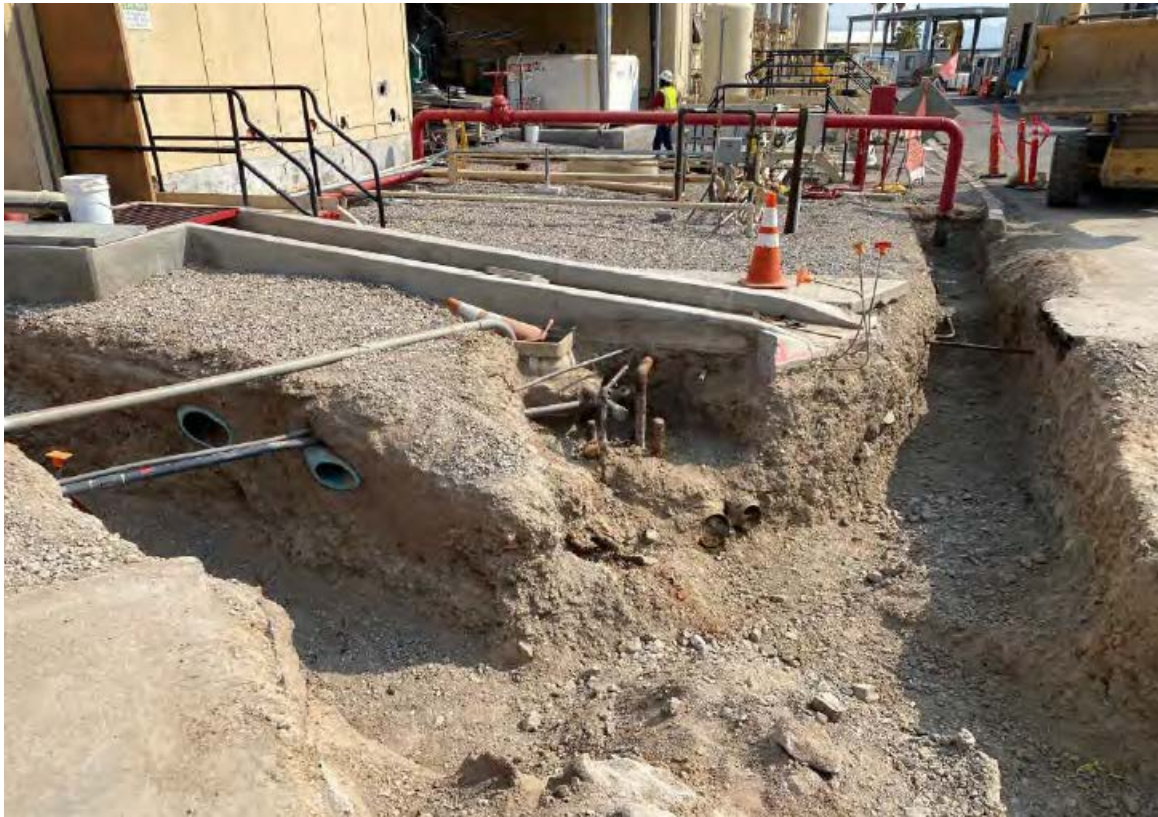
Photo showing trenches for firewater and raw water pipelines.
