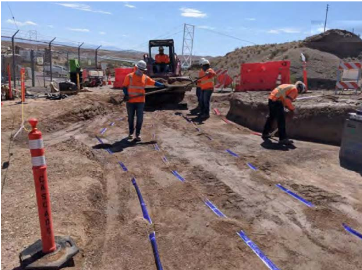
Photo showing installation of detectable marking tape at Pipeline J Segment J3.
