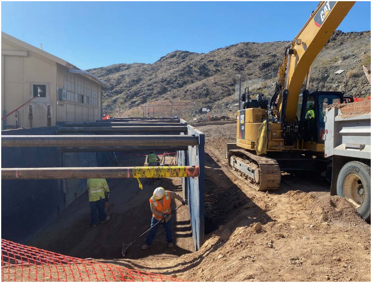
Photo showing compaction of AB material inside shore box.
