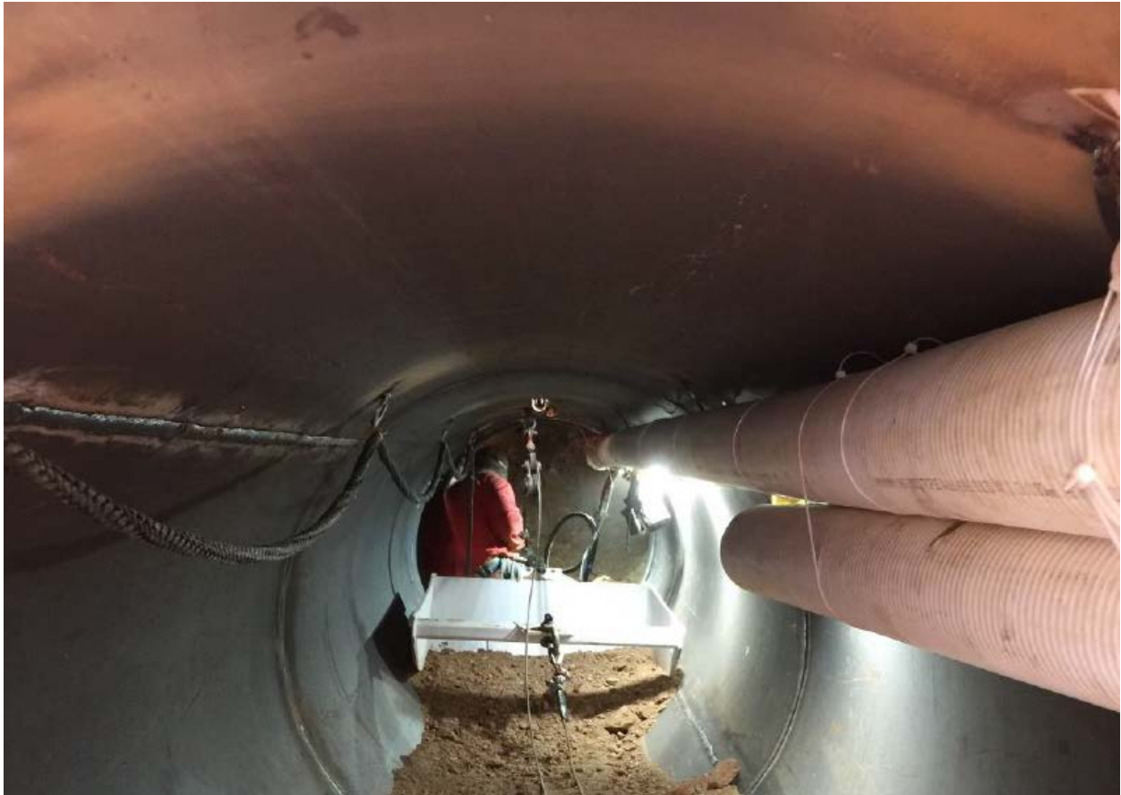
Photo showing hand mining operation at C9 jack and bore.
