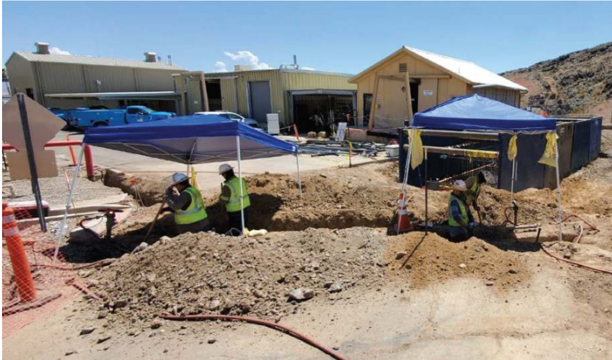
Photo showing hand dug of remedy pipe/conduit trenches inside TCS.
