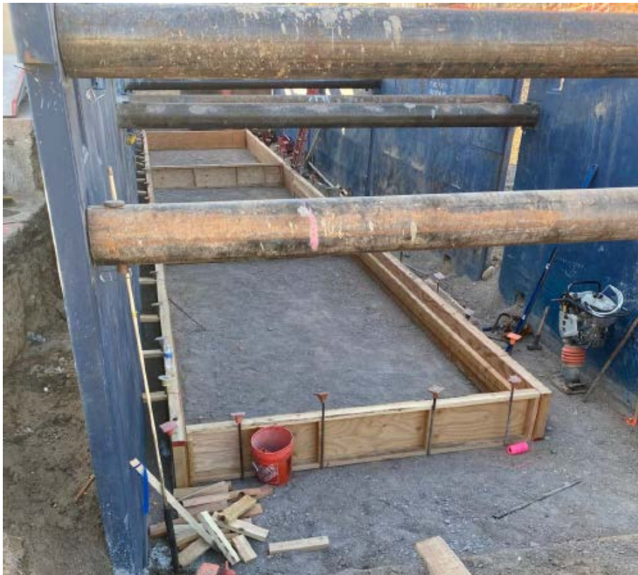
Photo showing compaction of AB material inside shore box.
