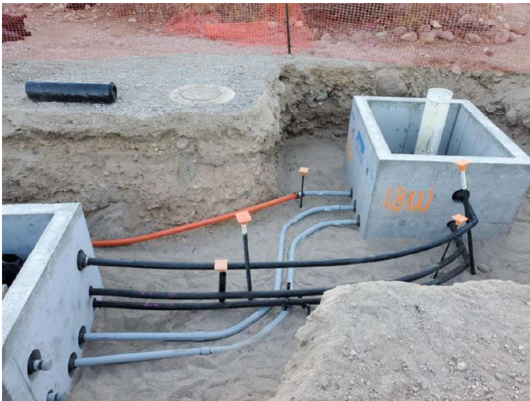
Photo showing pipe and conduit installation at IRZ-18.
