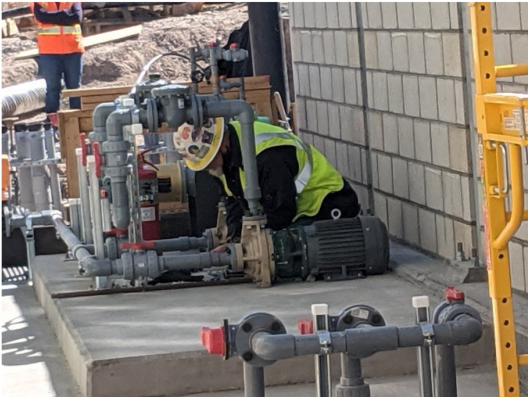
Photo showing bolting of components at the Remedy-produced Water Tank Pad at TCS.
