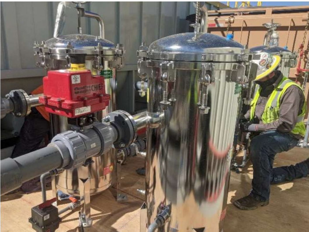
Photo showing cartridge filters at the Remedy-produced Water Tank Pad at TCS.
