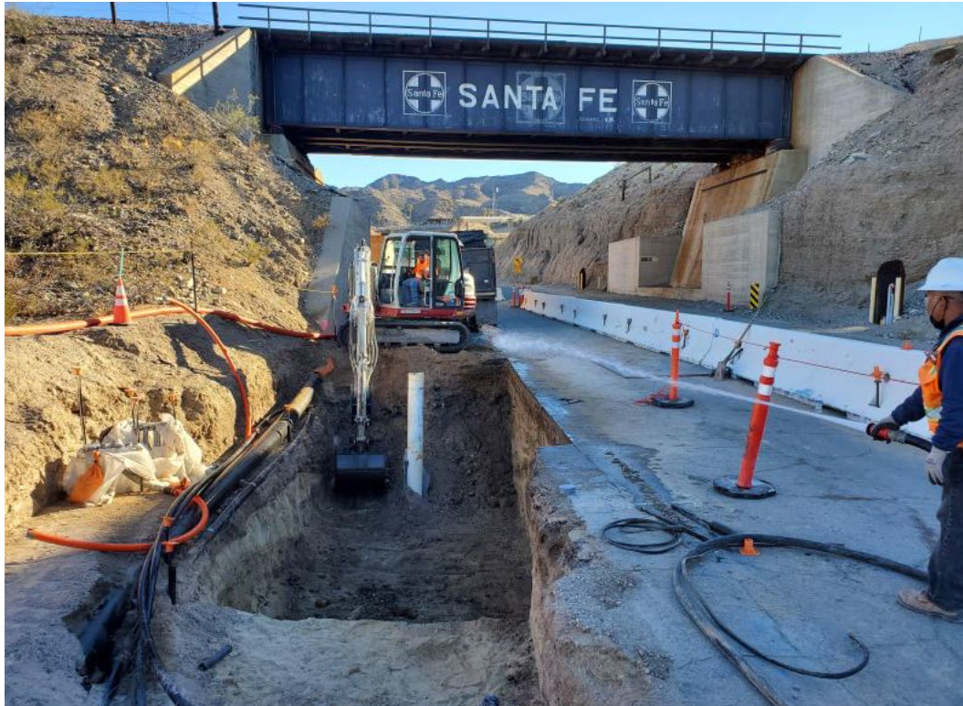
Photo showing excavation for installation of IRZ-27 vault and dust control.
