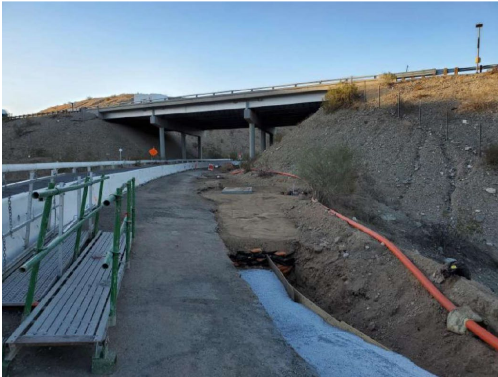
Two photos showing earth fill installation at Pipeline C Segments 19 and 20 along National Trails Highway.
