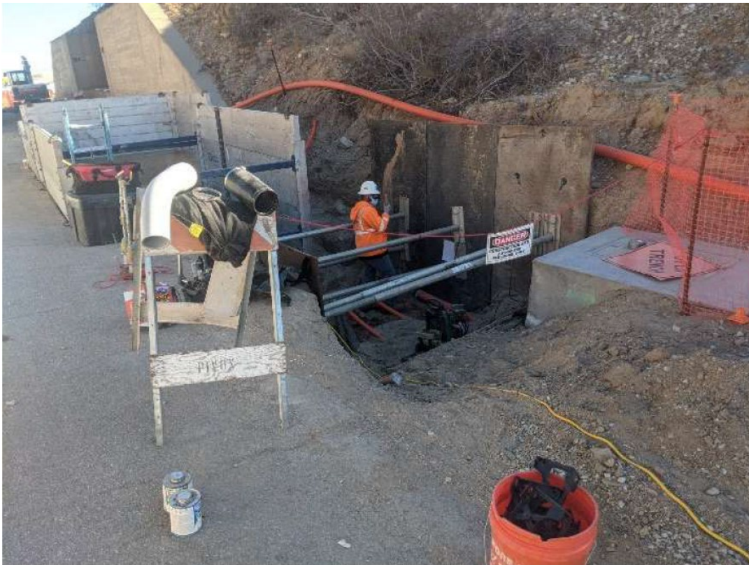
Photo showing conduit installation and form work for backfill along National Trails Highway.
