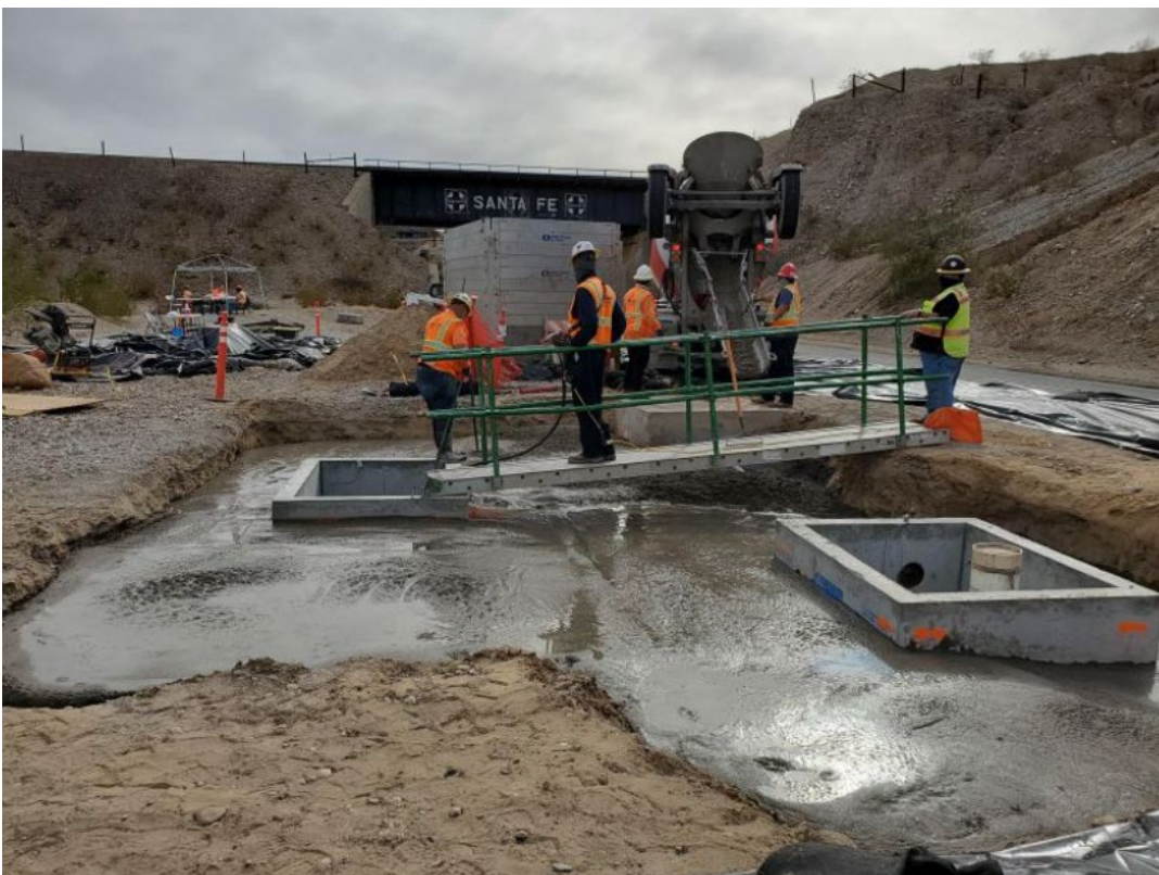
Photo showing slurry backfill at IRZ-25.
