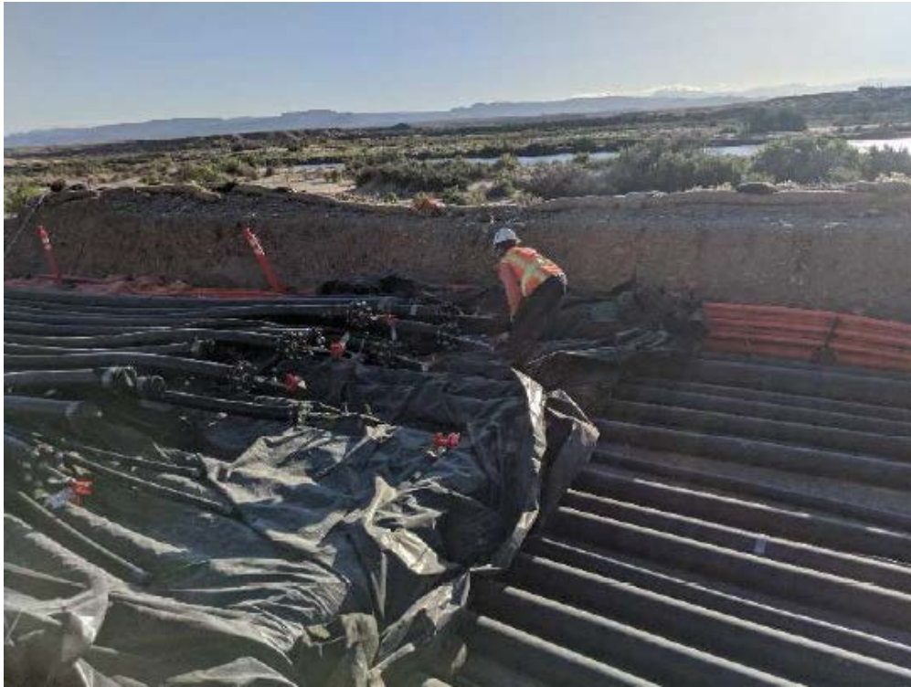
Photo showing hydrostatic testing at Pipeline C6 on the MW-20 Bench.
