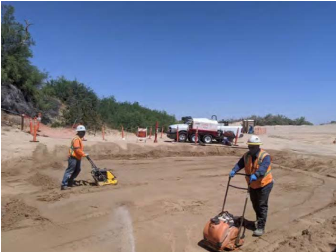
Photo showing backfill and compaction at Pipeline C6, Floodplain.
