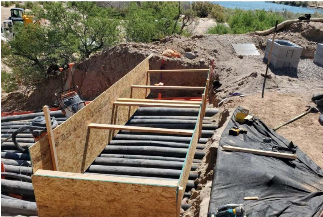
Photo showing form installation for concrete encasement at C6, top of slope
