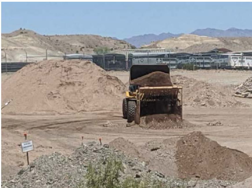
Photo showing material screening at the Soil Processing Yard.
