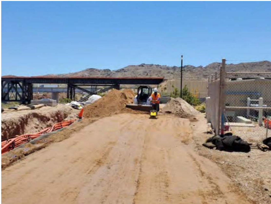
Photo showing backfill and compaction at Pipeline C6, MW-20 Bench.
