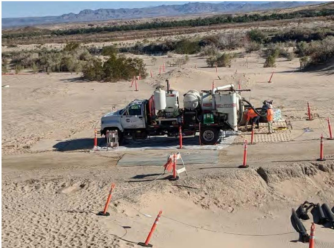
**Photo showing surface completion at MW-D**
