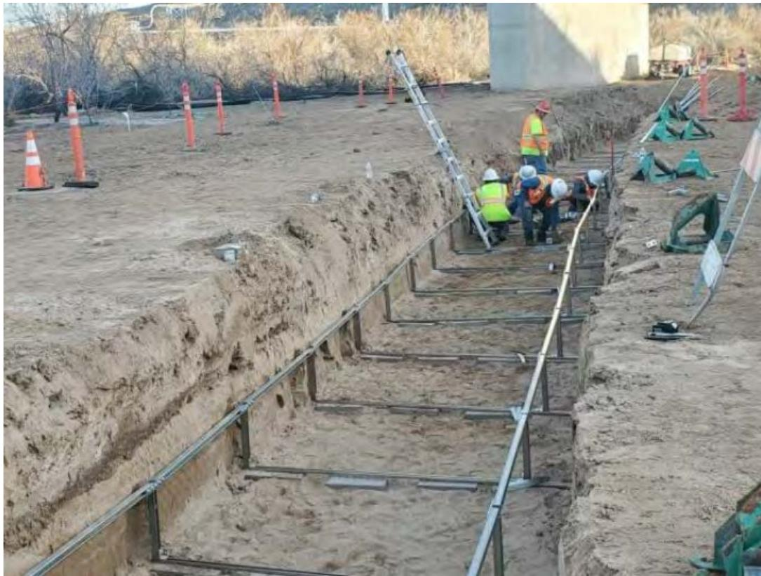
**Photo showing pipe support installation at Pipeline C8-Alt**
