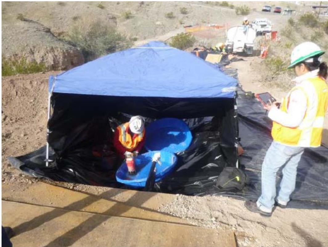
**Photo showing pumping of pipe flushing water at Pipeline B/J into water truck (background)**
