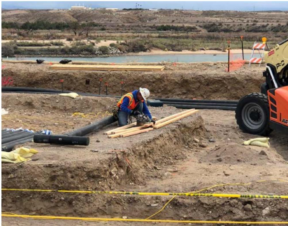
**Photo showing a worker setting form at MW-20 Bench**
