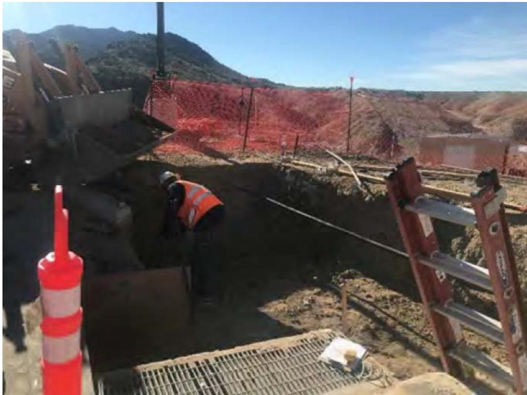
**Photo showing hand excavation at 90-degree corner at Pipeline M3 Station 61+90**
