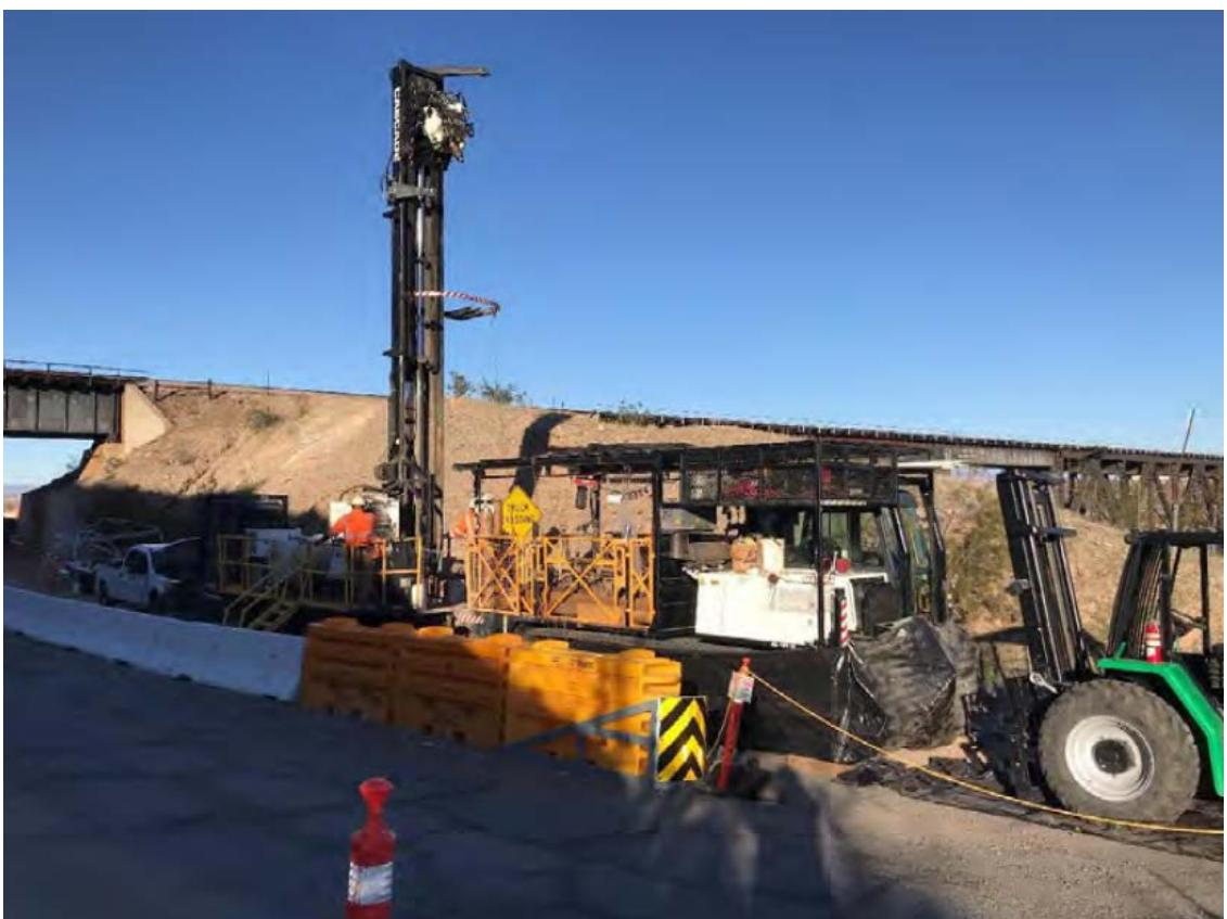
Photos showing drilling of IRZ-33 and IRZ-31 pilot boreholes along NTH
