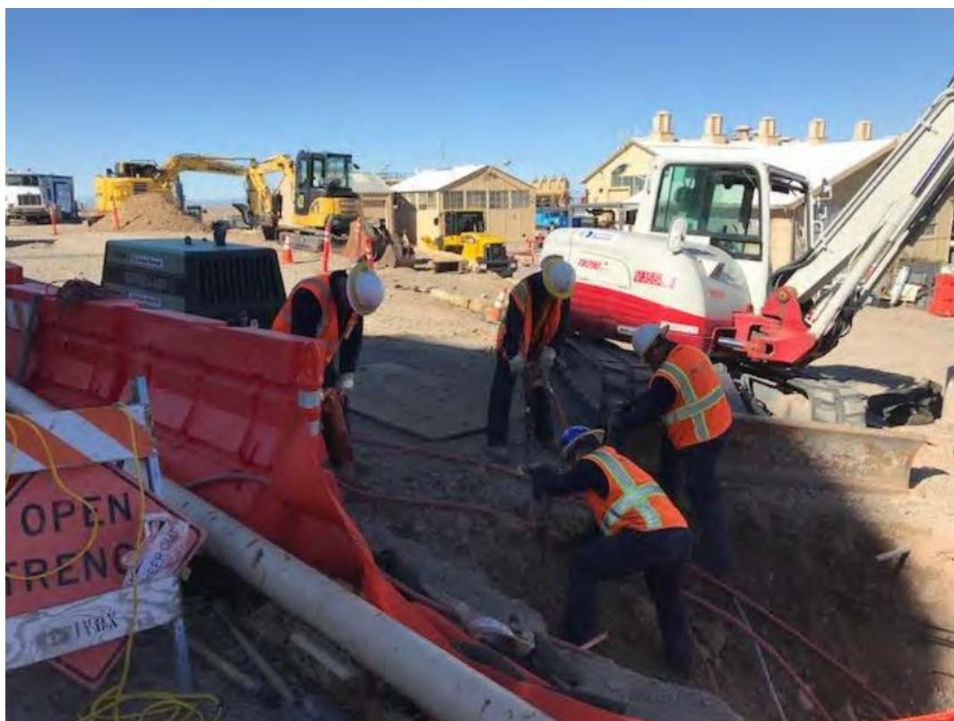
**Photo showing hand excavation at Pipeline B inside TCS**
