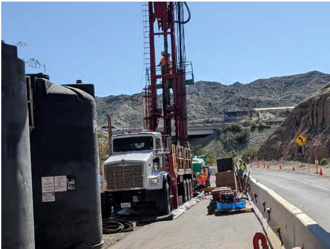
Photo showing well installation at IRZ-29.
