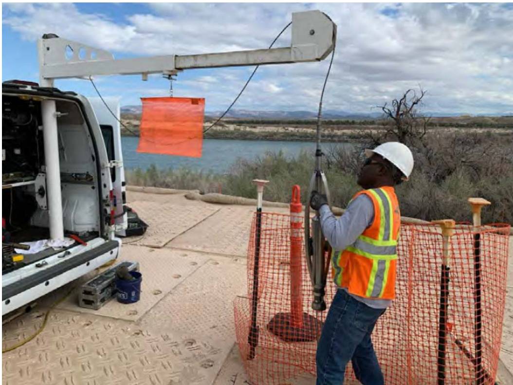
Photo showing installation of downhole camera at RB-2.
