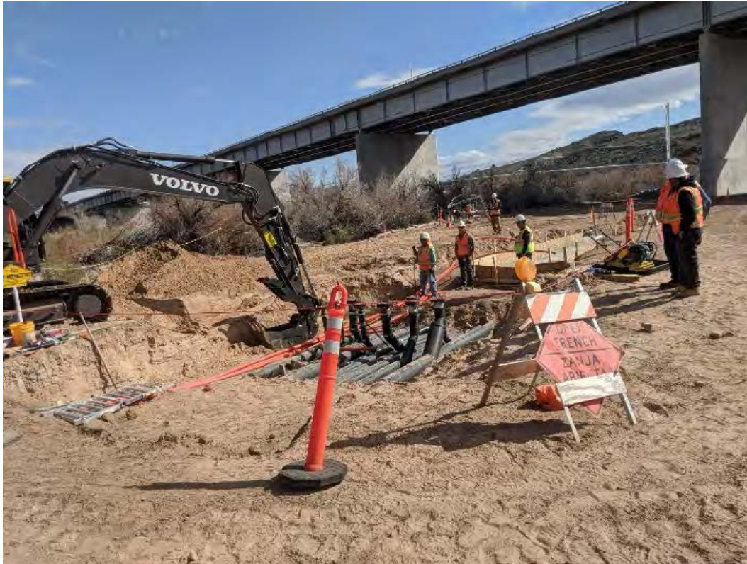
Photo showing backfilling at Pipeline C.
