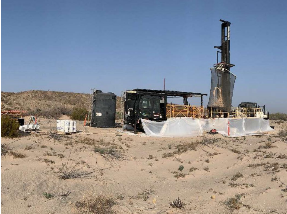
Photo showing installation of MW-96 with a rotosonic rig.
