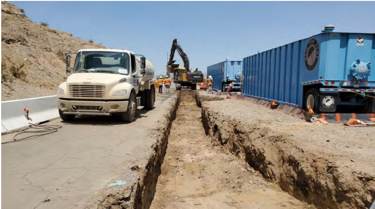
Photo showing excavation of Pipeline C Segment C13.
