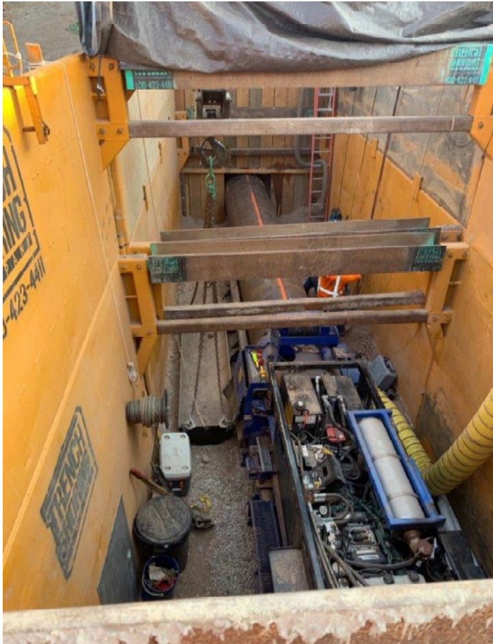
Photo showing Cal Boring auger operation.
