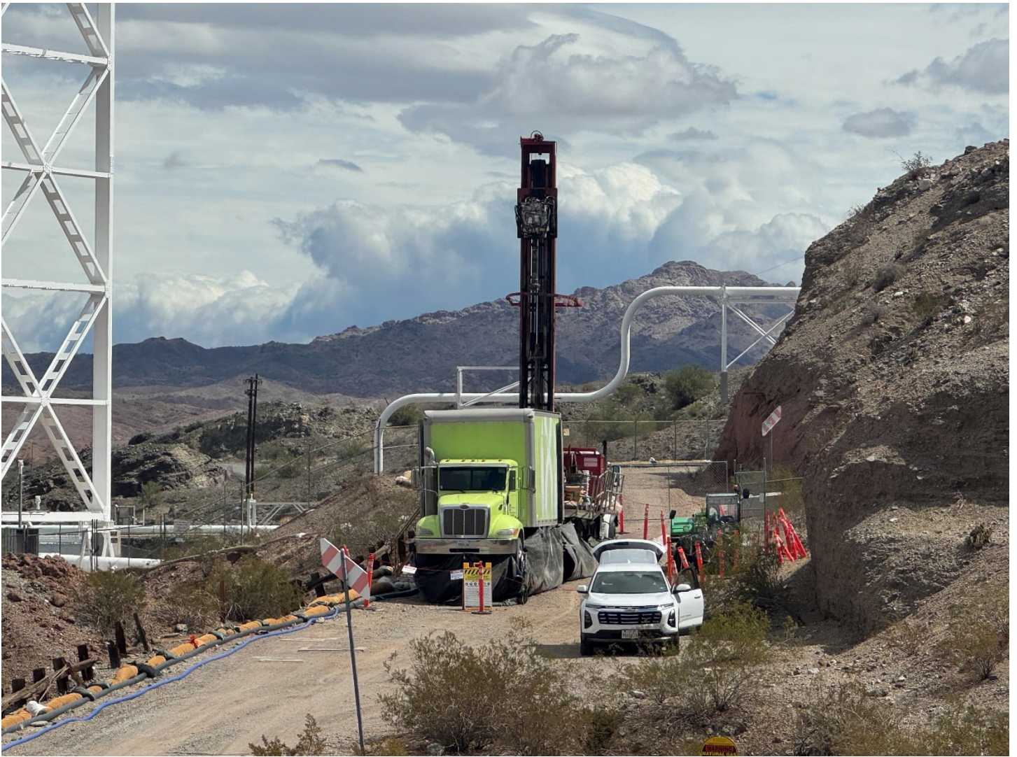
Photos showing the drill rig at MW-111 (former MW-T). Photo taken on 09/30/26.
