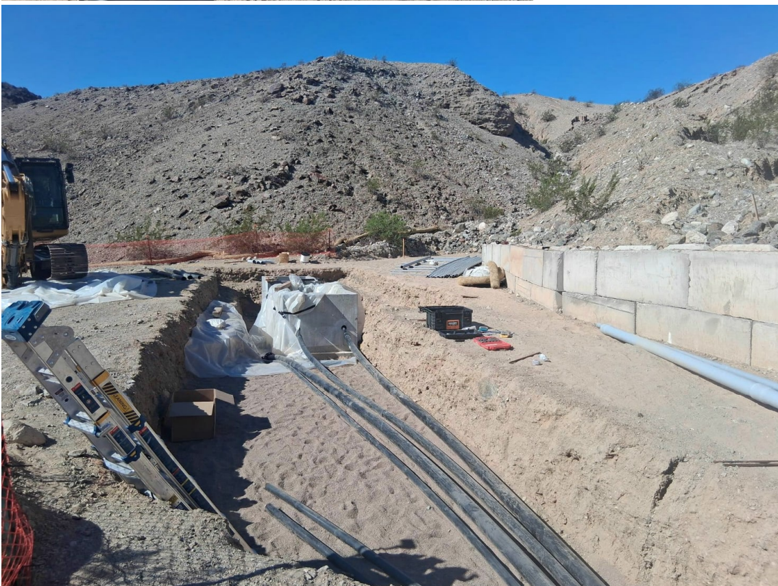
Photos showing in-progress Pipeline I2 and well vault at FW-02B looking towards Bat Cave Wash. Photos taken on 09/26/26.
