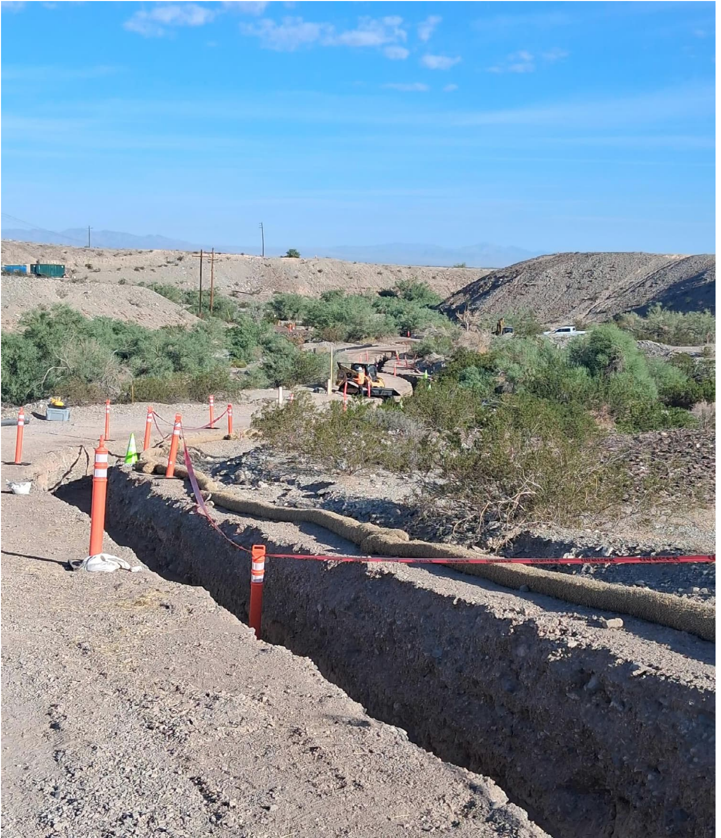
Photo showing in-progress Pipeline A, looking towards IM3 and Bat Cave Wash. Photo taken on 09/26/26.
