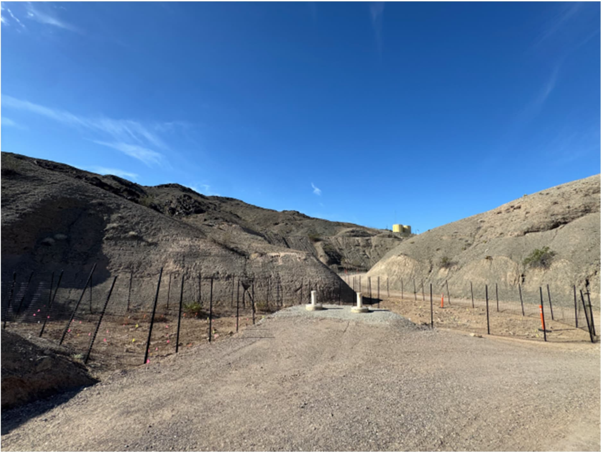
Photos showing in-progress Soil NTCRA mitigation planting areas in East Ravine. Photos taken on 09/26/26.
