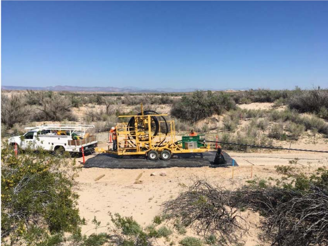
Relaxing pipe along the Pipeline C3 work area
