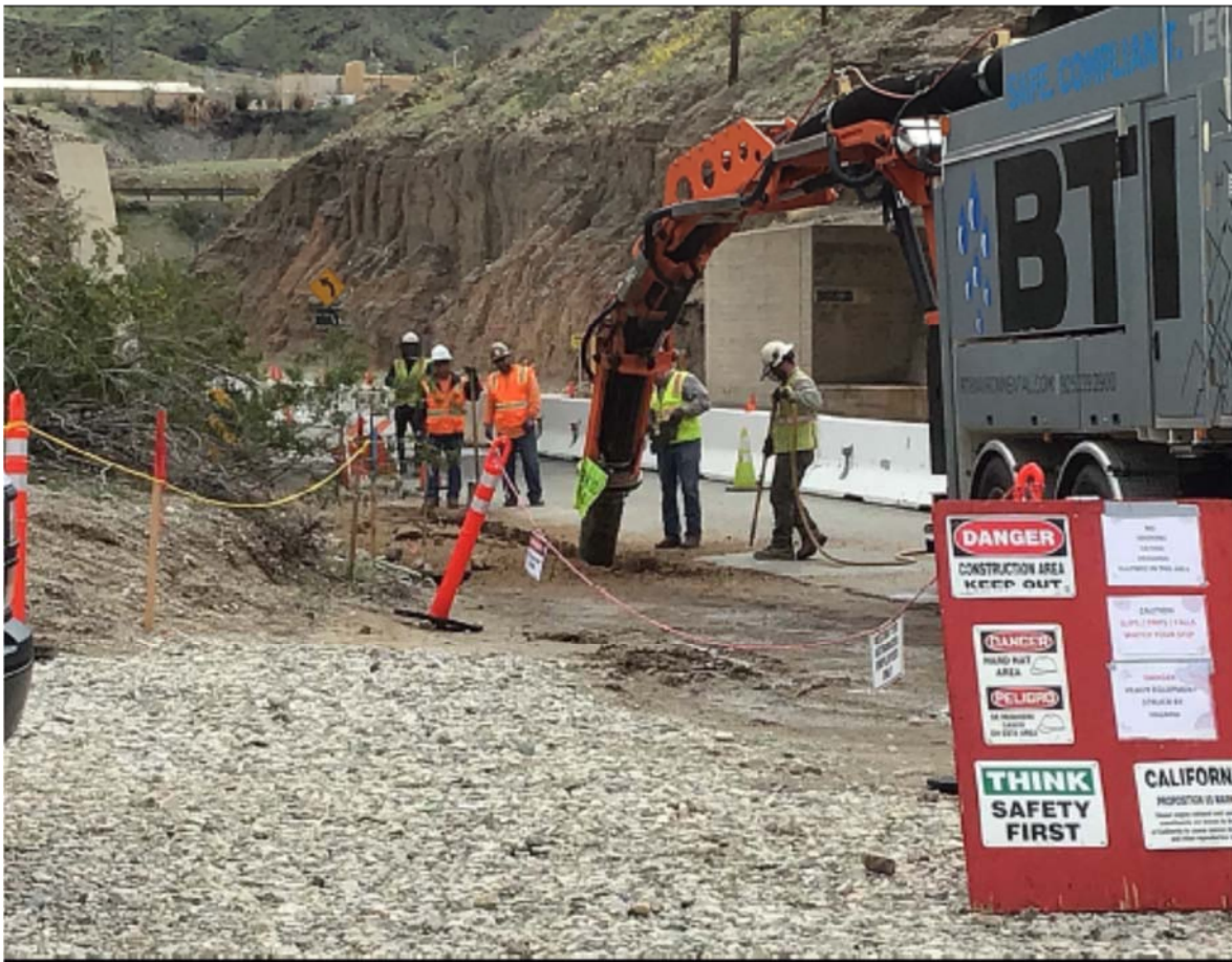
Air Vacuum Excavation to Daylight Utilities Along National Trails Highway
