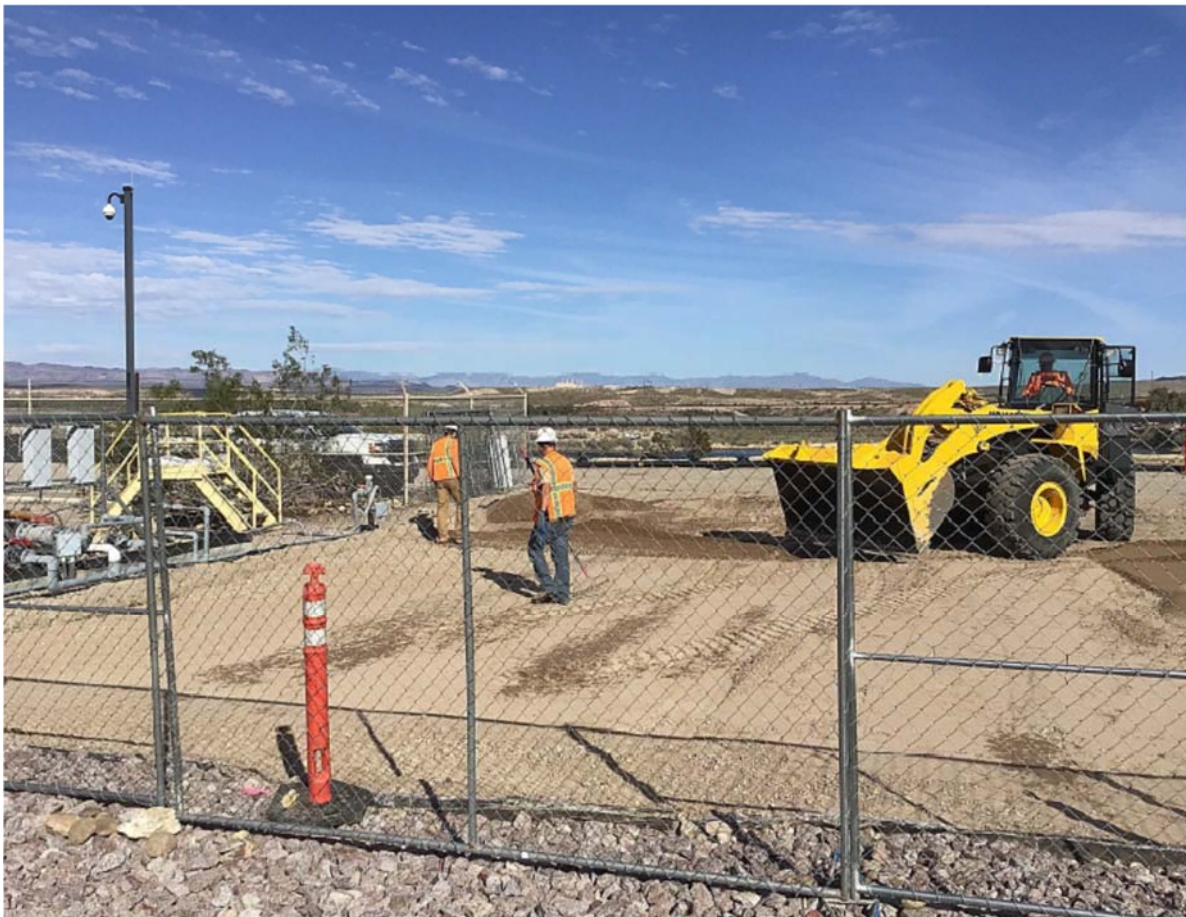
Compaction for brine tank containment upgrade
