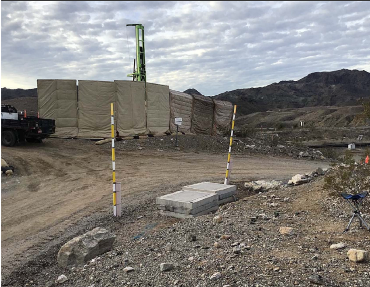
Sound curtain at MW-N well drilling location
