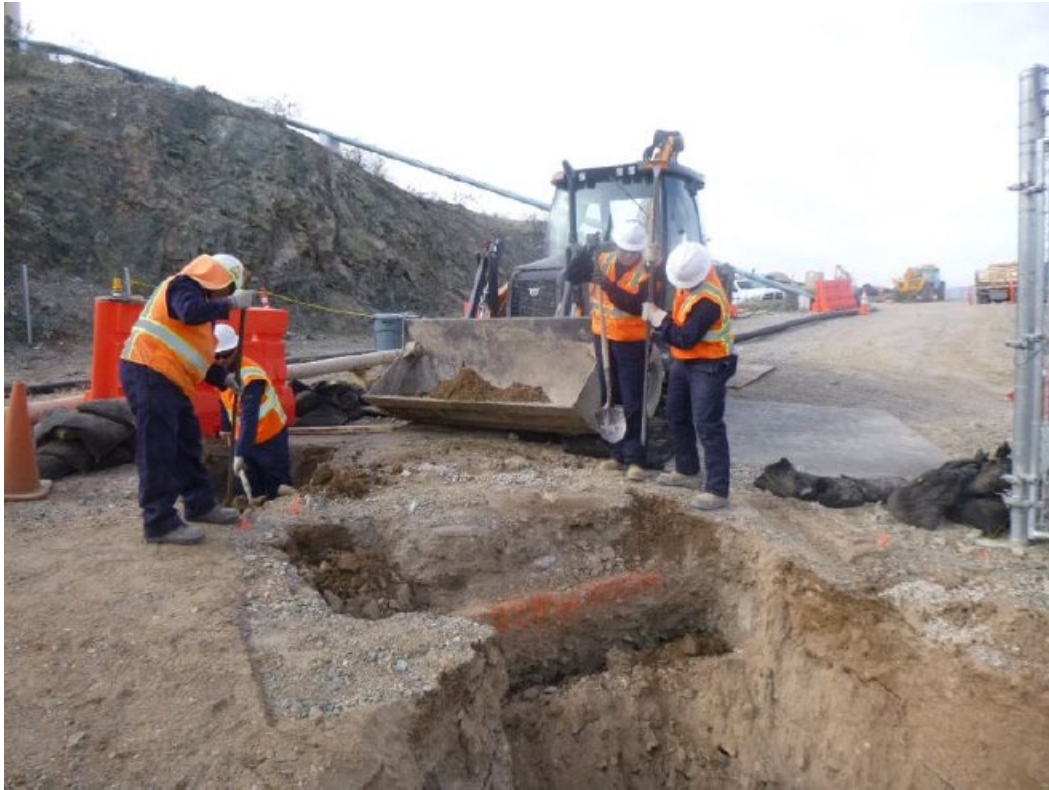
Photo showing hand excavation to locate utilities at Pipeline B, just inside TCS fence/gate
