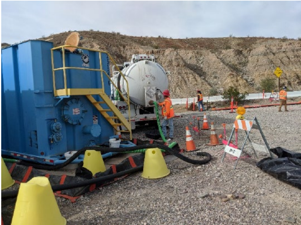
Photo showing transfer of wastewater from frac tank to vac truck for transport to pond for disposal
