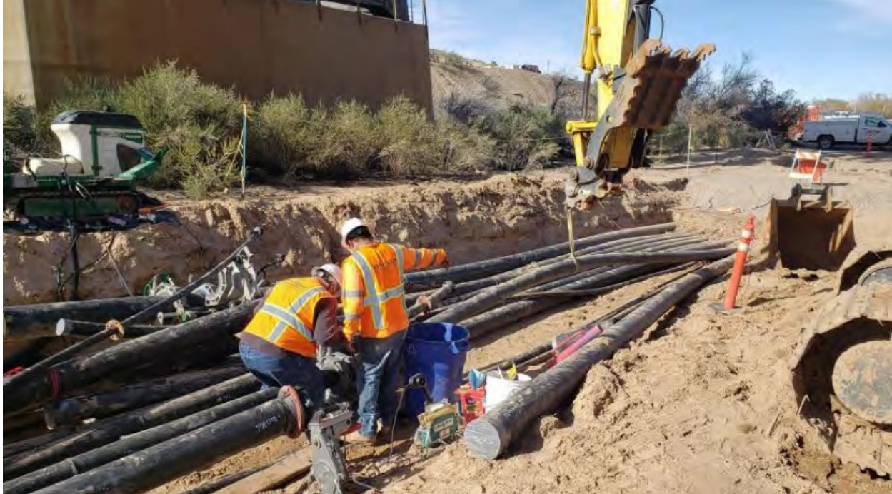
Photo showing fusing of pipes at Pipeline C7 in the floodplain
