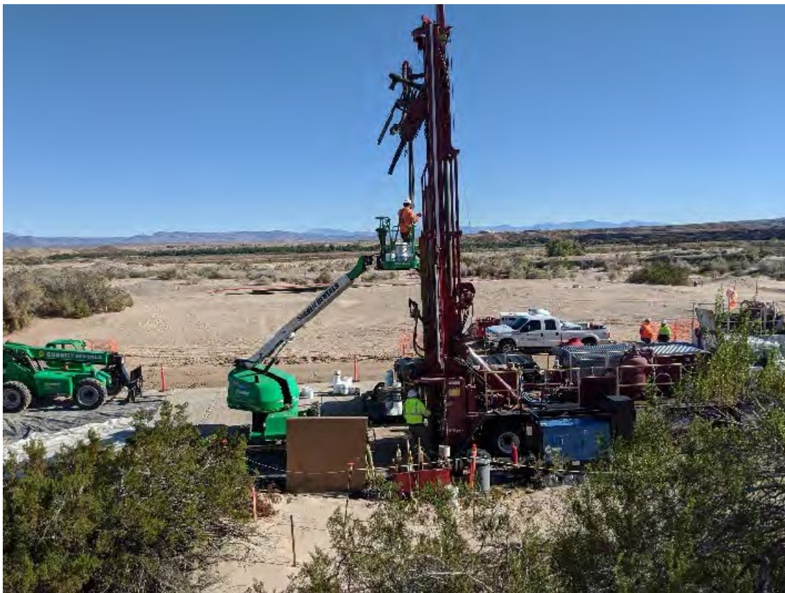
Photo showing backfilling of well at IRZ-16 in the floodplain
