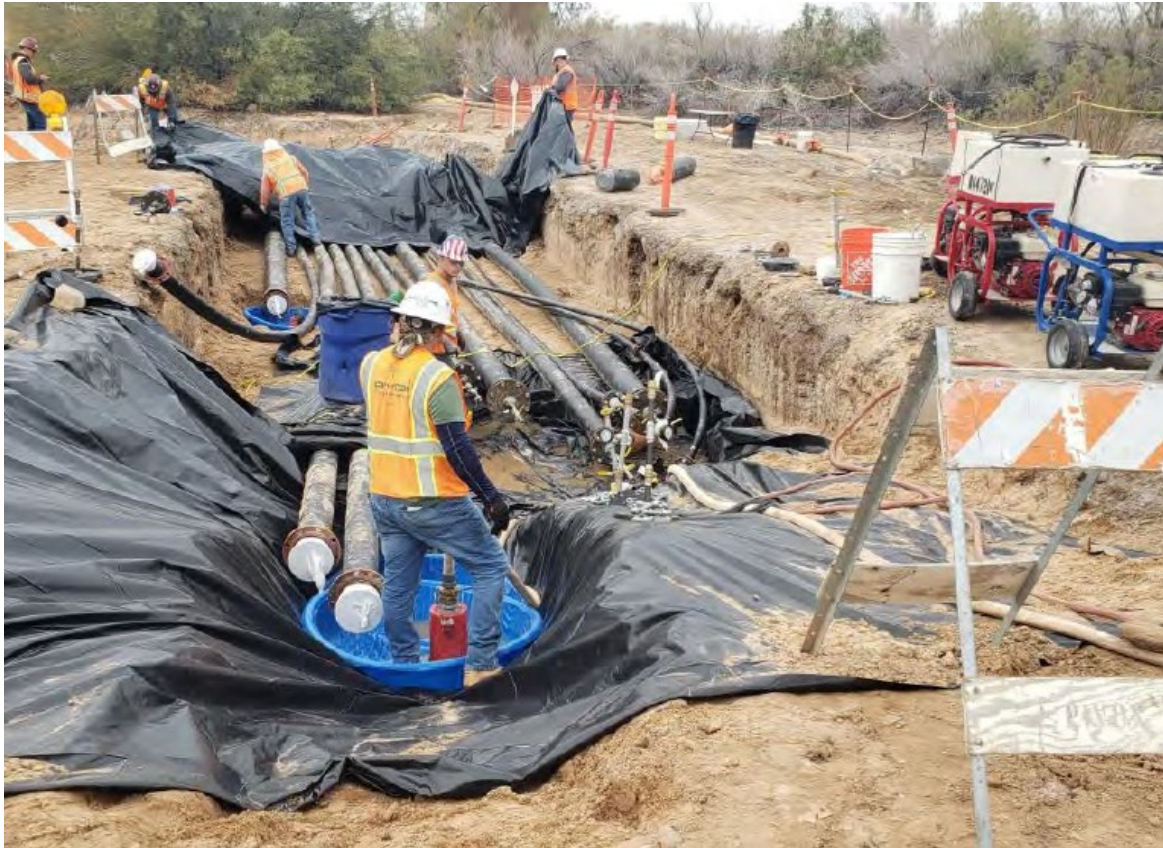
Photo showing pipe flushing setup/activities at Pipeline C8
