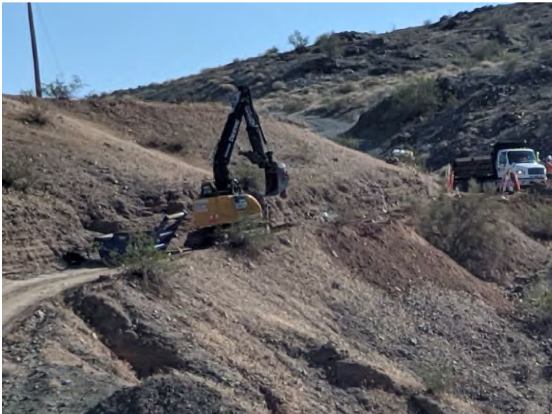
Photo showing trenching along the narrow alignment of Pipeline J
