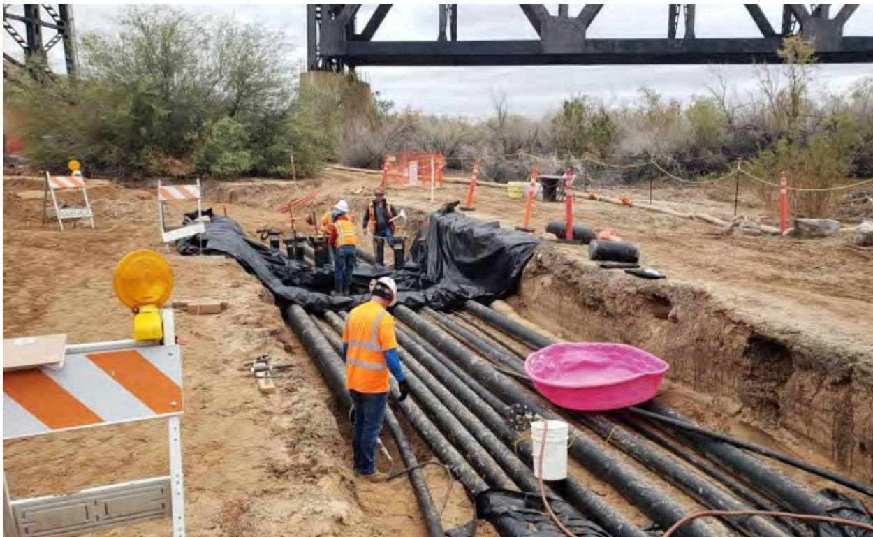
Photo showing leak test setup at Pipeline C8 end of the Pipeline C7, C8, C14 testing segment
