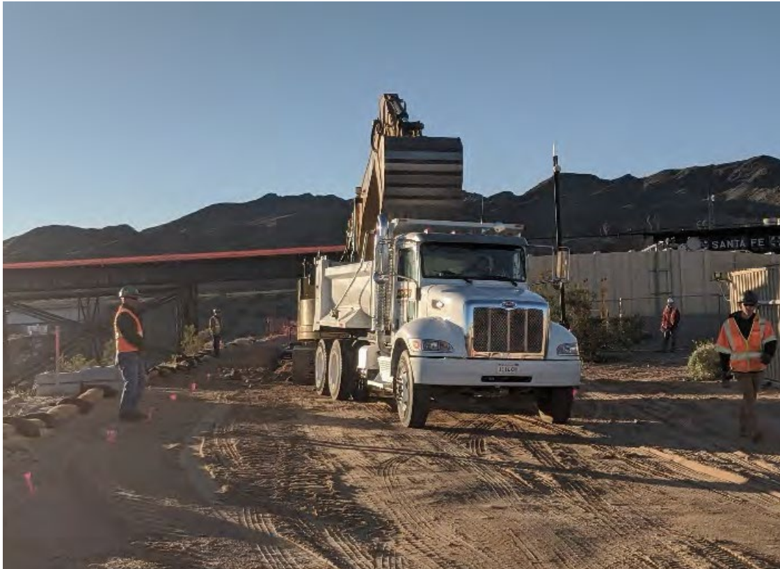
Photo showing loading of excavated material from MW-20 bench into dump truck for transport to SPY
