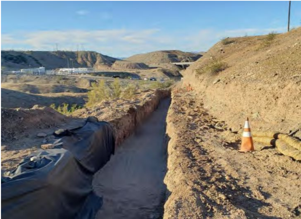
Photo showing Pipeline J trench prior to pipe placement
