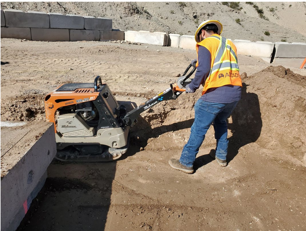
Photos showing backfill and compaction around TWB- 1 well vault
